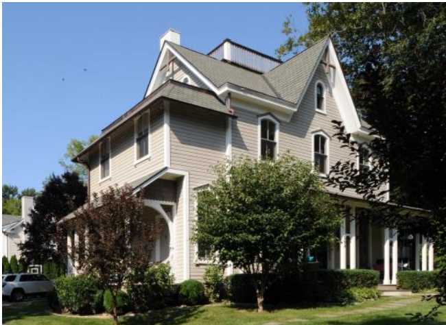
Additions to historic structures should not compete with the primary façade of the house. This addition at the side of the house would have been more appropriate if it had been set back off the face of the primary façade.
