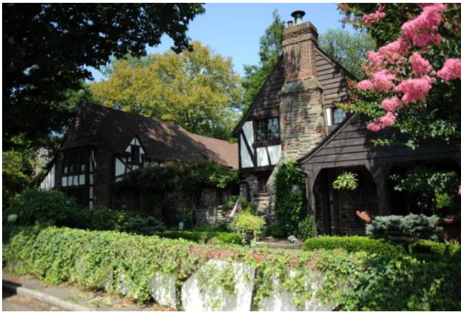
English Village Historic District is comprised of Tudor Revival twin and single family detached dwellings (with only two exceptions).
