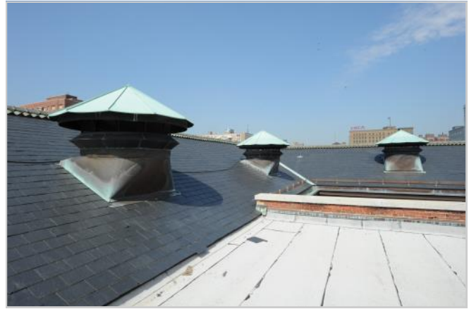
Ornamental sheet copper gravity ventilators were commonly employed on institutional buildings prior to mechanical air conditioning. Often still functional for attic ventilation, they should be preserved.
