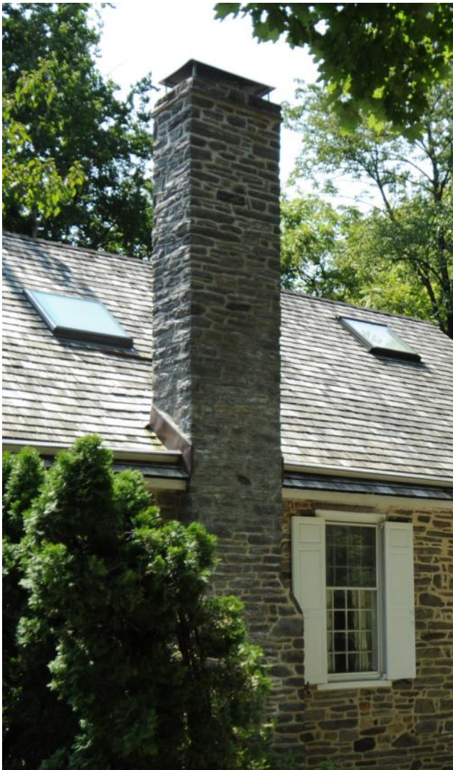
Chimneys on the oldest buildings in Lower Merion, like this example in Mill Creek, were usually more simple, and should be preserved.
