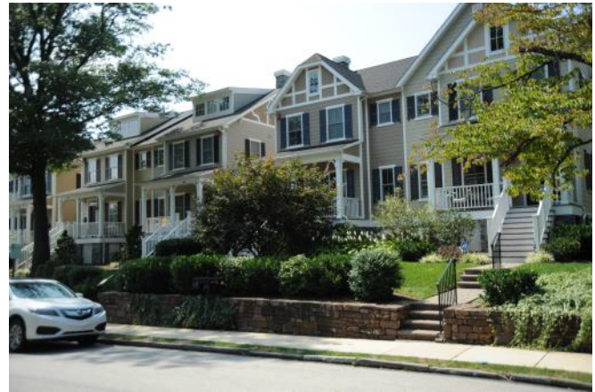
Successful new construction in Haverford Station has maintained a setback, elevation and rhythm similar to that of its immediate neighborhood.
