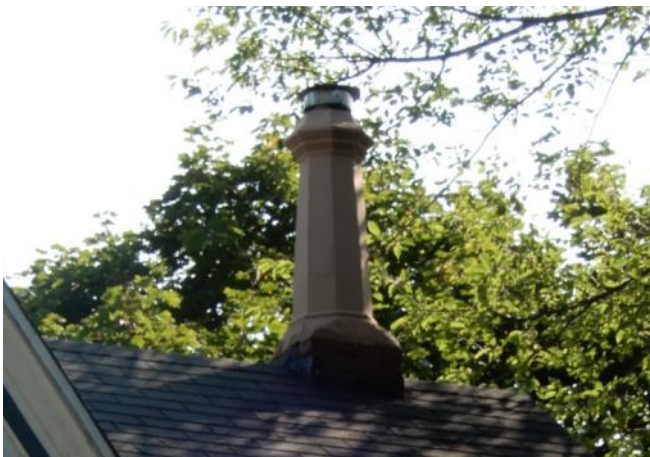
Chimneys pots may be original features of some 19th century homes in Lower Merion and should be preserved, even if they are strictly decorative.
