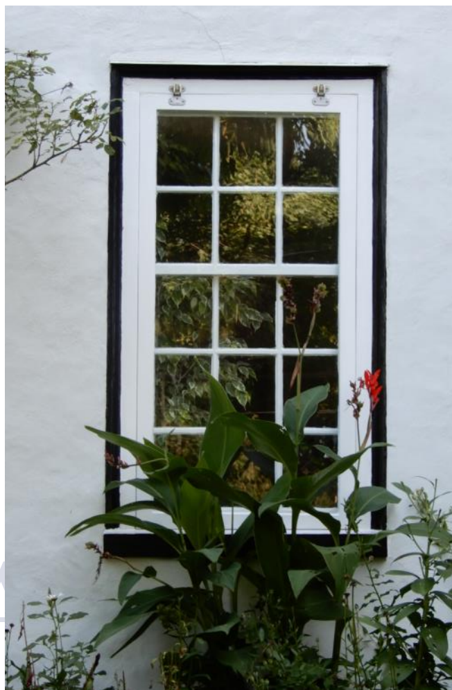
Historic storm windows like this one in Gladwyne were made of wood and were removed seasonally.
