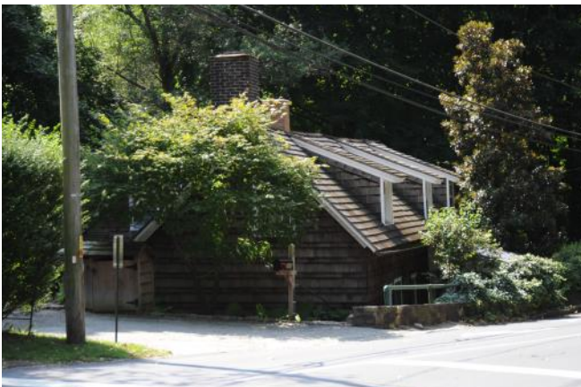
The John Roberts house in the Mill Creek Historic District may be the earliest extant dwelling in Lower Merion.
