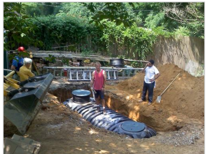
Although invisible after installation, an underground rainwater collection tank requires a property of adequate size and accessibility.
