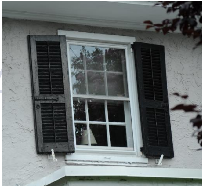
Traditionally shutters were paneled on the first floor and louvered (blinds) on the second floor. Where possible, old shutters should be retained and restored, or if necessary, replaced in kind.
