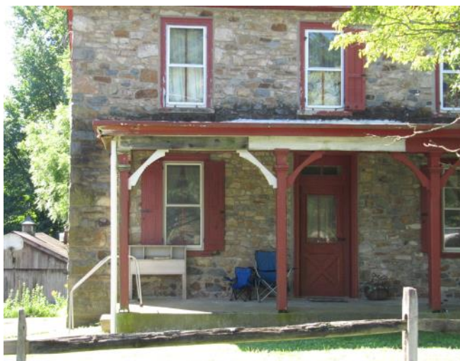
Repair, restoration or replicate components should be employed when character defining features like porch posts and brackets are deteriorated.
