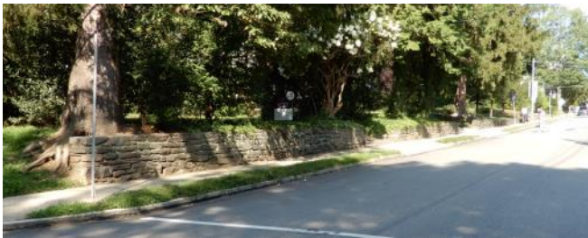
Retaining walls are distinguishing features in several Historic Districts and should be preserved.
