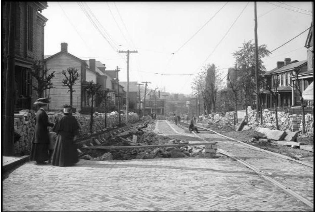
Paving Chartiers Avenue in Elliott, April 28, 1910, view northwest from Lorenz Avenue.
