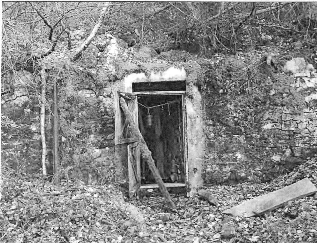
Access door to an upper canyon tunnel, photographed just prior to demolition.
