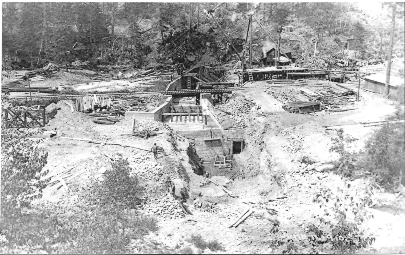
Construction of diversion dam at Maurice.
