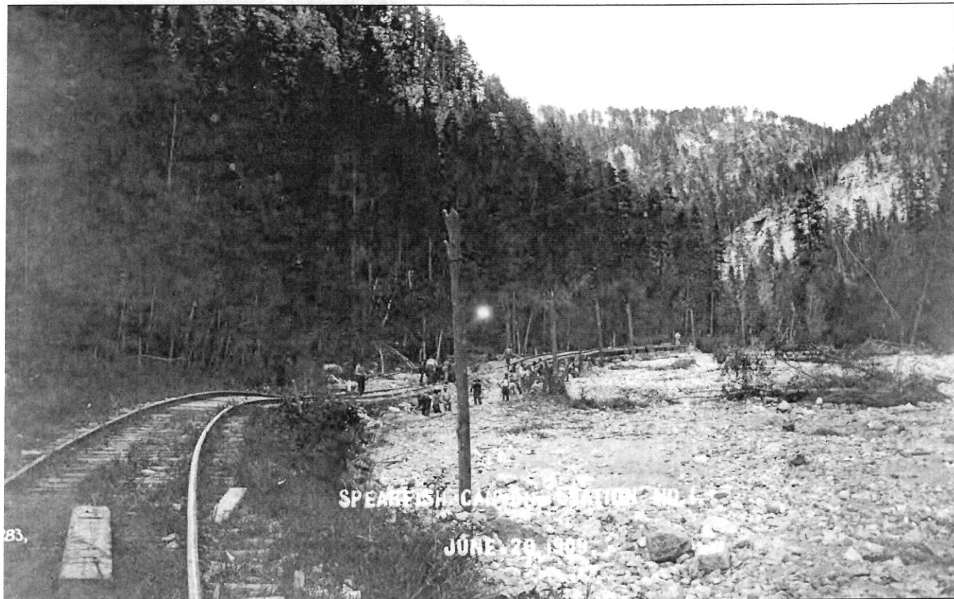
Rail damage after the 1909 flood.
