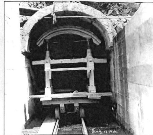
Tunnels were lined with concrete in 1910.
