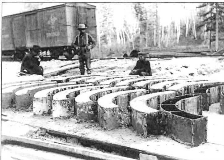
Forms for arched tunnel ceilings.
