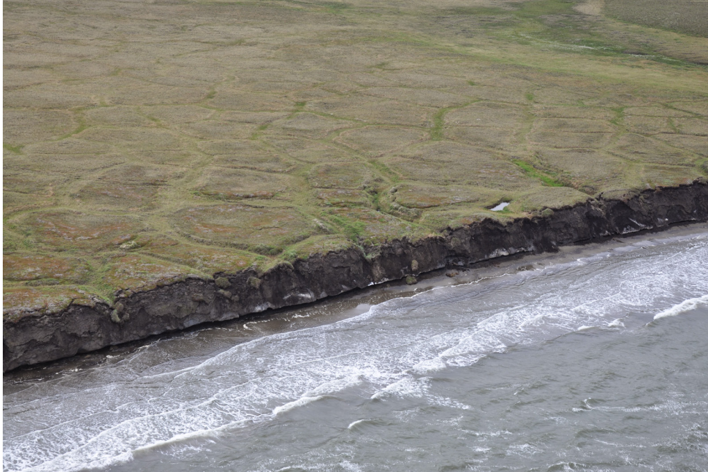
Figure 3. Eroding permafrost bluff along the north coast of BELA between Espenberg and the Kitluk River. This is the shore with most actively eroding permafrost bluffs in BELA. Note the ice (whitish colors) at the bottom of the escarpment, and the shaded notch below where waves have undermined the sediments by thermoerosion (combined erosion and thaw). The beach is narrow here, allowing constant wave action against the scarp. Ice-wedge polygons are visible on the tundra flat above the escarpment. Shorezone (2019) photo nw12_kz_05183 (latitude 66° 35' 9" N, longitude 164° 16' 15" W, 19 July 2012).
