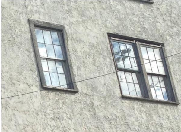
Figure 4 6 over 6 double hung windows
