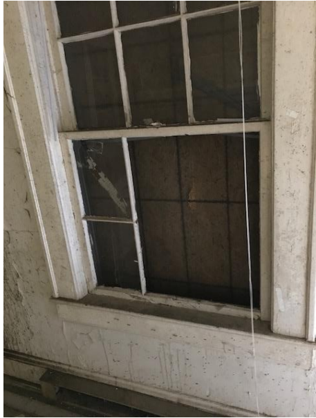
Photo 1 See A2 “Right Courtyard”
