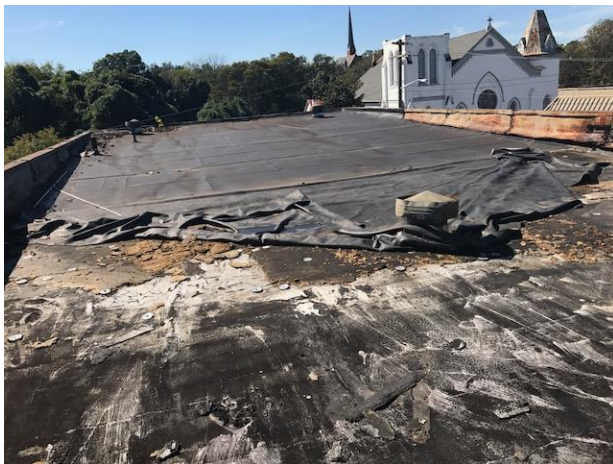
Figure 5 Partial install of new membrane
