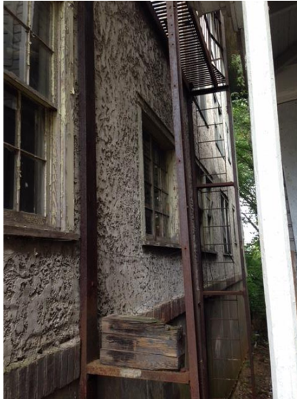
Fire escape and supports below
