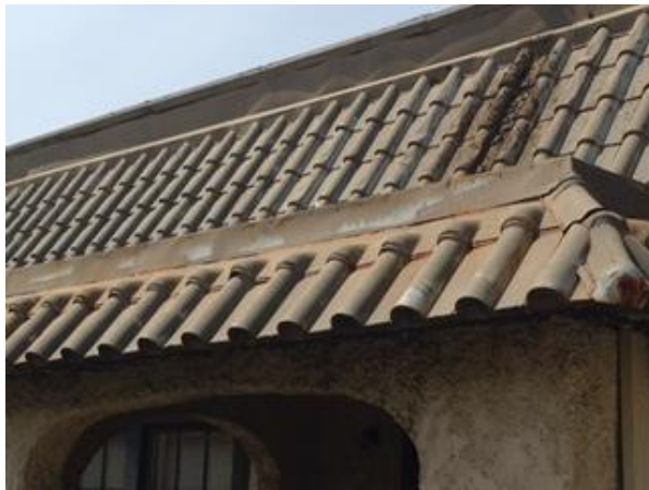
Figure 2 Metal tile roof
