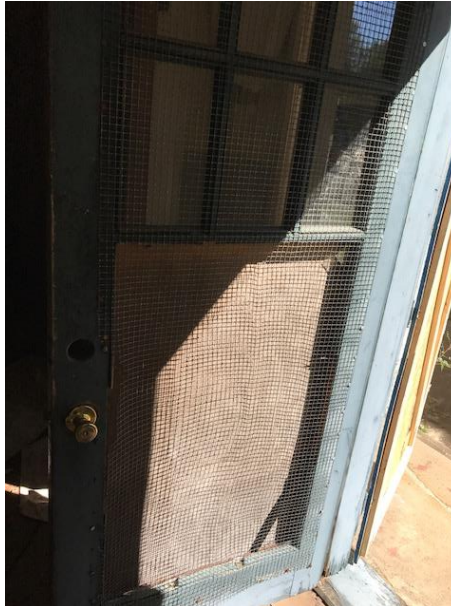
Photo 4 See A3 “Left Courtyard”
