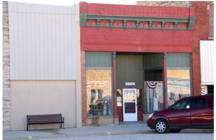
Crawford Plumbing and Tin Shop Building at 139 E. Lincoln is an 1880s one-story building with brick piers and cast-iron columns, and a pressed metal facade and cornice.
