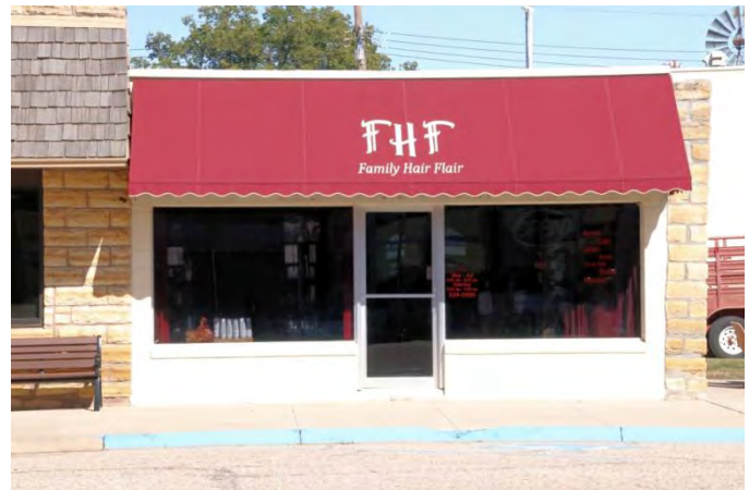
The old Milk Depot/Laundry and Tailor Building at 150 E. Lincoln is a concrete block building with smooth stucco piers and bulkhead around the punched display windows. Built ca. 1945, it is a typical example of the Minimal Commercial style.
