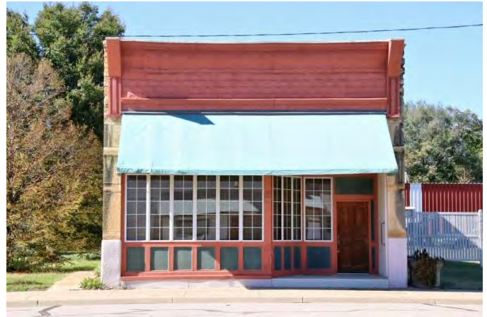
Above and Left: The old Farmers State Bank building at 108 S. Main, is now home to Meyer Land and Cattle. Built ca.1900, it retains pressed-metal detailing and cast-iron columns, both characteristic of the Italianate style.
