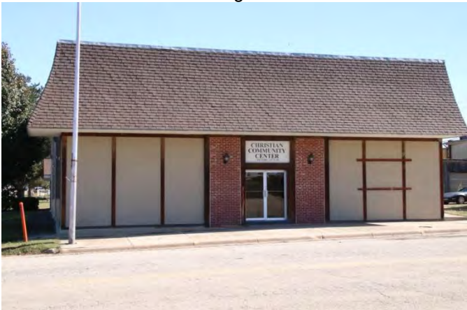
The former Livingood Motor Co. at 137 N. 4 th Street underwent a major remodel in 1970 by the Masonic Lodge, changing the character of the original building.
