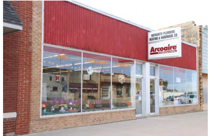
The old Nelson Produce and Creamery Building at 119 E. Lincoln has a replacement aluminum storefront in punched masonry openings typical of the Minimal Commercial style.
