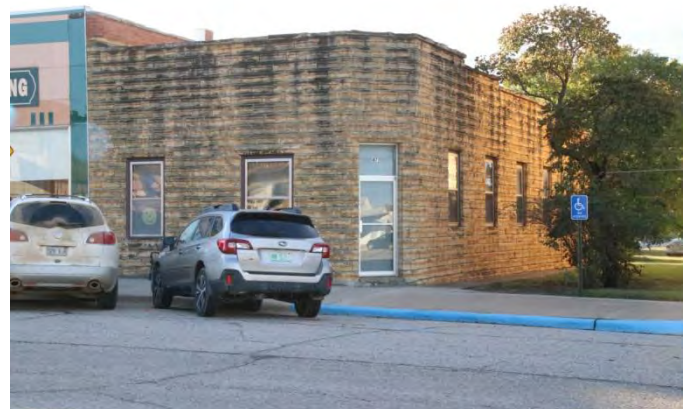
The old Lincoln Sentinel/Republican Newspaper office at 147 W. Lincoln could be classified as a Vernacular design but it is also a different example of a Minimal Commercial style building. Built as a commercial building of native stone in 1915, it has simple punched windows in lieu of a storefront. The canted entry is the only distinctive feature.
