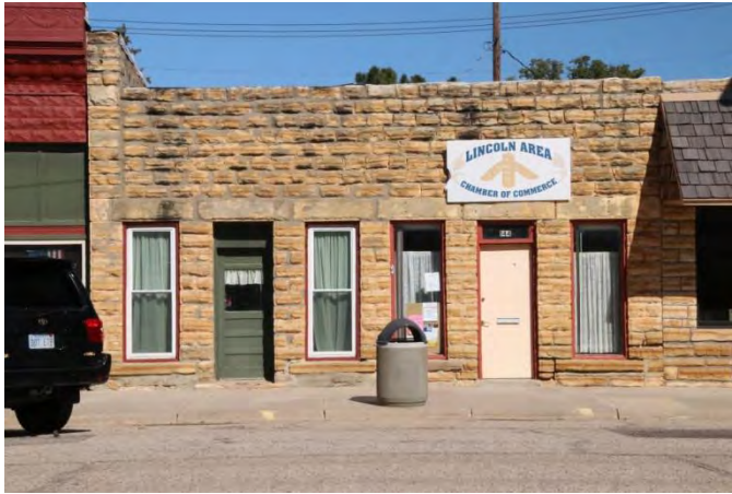
The building at 142-146 E. Lincoln has two small offices, designed and built ca.1905 with doors and windows with large flat stone lintels instead of storefronts.
