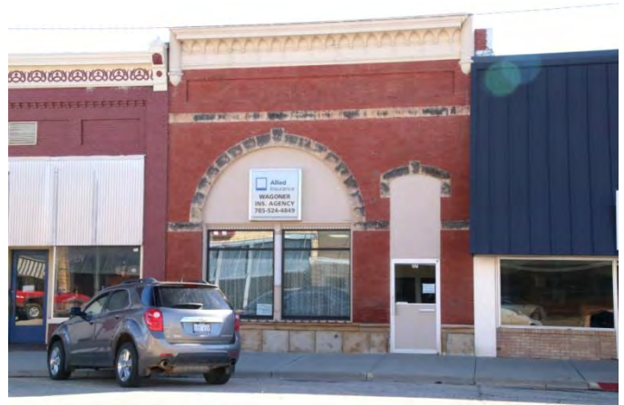
The old Farmers State Bank Building at 117 E. Lincoln has a brick facade dominated by a large arched opening with heavy stone lintel and banding, capped by an ornate metal cornice.
