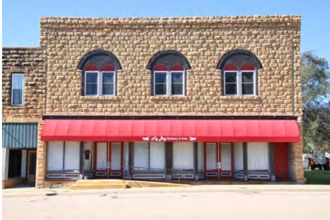
Upper Left: Behrhorst/Lawson Hardware Building built at 105 N. Main in 1905 and the Foster Building built 1913 at 126 N. Main (Upper Right) are characterized by the prominent arched openings typical of the Romanesque style. The Foster Building also retains cast-iron columns along the storefront. Center Right – The old Sylvan State Bank Building is a one-story example of the style and features cast-iron columns at secondary storefronts.
