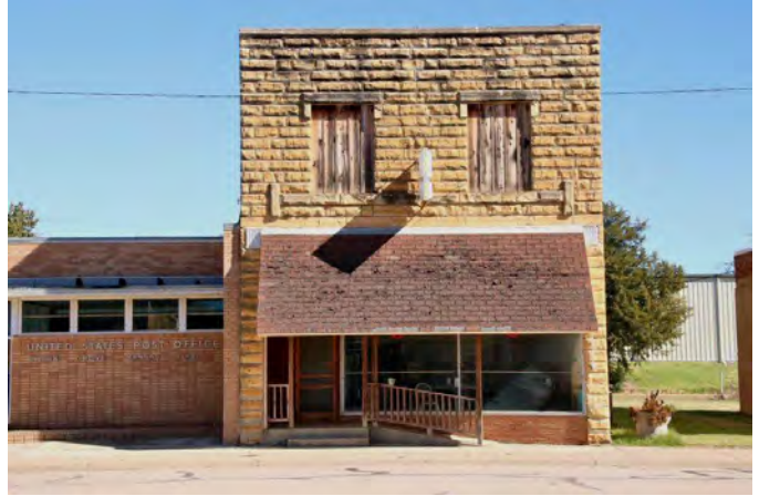
The Stout / Thorpe Bakery Building at 105 S. Main was constructed of stone in 1925 and is a simple example of the Commercial Style. The upper facade is unadorned except subtle detailing at the window sills and lintels. Additionally, the window openings are wider than its tall narrow predecessors. The building is not classified under the Minimal Traditional style because of the detailing at upper windows.
