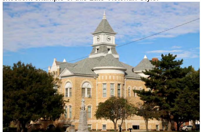
The Lincoln County Courthouse designed by C.W. Squires in 1899 is an excellent example of this Late Victorian Style.
