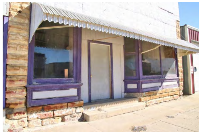
Building at 117 S. Main with pressed metal panels on upper facade and wood storefront on limestone base.
