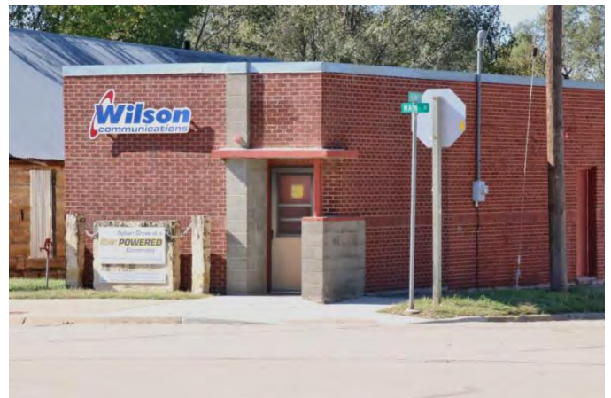
The Wilson Telephone Co. Building was built in 1957 and conveys the basic tenets of the Post-WWII Modern Movement. Concrete blocks contrast with the brick facade to define the entrance at the corner of the building. A flat canopy over the door breaks the vertical block pilaster.
