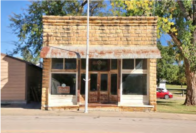
The old Cuddy's Drug Store / Thaemert's Music Store Building is the one of Sylvan Grove's historic commercial buildings with the highest level of historic integrity clearly conveying its original design and construction. Located at 110 N. Main, the free-standing building was built in 1890 and features a limestone base below the storefront as well as a projecting stone cornice. Cast-iron columns frame the recessed central entrance. The building is an excellent example of a One-Part Commercial Block building.
