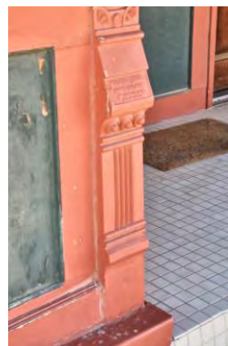
Above and Left: The old Farmers State Bank building at 108 S. Main, is now home to Meyer Land and Cattle. Built ca.1900, it retains pressed-metal detailing and cast-iron columns, both characteristic of the Italianate style.
