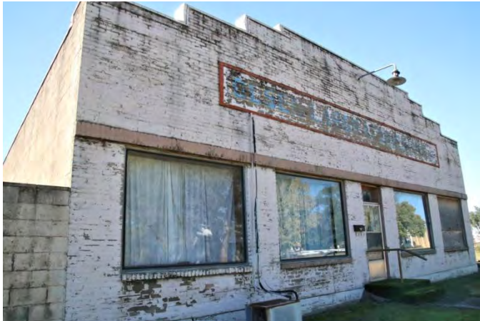
The old Modrow and Holman Repair Shop at 115 W Elm is a more traditional example of the Commercial Style with its brick facade with stepped parapet, brick piers and bulkhead surrounding the display windows.
