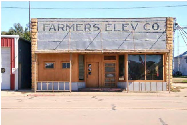
The building above located at 131 S. Main is a typical example of a One-Part Commercial Block configuration where masonry piers and upper facade frame a storefront with large display windows and bulkhead. Stamped metal is located over the masonry above the storefront and used as a signboard in this example. The storefronts may or may not have a transom area above the storefront and there is often an awning above the transom or storefront. The Two-Part Commercial Block is similarly configured but with a second floor that has regularly-spaced windows across the front and is separate and distinct from the lower facade/storefront.
