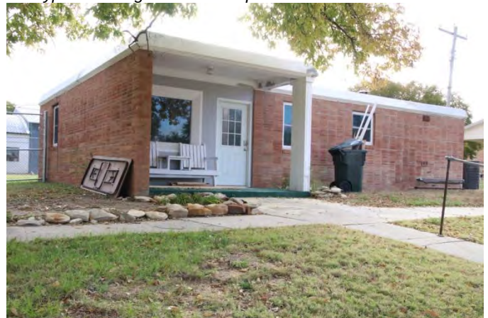
Built in 1950, this one-story office building at 205 S. 5 th Street conveys the Modern Movement with its simple brick facade that has punched openings. A projecting concrete canopy defines the entry bay on the asymmetrical facade.
