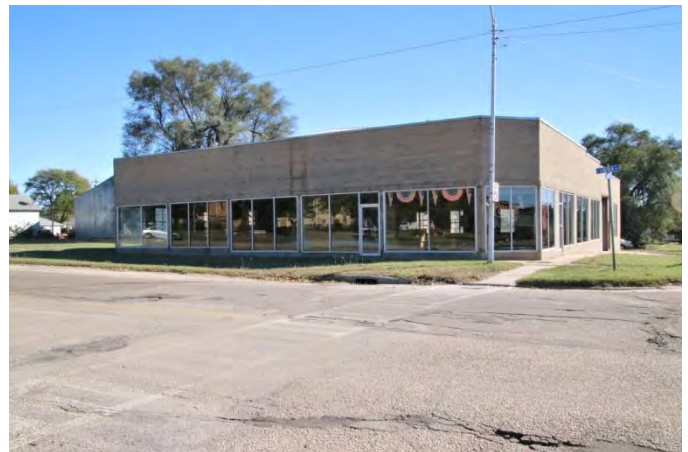
The Chard Motor Co. building at 201 E. Lincoln is a classic example of the post-WWII Modern Movement reflecting the use of new materials in the form of an aluminum-frame storefront that spans two sides of the building with no masonry piers. Built in 1954, the continual ribbon of display windows was typical among car dealerships of this era.
