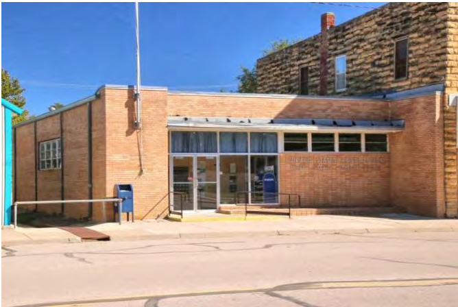
The U.S. Post Office located at 103 S. Main in Sylvan Grove was built in 1961 and is one of the town's best examples of the Modern Movement in Architecture.
