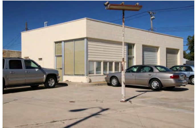
Built in 1950, this concrete block building was a Standard Service Station. Although altered, a distinguishing feature was the aluminum-framed corner display, the only articulation on a plain facade with garage bays.
