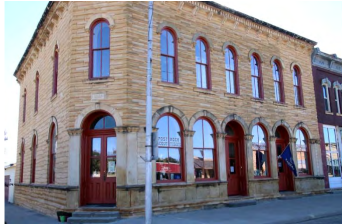
The Cummins Block at 161 E. Lincoln is individually listed in the National Register of Historic Places. It is an excellent example of a two-story commercial building of native limestone with dominant round-arched window openings and a bracketed stone cornice.
