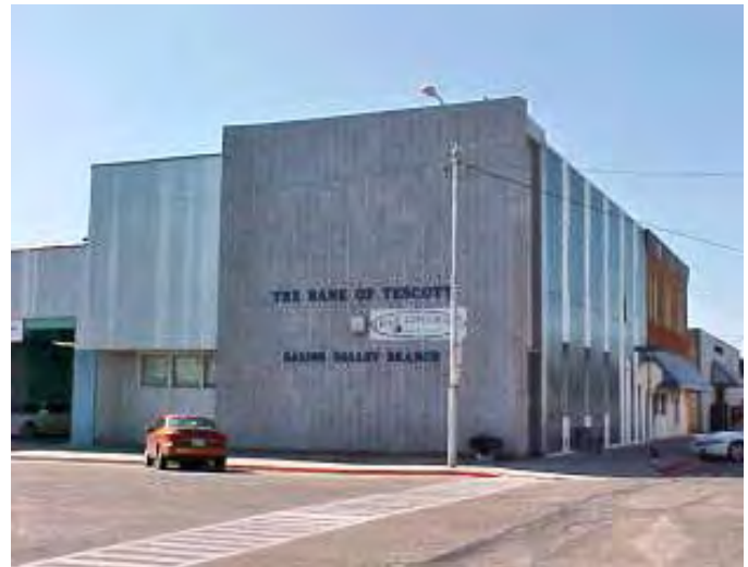
This ca. 1980 view of the Bank of Tescott (former Saline Valley Bank) at 4 th and Lincoln is a typical example of the slipcovers installed in the 1960s-70s obscuring the original facades.
