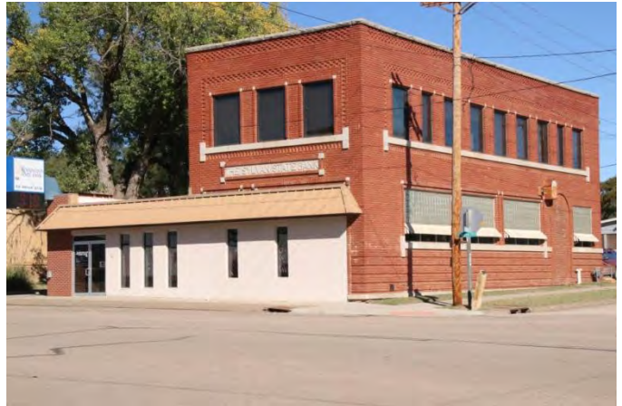
The 1912 Sylvan State Bank Building at 102 N. Main is a traditional example of the Commercial Style executed in brick with brick corbelling and minor stone detailing. Upper windows are wider than the turn-of-the century designs and the corbelled parapet is typical of the style. The stone trim at the window openings is a notable break from the ornate window hoods of the Victorian and Revival styles.
