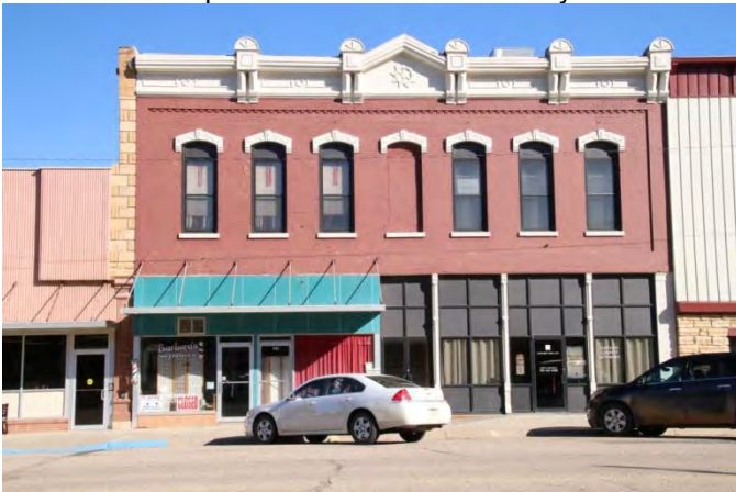
The two-story brick facade at 108 W. Lincoln was home to Hall's Cash Hardware and later Dodd's Hardware. It is a classic Italianate design with ornate metal window hoods and a bracketed metal cornice as well as cast iron columns.
