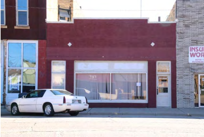
Built in 1940, the one-story brick facade at 145 E. Lincoln is a classic example of the One-Part Commercial Block classification based on building form.
