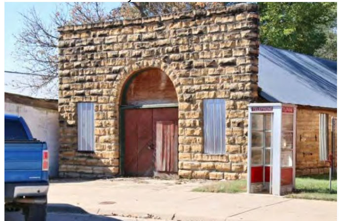
Above - Rohlfe's Blacksmith Shop was built in 1907 at 123 N. Main. It is a gabled-roof structure with a native stone facade.
