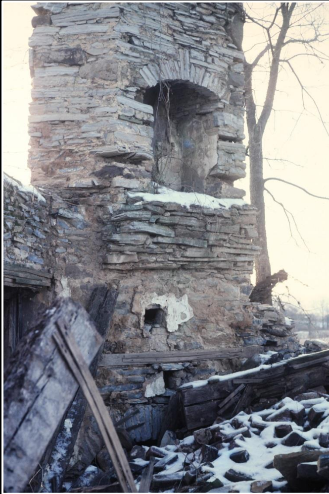
Undated late twentieth century photograph of Mill Pond House, corner chimney detail
