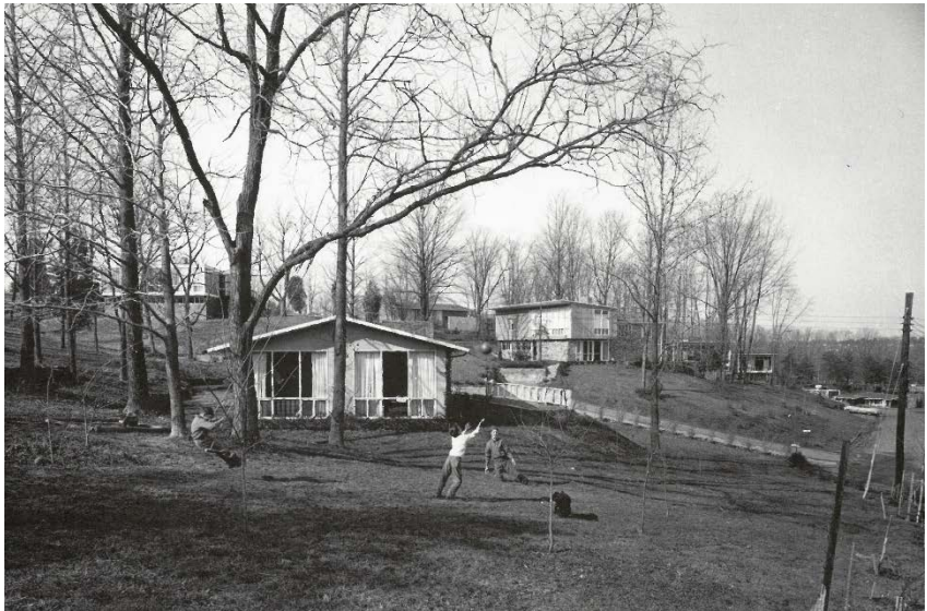
Figure 13: The Goodman-designed houses that comprised the Hollin Hills development were sited to respond to the hilly terrain. [Hollin Hills: Community of Vision, A Semicentennial History, 1949-1999]
