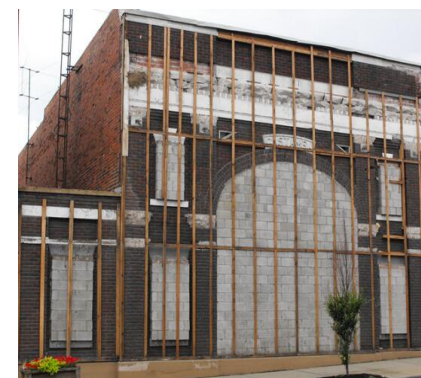
Photo showing the reveal of the historic theatre storefront recently uncovered, present day.
