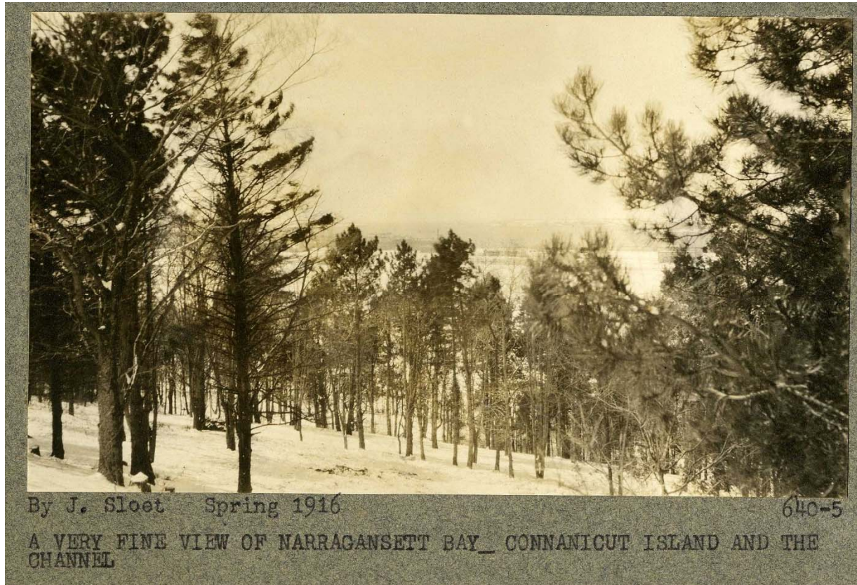
Job # 00640, A. P. Stokes, Miantonomi Hill, Photo 5. Courtesy of the National Park Service, Frederick Law Olmsted National Historic Site.
