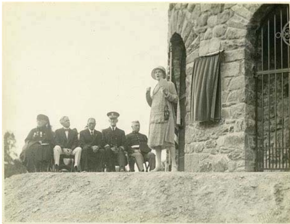
1929 Dedication of the Miantonomi Park Tower (Collection of the Newport Historical Society)
