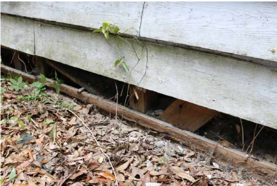
Figure 48: North Elevation of Two-Story Building: Detail of corner brace intersecting the deteriorated north perimeter sill.
