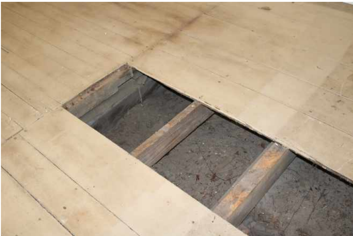
Figure 57: Crawlspace Below Room 103: Overview of differently sized floor joists.
