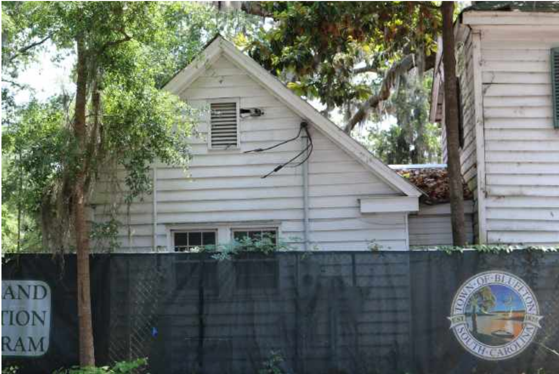
Figure 31: North Elevation, One-Story East Building.
