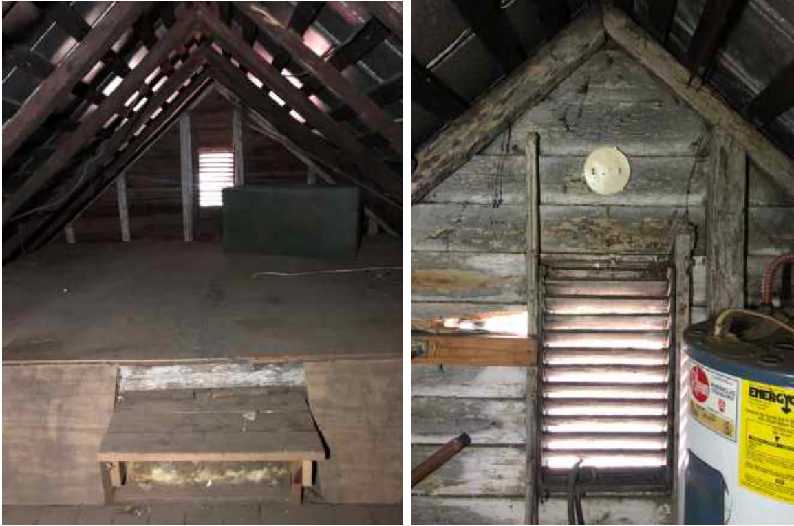
Figure 107: Attic of the One-Story Building: Overview of the roof framing looking south (at left) and north (at right).
