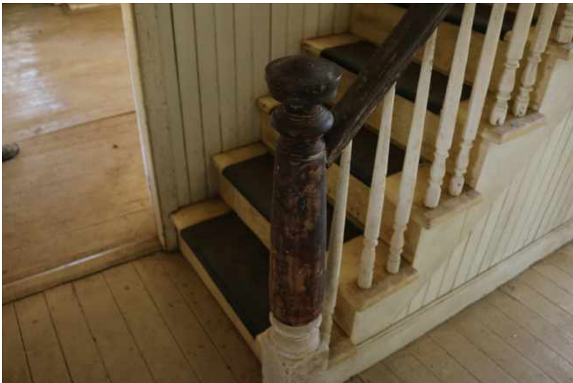
Figure 87: Room 102, Stair-Hall: Detail of the newel post and balustrade.
