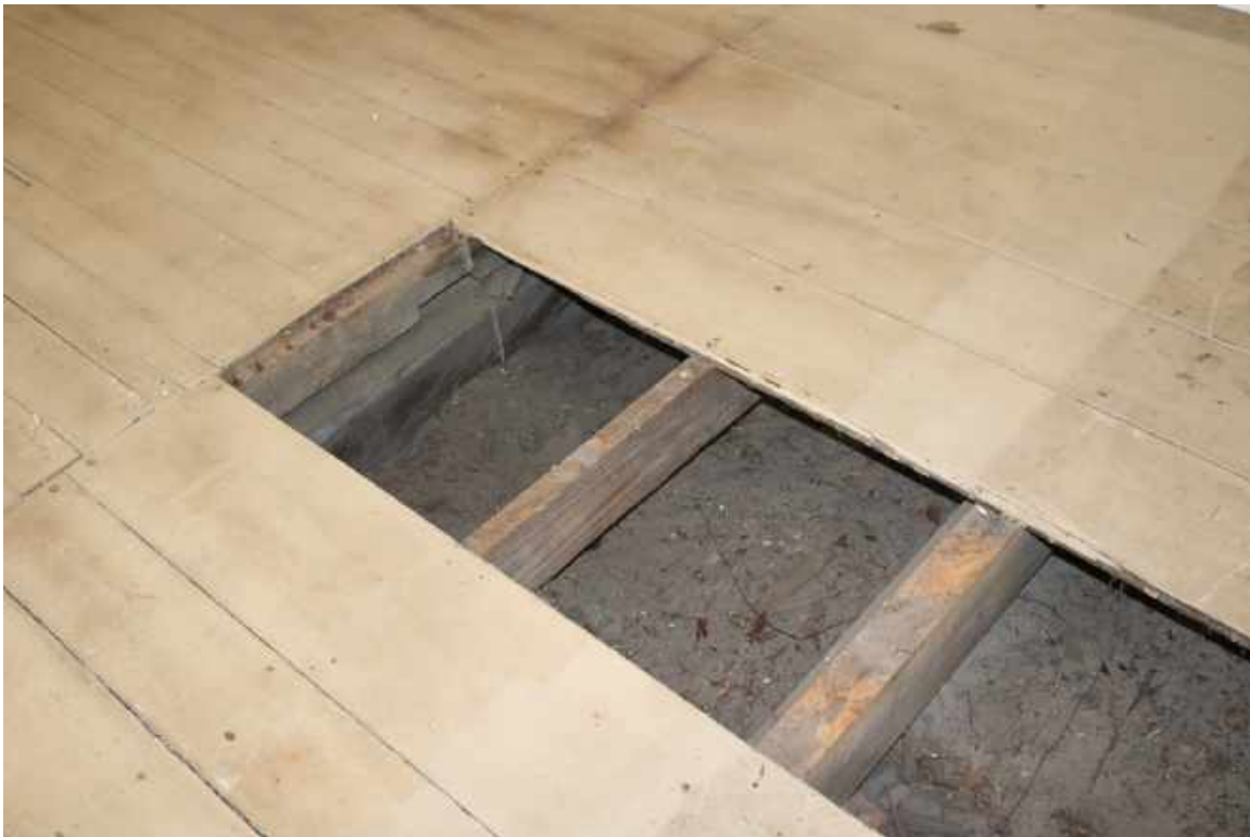
Figure 121: First Floor, Room 103: Detail of flooring removed at the center of the room, exposing the original first floor framing and later repairs.
