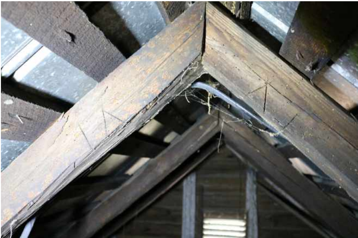
Figure 108: Attic of the One-Story Building, Looking North: Detail of matching carpenter's marks.
