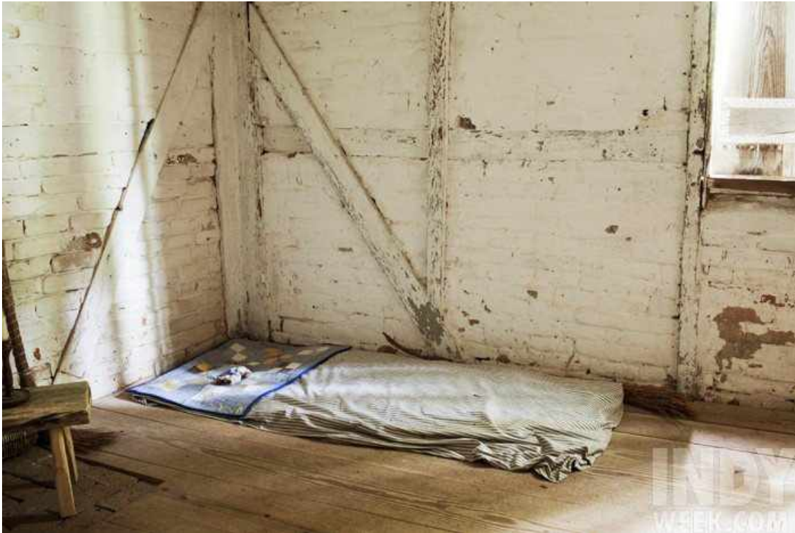
Figure 131: Interior of Horton's Grove slave cabin. The interior has been whitewashed similar to that seen at the Squire Pope Carriage House. Unlike at Squire Pope, the space between the framing members has been infilled with masonry (NCpedia.org).
