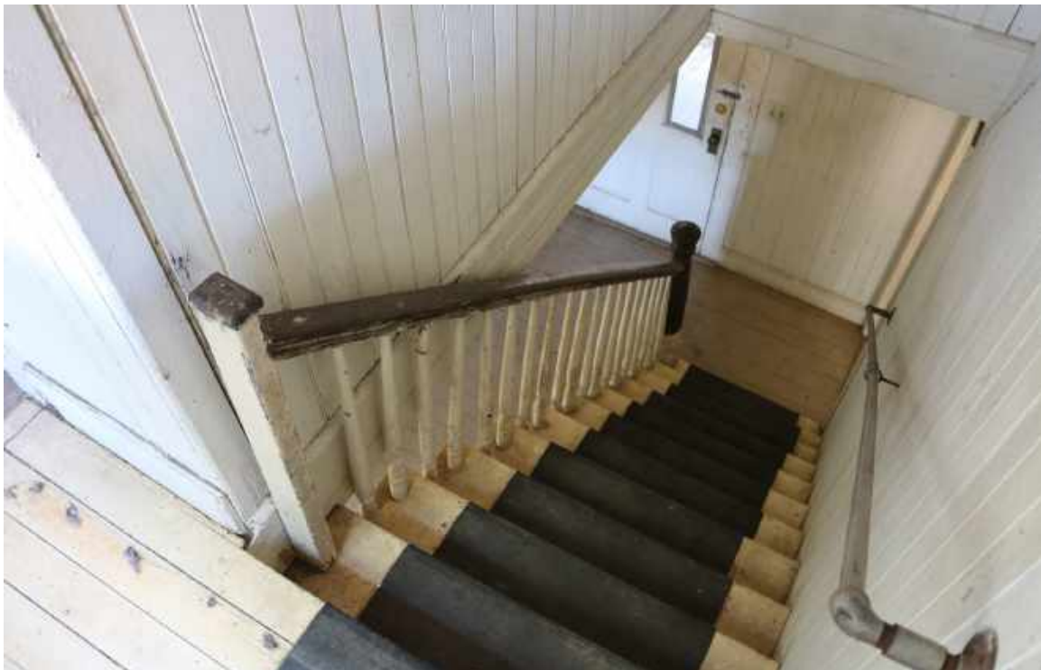
Figure 99: Room 203, Stair-Hall: The landing on the second floor is narrow. Thinner tongue and groove floors are installed over older flooring boards.
