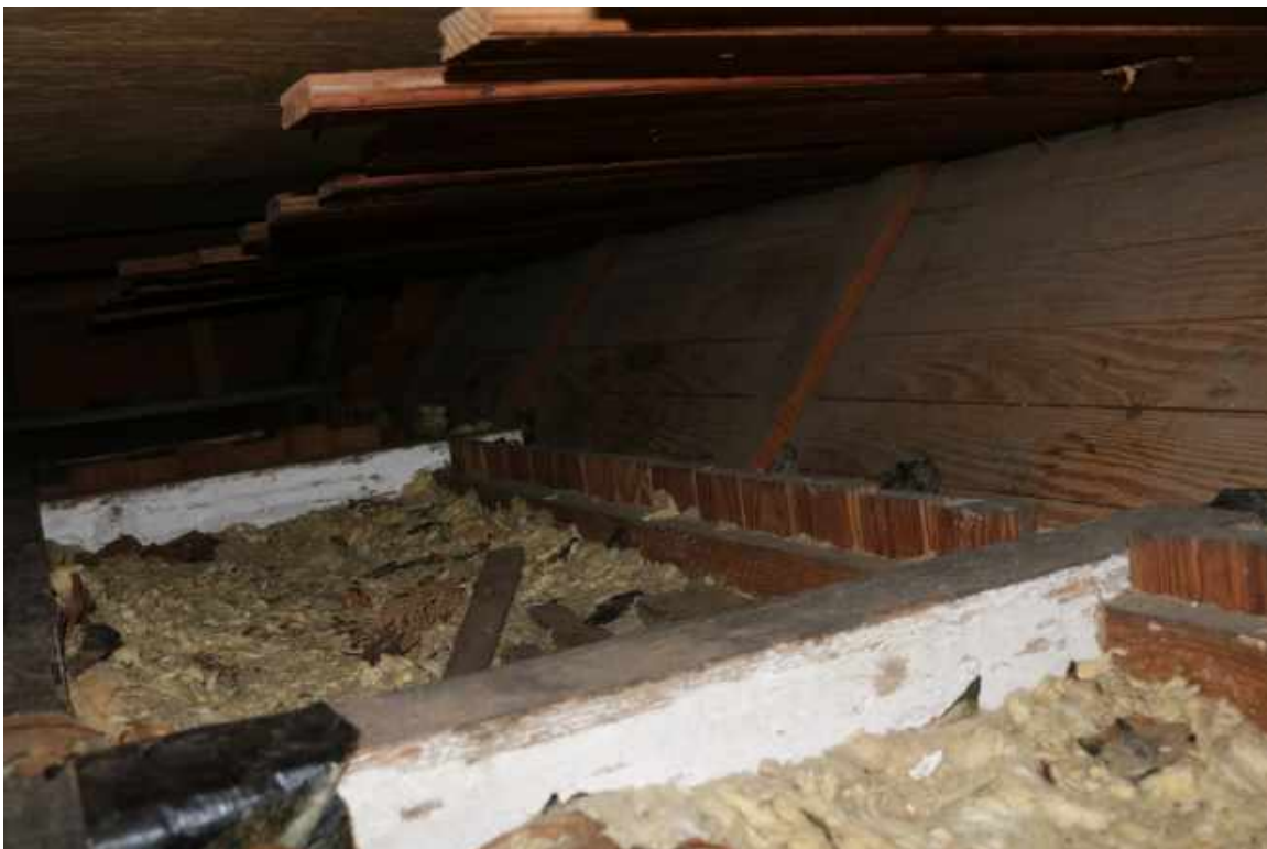
Figure 114: Attic of Two-Story Building, Beneath Plywood Floor: The second-floor ceiling joists have been cut to accommodate the installation of the cant ceiling.
