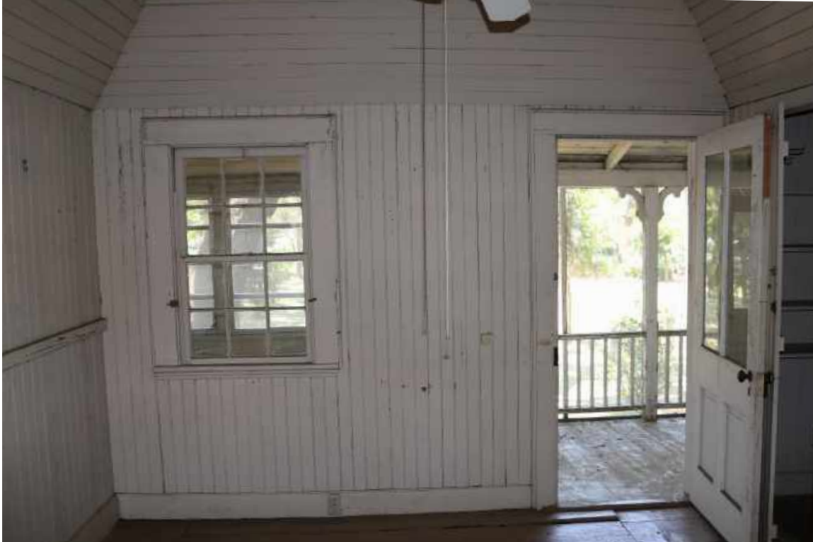
Figure 100: Room 204, Looking South Towards Porch: This room is finished in a similar fashion to Rooms 202 and 205.
