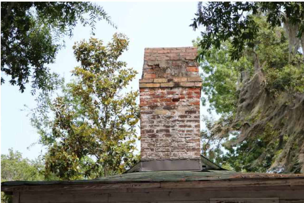
Figure 79: West Elevation of the Two-Story Building: The chimney at this elevation is believed to be the oldest on the house. The upper cap has been modified as evidenced by the change in brick color.
