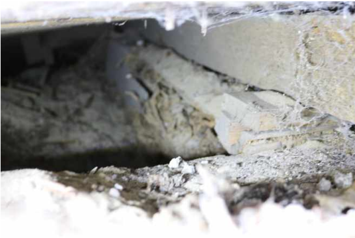
Figure 50: Crawlspace Beneath Room 101, Northwest Corner: Detail of deteriorated western perimeter sill. The settlement in this area is due to the failure of this structural member.
