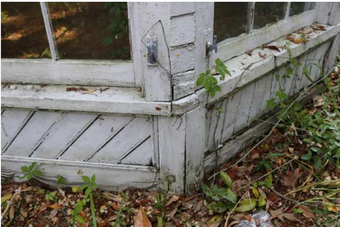
Figure 52: South Elevation of One-Story Building: Detail of the foundation of the bay window. The decorative paneling is extensively deteriorated.
