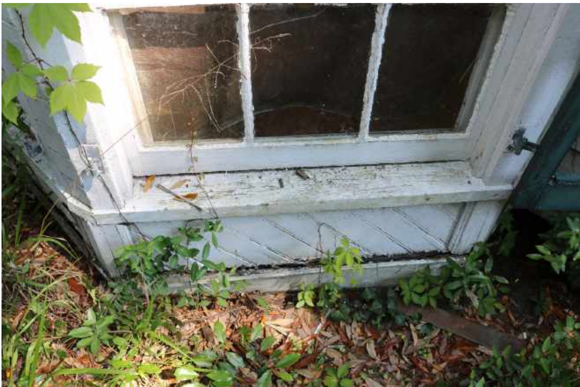
Figure 67: South Elevation of One-Story Building: Detail of window and trim deterioration within the south bay window.
