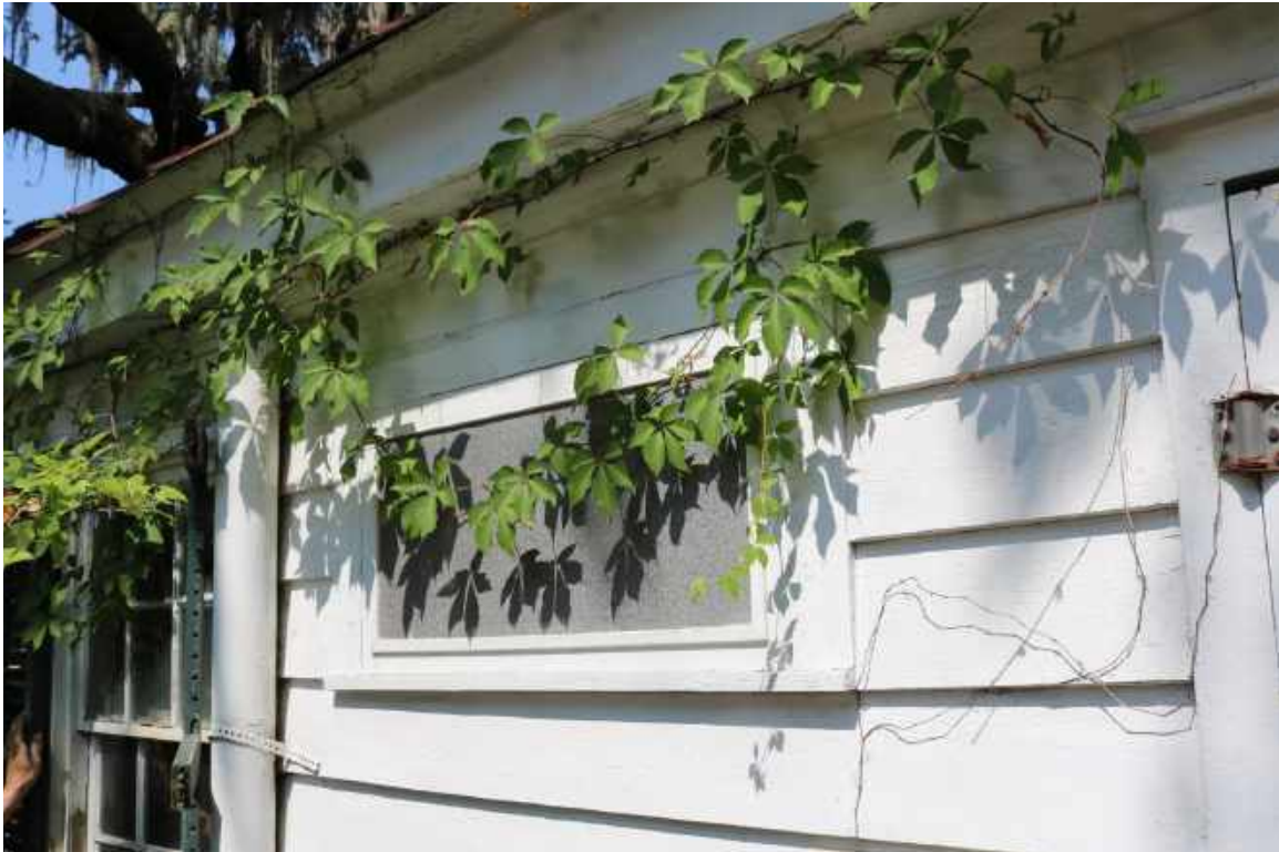
Figure 66: East Elevation of One-Story Building: Detail of transom window.
