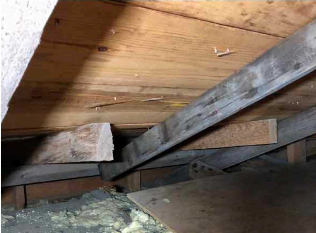
Figure 183: Attic: Detail of newer porch roof framing intersecting the historic rafters.
