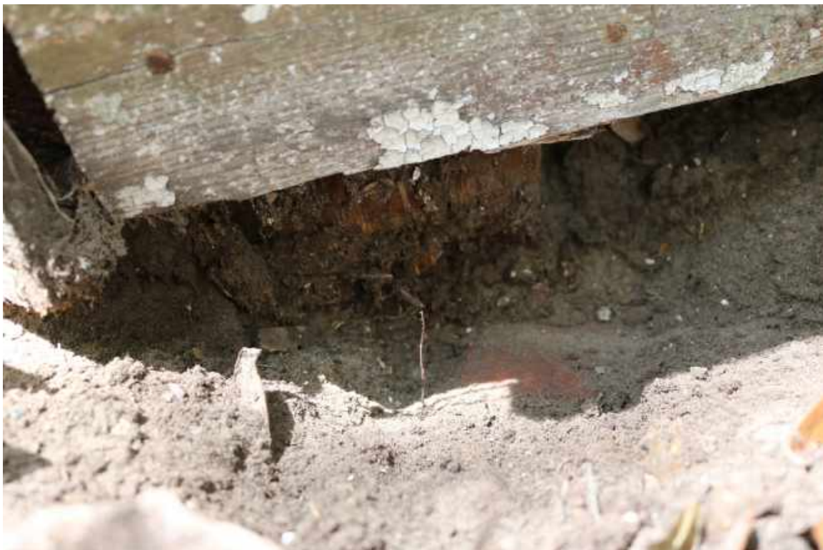
Figure 142: South Elevation, One-Story Kitchen Building - Detail of the deteriorated lower end of a vertical framing member.
