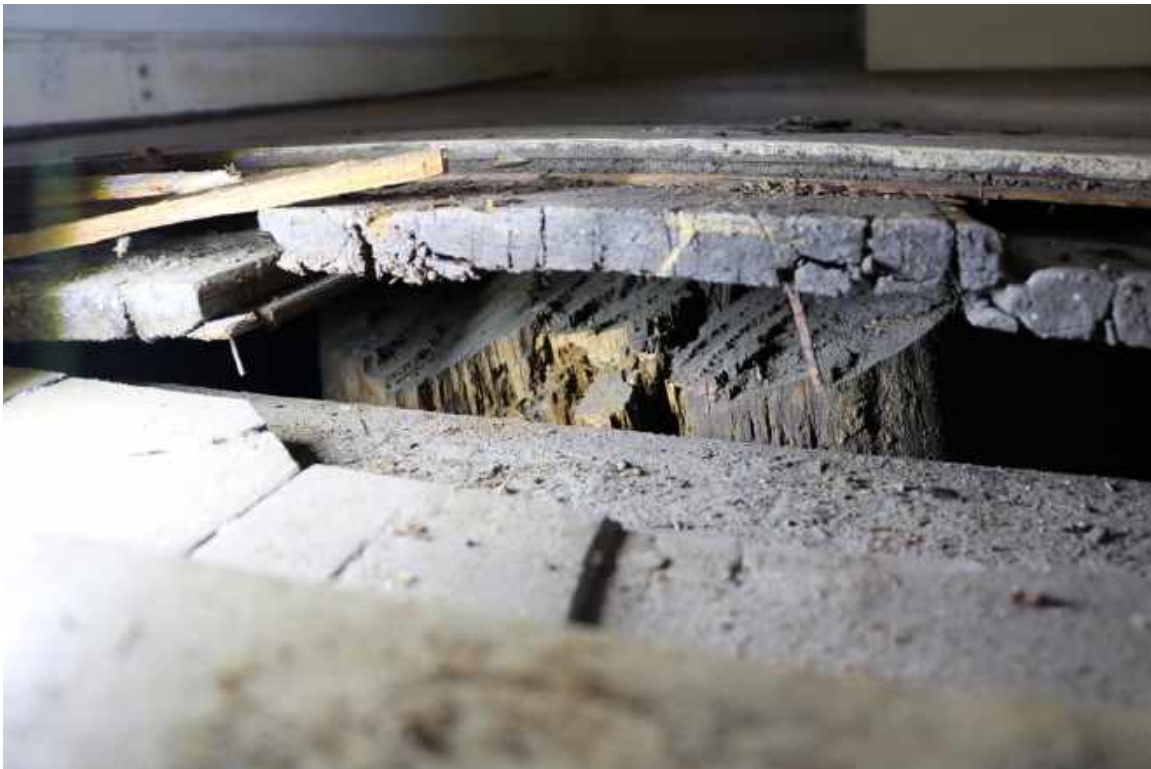
Figure 118: First Floor, Room 101: A deteriorated tree stump was found between two joists at this location.
