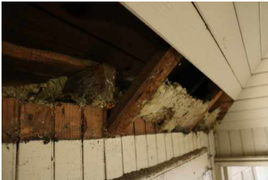
Figure 175: Photograph of Room 204. Detail view of transition between wall board and cant at the uppers section of the wall. The ceiling joists in this area were modified to elevate the ceiling height. A cant, at the top of the wall, appears to have been installed at this time
