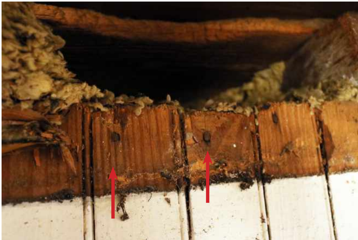
Figure 129: Second Floor, Room 204: Detail of cut nails in the vertical paneling (arrows).
