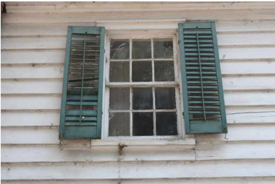
Figure 62: North Elevation of Two-Story Section: Overview of the historic second-floor single hung gunstop windows and louvered shutters.
