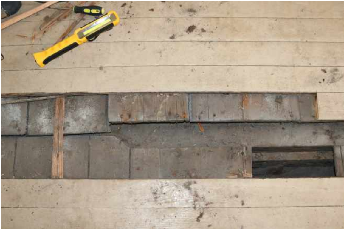
Figure 116: First Floor, Room 101: Large wide plank flooring was uncovered directly beneath the existing small plank flooring. The underlying floor is fastened directly to the joists and is interpreted to be original.
