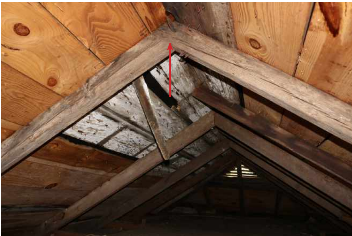
Figure 110: Attic of Two-Story Building: Detail of transition between pegged (arrow) and toenailed rafters (behind). Reclaimed floorboards have been used as decking at this location. The reclaimed material is deteriorated.
