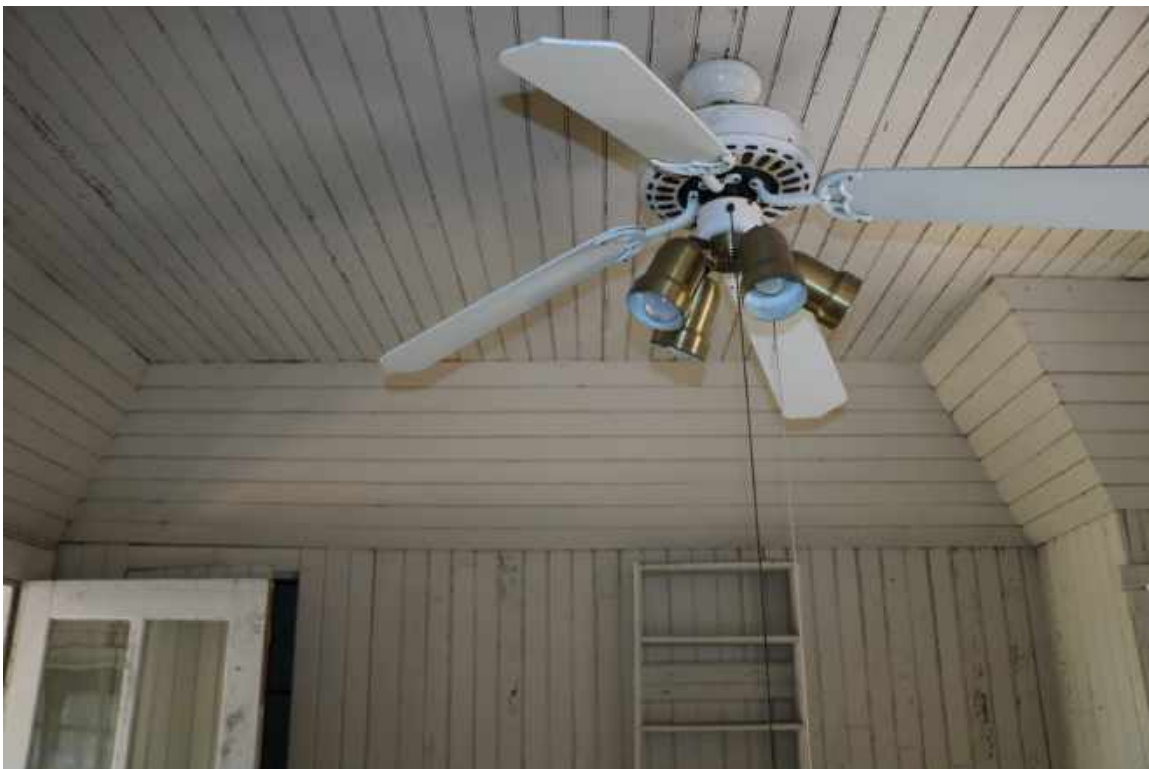
Figure 101: Room 204, Looking West: Detail of ceiling paneling.
