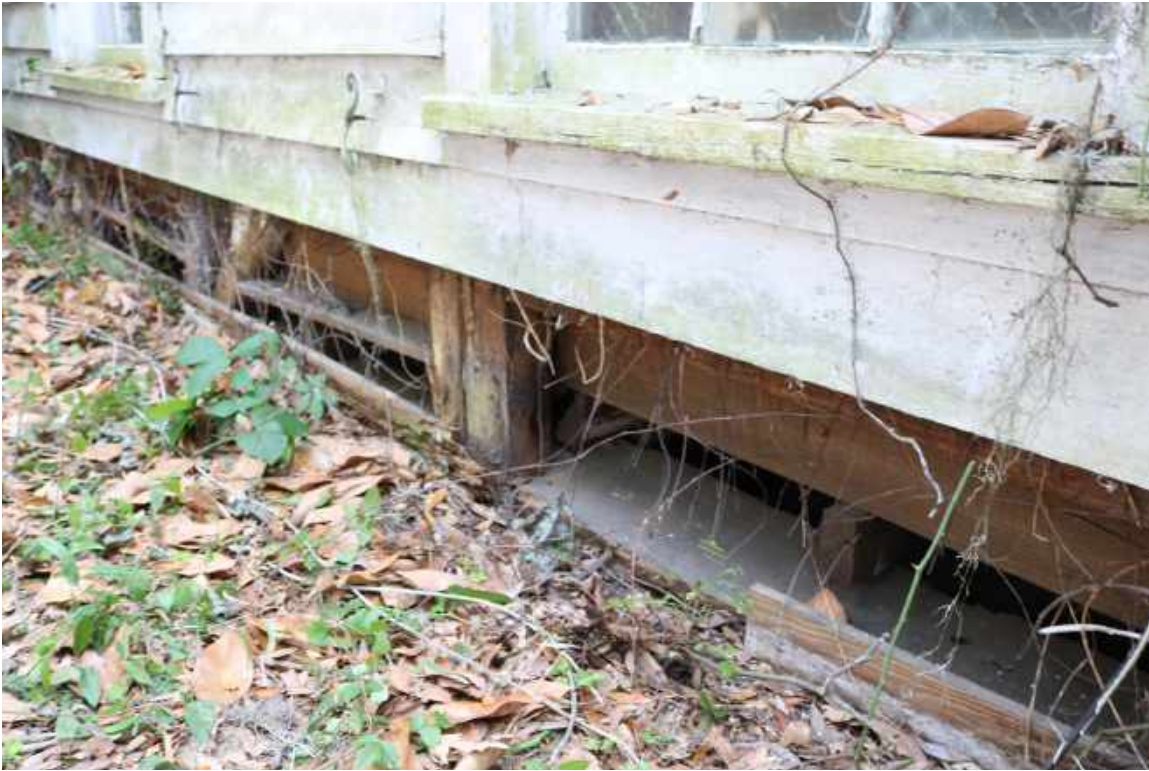
Figure 47: North Elevation of Two-Story Section: Detail of framing members at grade level to the west of the north chimney.
