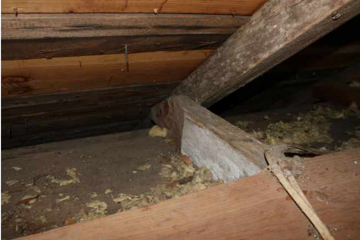
Figure 113: Attic of Two-Story Building: Modern plywood has been installed over whitewashed collar ties
