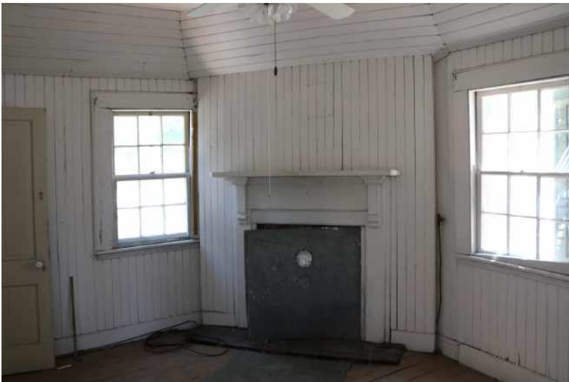
Figure 103: Room 205, Northeast Corner: Detail of the interior finishes within this room.
