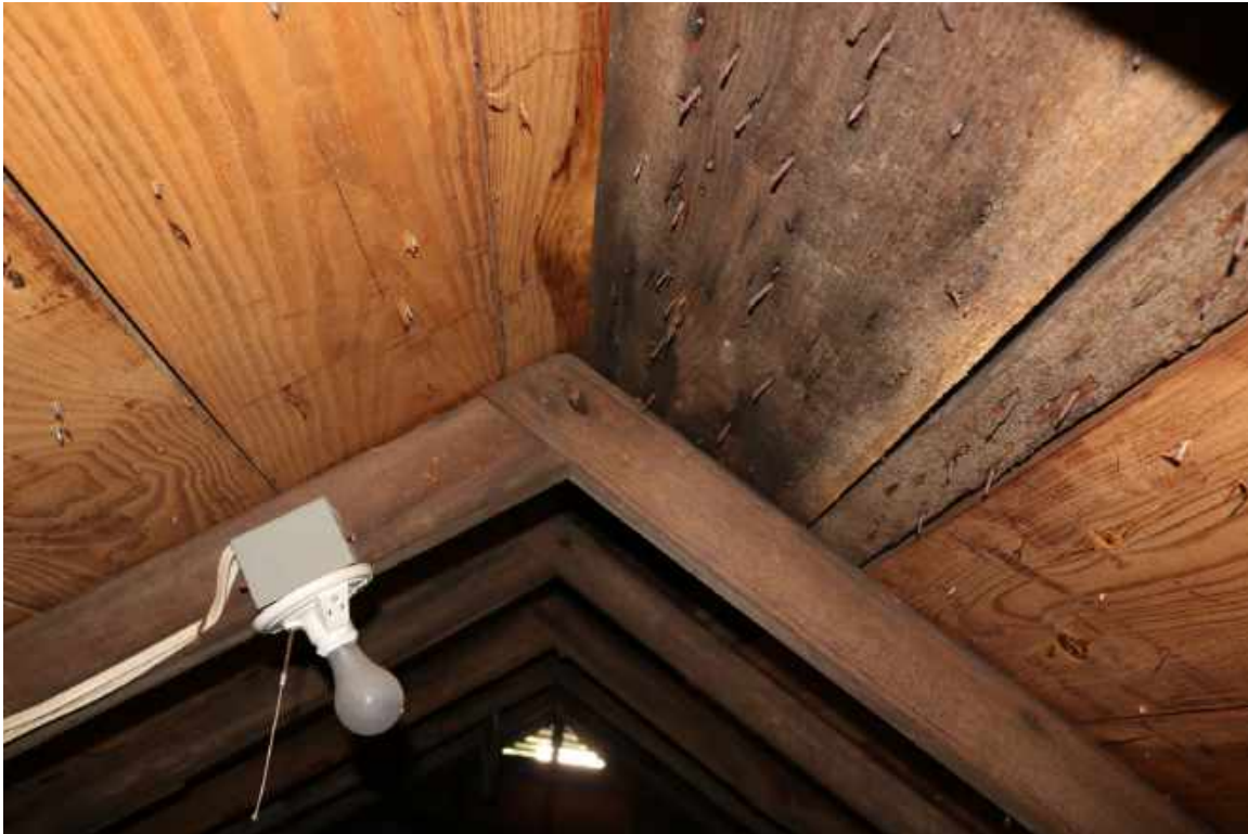
Figure 109: Attic of Two-Story Building: The western rafters are joined together with pegs at the ridge. Much of the roof decking has been replaced.
