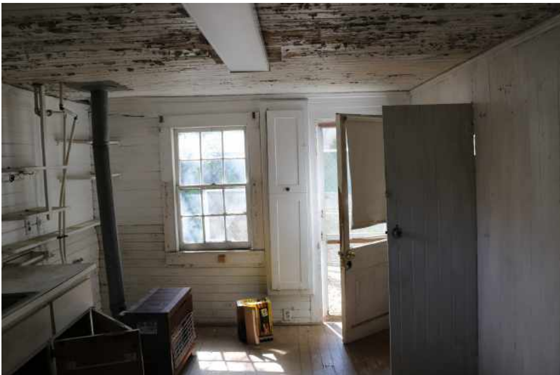
Figure 92: Room 105 (Kitchen) Looking East: There is extensive paint failure within this room.
