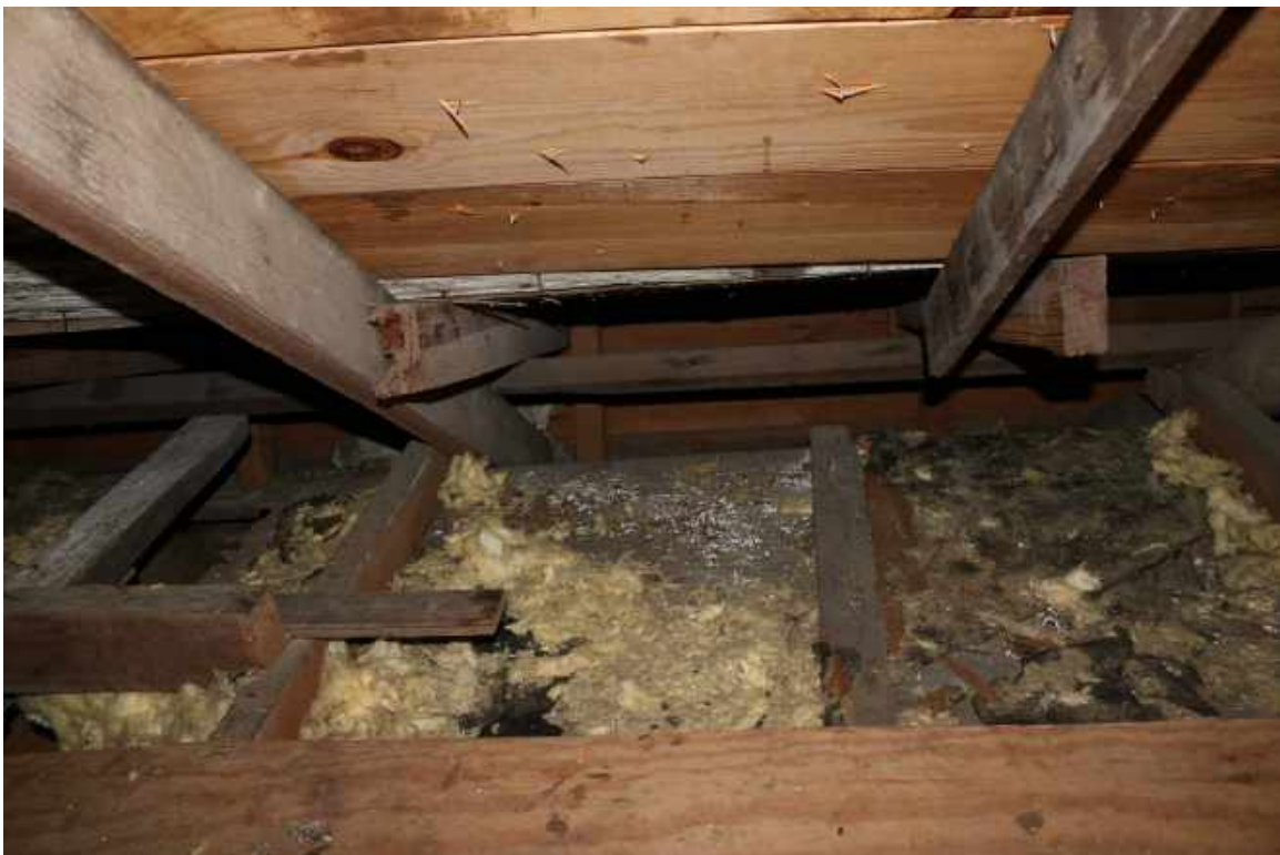
Figure 112: Attic of Two-Story Building, Looking South: The rafter tails from the porch framing rest adjacent to the historic roof framing. The porch framing is modern and the rafter ends are deteriorated at select locations.
