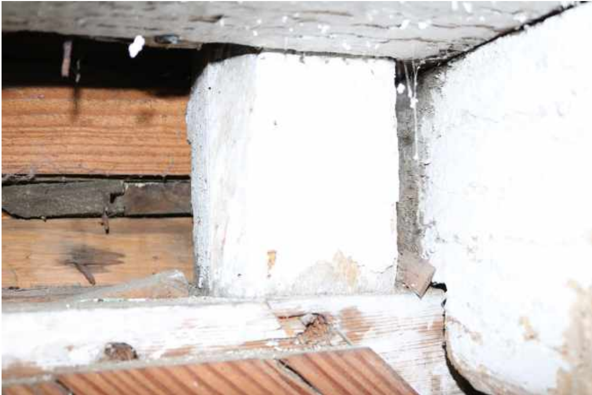
Figure 125: Second Floor, Room 204: Detail of a stud on the south elevation showing the presence of the whitewash on the girt, joist, and stud.
