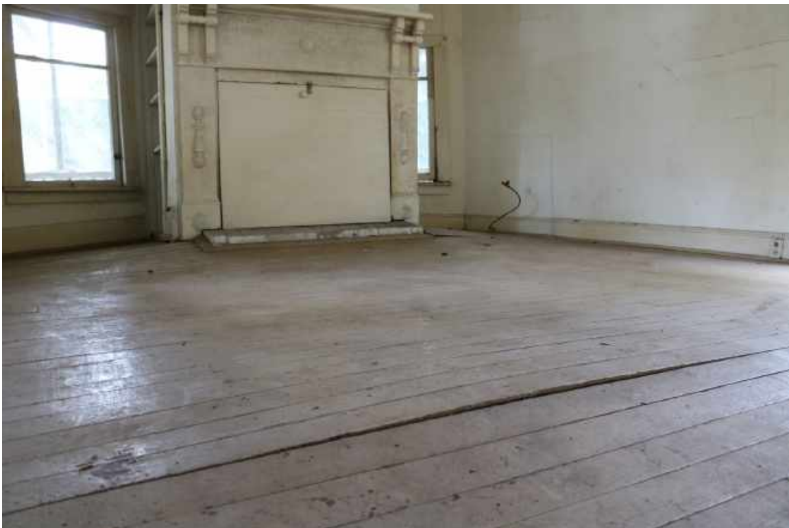
Figure 115: Room 101: Detail of flooring conditions prior to selective disassembly.
