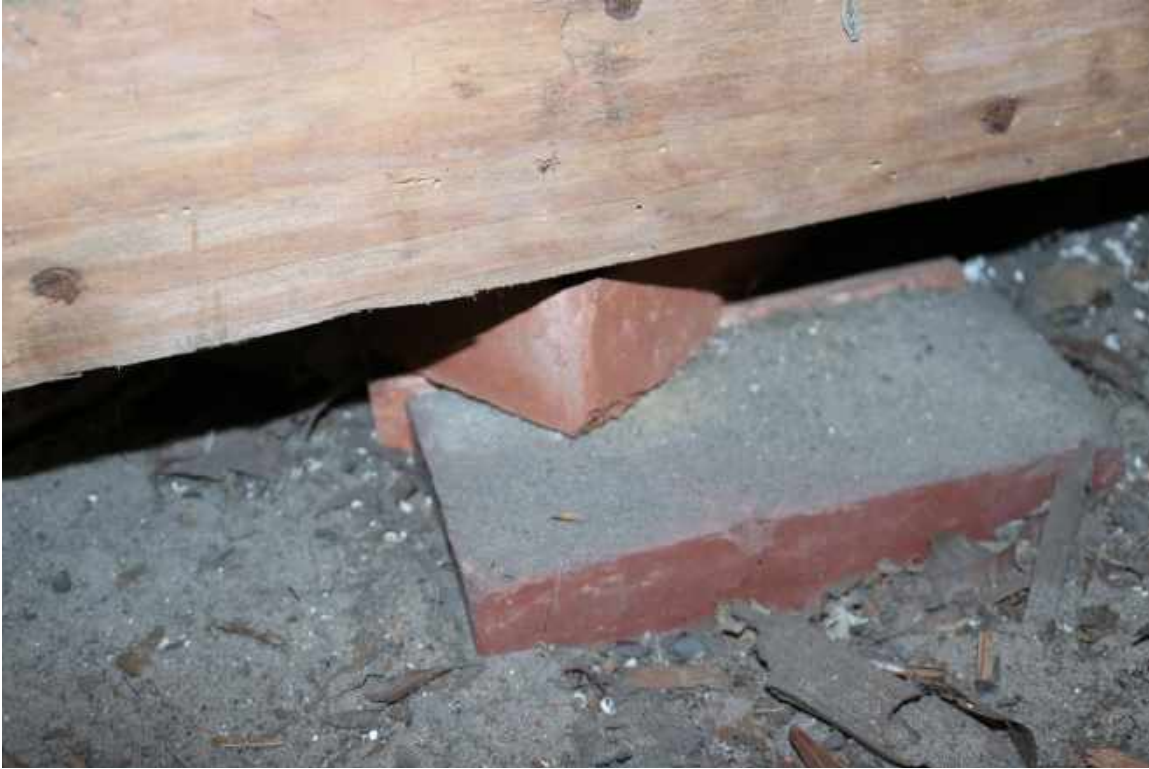
Figure 49: Crawlspace beneath Room 103: Detail of dry stacked modern masonry installed below floor joist.
