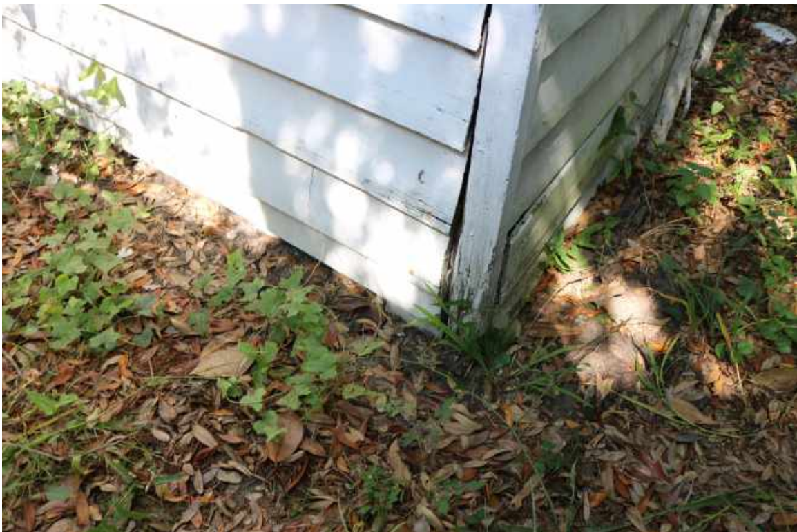
Figure 69: South Elevation of One-Story Building: Detail of siding failure due to corrosion of the steel fasteners.
