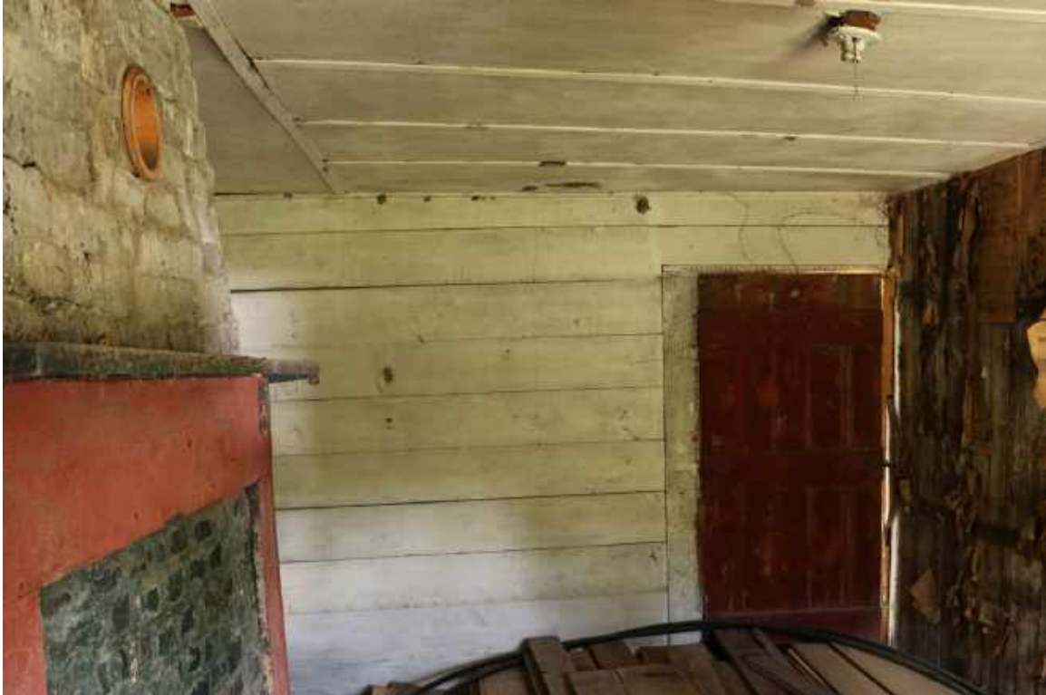
Figure 133: Interior of Friendfield Plantation outbuilding. The interior face of the siding and framing members have been whitewashed similar to Squire Pope.
