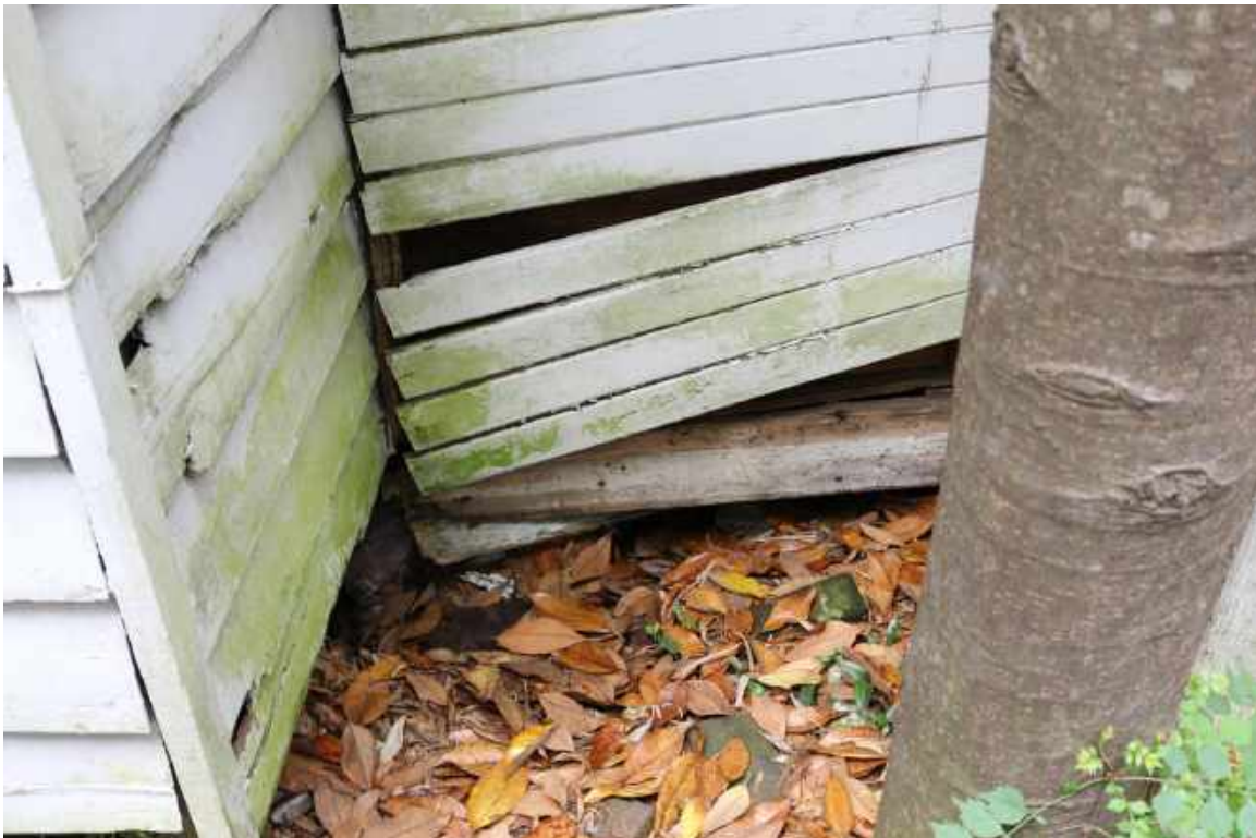
Figure 54: North Elevation, Hyphen: The foundation of the hyphen has failed.
