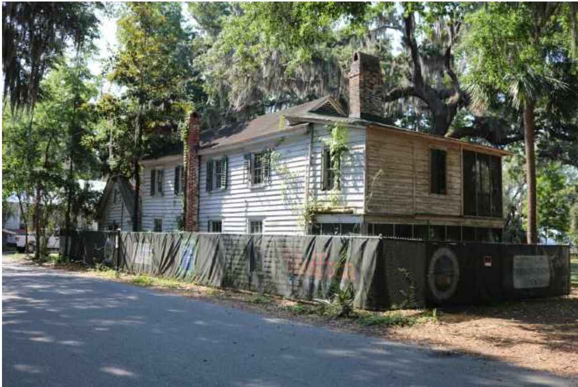
Figure 43: Squire Pope Carriage House, Northwest Corner: Overview of existing exterior conditions.
