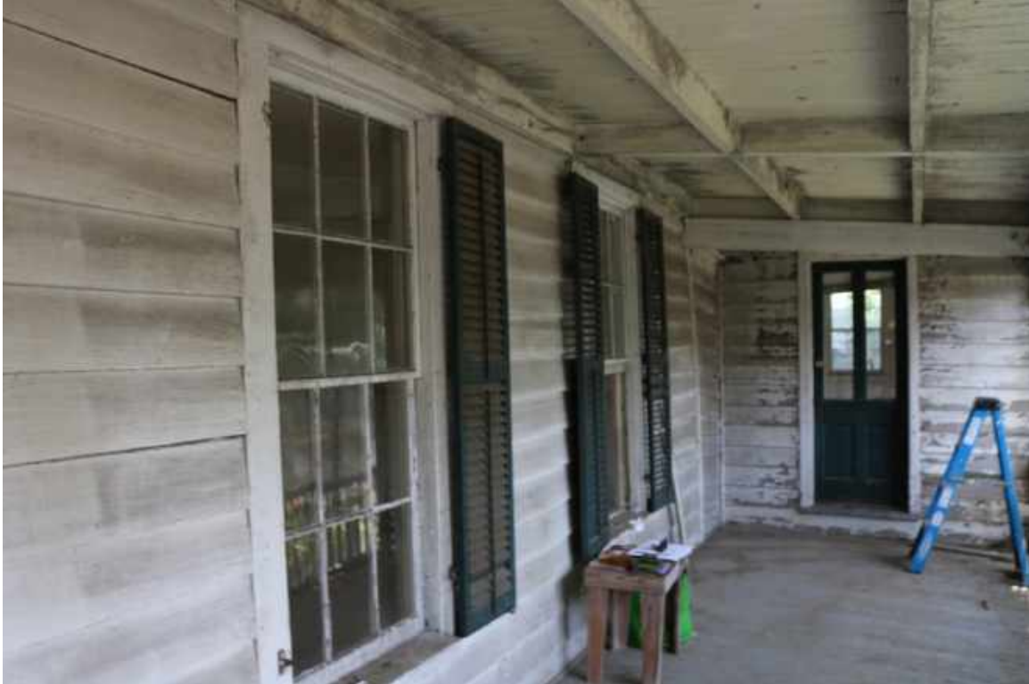
Figure 61: South Elevation of Two-Story Section: Overview of the historic first-floor single hung gunstop windows and louvered shutters.
