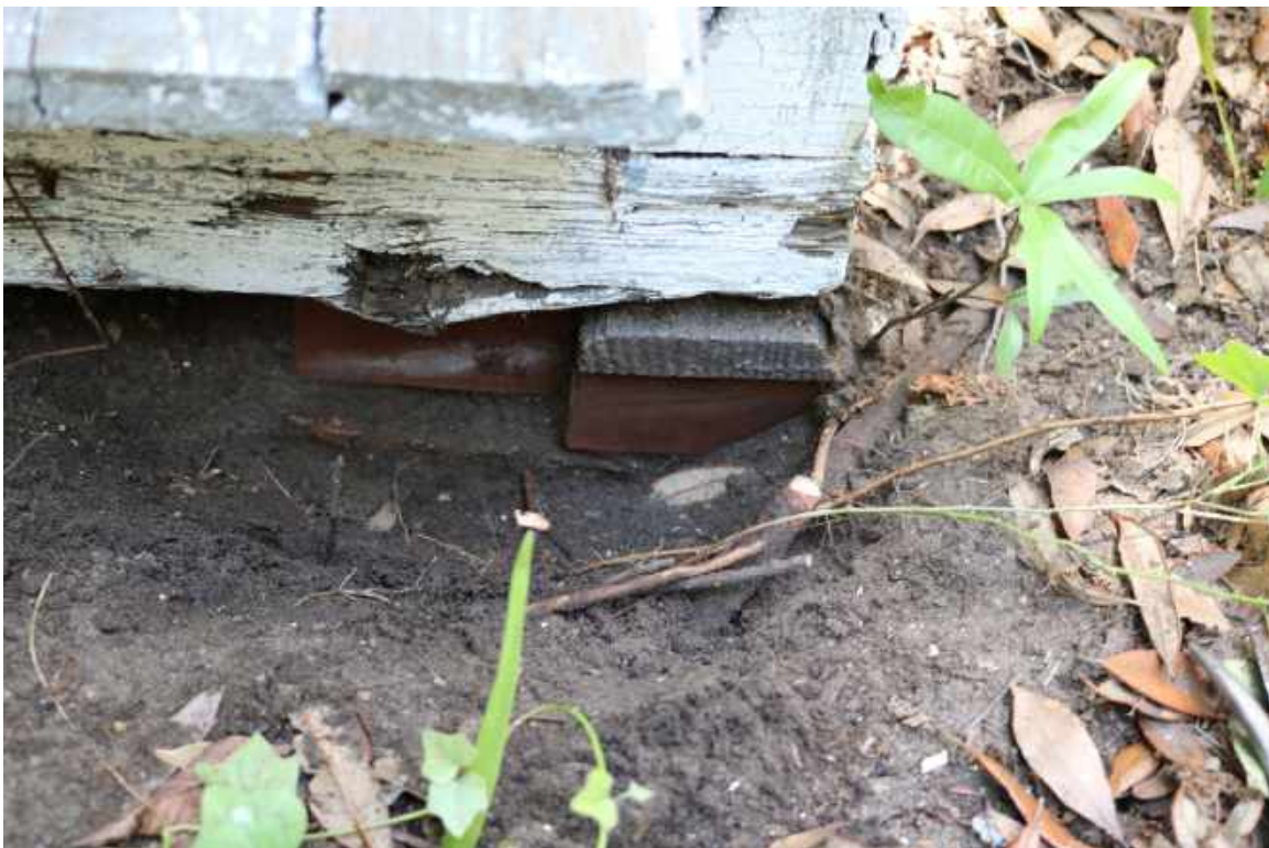
Figure 73: Southwest Corner of Porch: The porch foundation has also settled into the surrounding soil. The ends of the decking boards are deteriorated throughout the first-floor.
