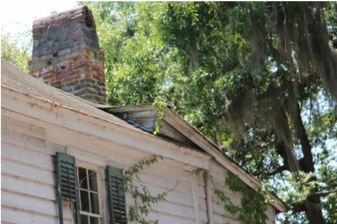
Figure 81: Northwest Corner of the Two-Story Building: Overview of the porch and infill roof detail where the roof intersects the original roof framing. This detail is also seen on the southeast corner of the building.
