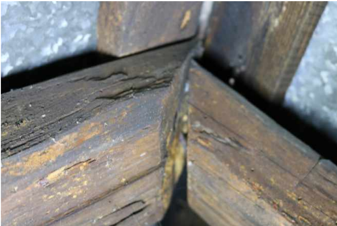
Figure 106: Attic of the One-Story Building, Rafters: Detail of toe-nailed rafters.
