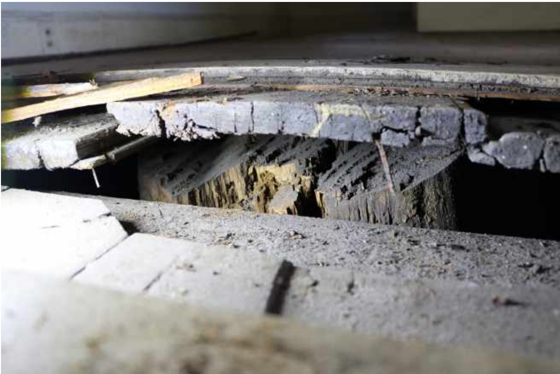
Figure 44: Room 101, Foundation: Detail of tree stump found between the floor joists when the flooring was selectively removed.
