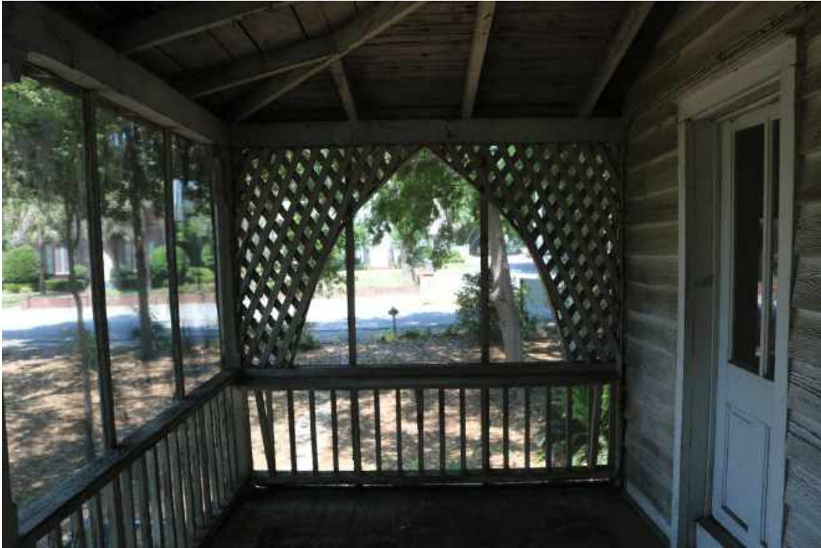
Figure 76: South Elevation, Second-Floor Porch: Detail of decorative lattice on the west end.
