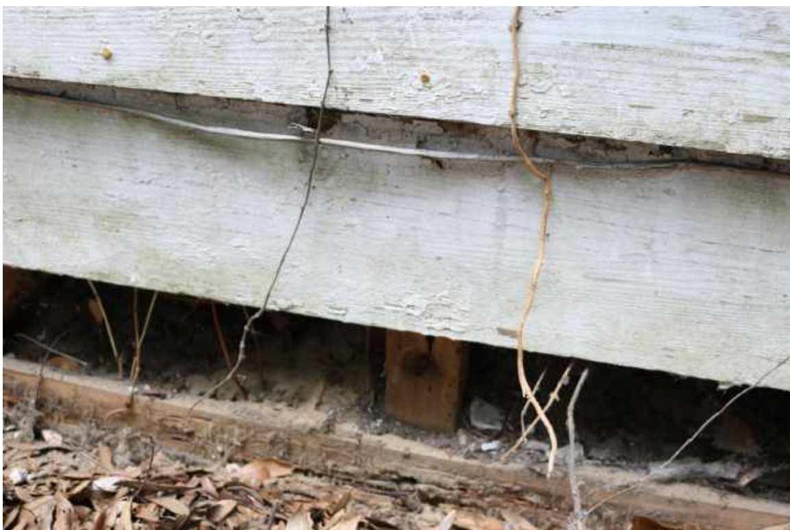
Figure 140: North Elevation: Detail of buried perimeter sill with a vertical framing member exposed.
