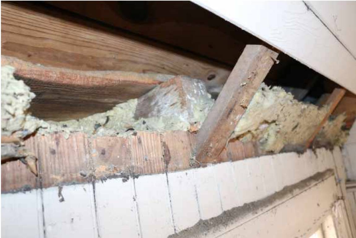
Figure 128: Second Floor, Room 204: Detail of the exposed framing members. The vertical wall paneling was installed up to the original whitewashed ceiling joists. The joists have been cut to accommodate the slope in the ceiling.
