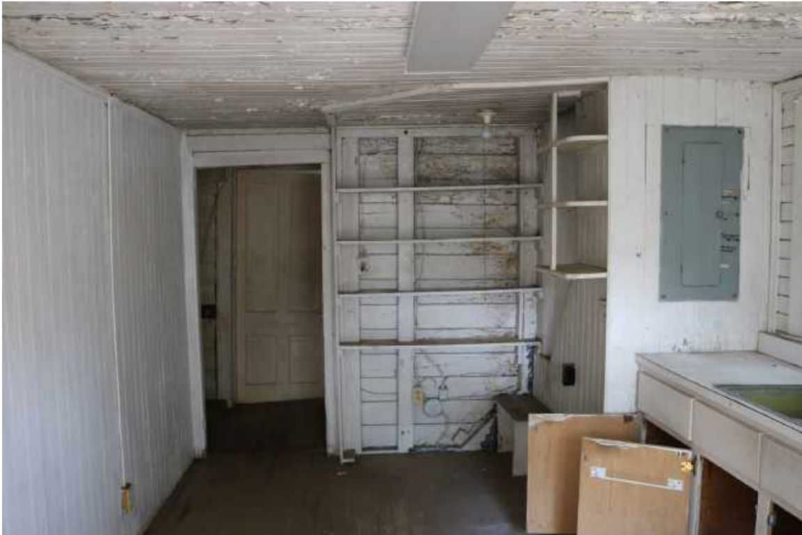
Figure 91: Room 105 (Kitchen), Looking West: Attic access is present at right. A variety of interior wall finishes are present throughout this space.
