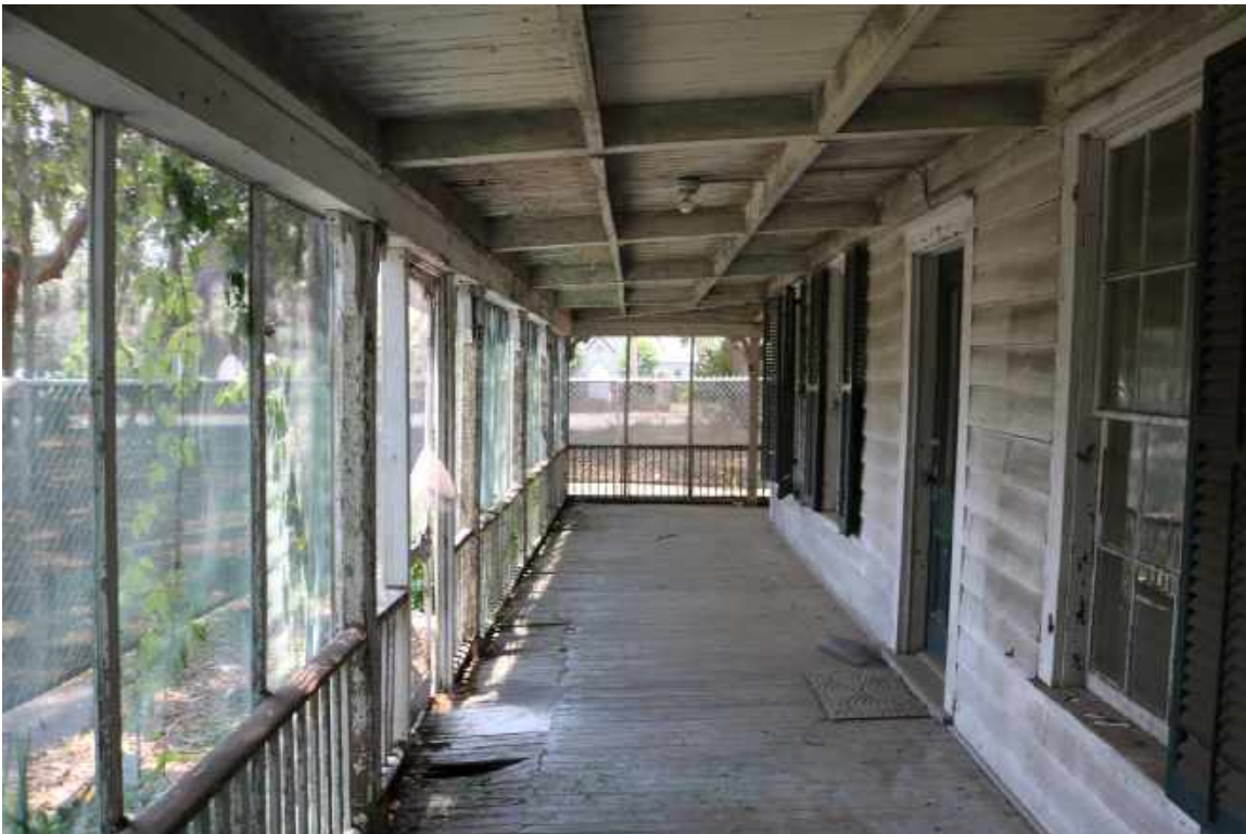
Figure 71: South Porch of the Two-Story Building: Overview of the first-floor porch looking west. The porch framing does not appear to date to the construction of the building.
