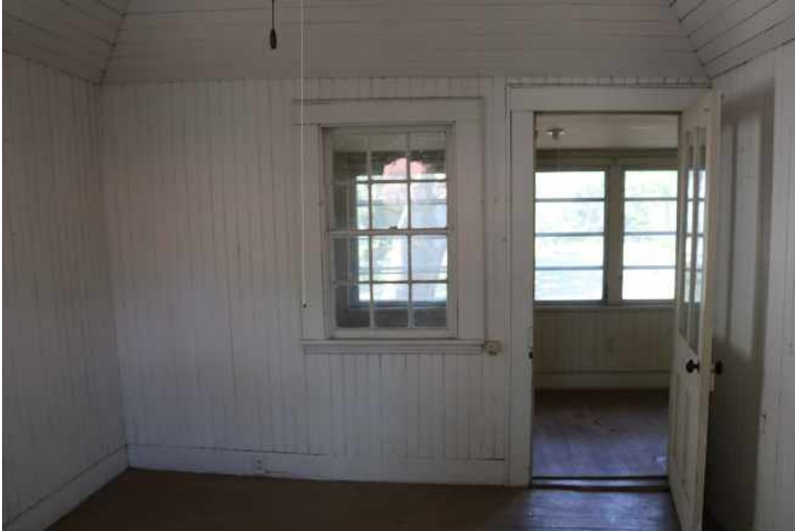
Figure 104: Room 205, South Elevation: Detail of the interior finishes within this room looking towards Room 206.
