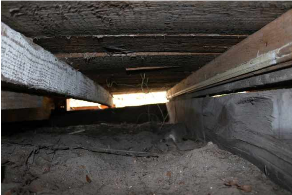
Figure 55: Crawlspace Below Room 103, Looking North: Detail of Floor Joists. The intermediate perimeter sill is located at right. An additional floor joist has been installed directly over the sill after the building was enlarged.
