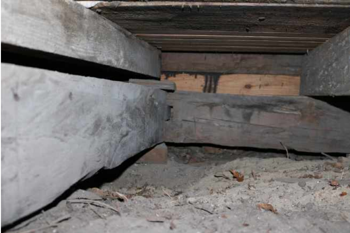
Figure 45: Crawlspace Beneath Room 103, Looking South: Detail of the intermediate eastern perimeter sill (at left) mortised into the south perimeter sill. The sill at left is believed to be the original eastern sill for the smaller structure. Note adze marks on both historic sills. An floor joist is installed above the intermediate perimeter sill.
