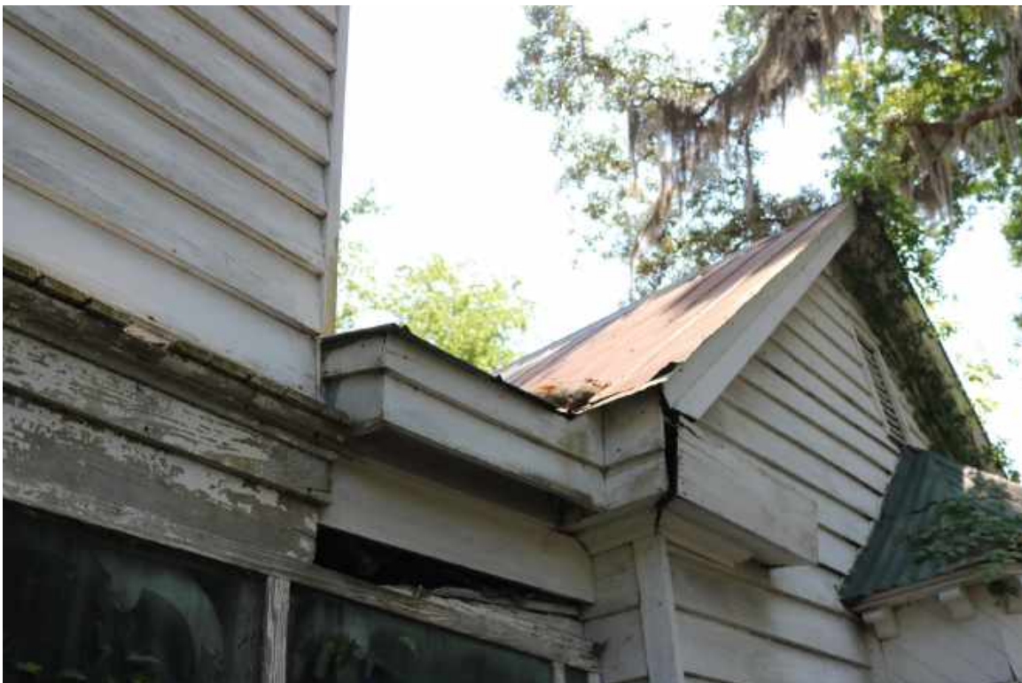
Figure 70: South Elevation of Hyphen: Detail of dislodged fascia trim on the gable eyebrows.
