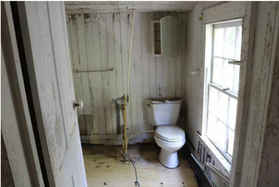
Figure 95: Room 201, Looking West: The room has been infilled on the roof of the first floor porch. Due to settlement in the foundation, this room is structurally unstable.
