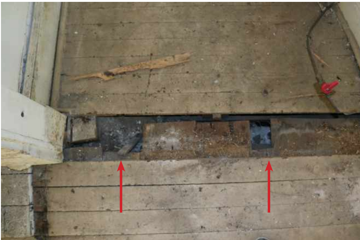
Figure 120: First Floor, Room 101 Northwest Corner: Detail of the underlying floor following removal of the thinner boards. Square cuts in the underlying floor are the locations of the vertical studs for the original west wall.
