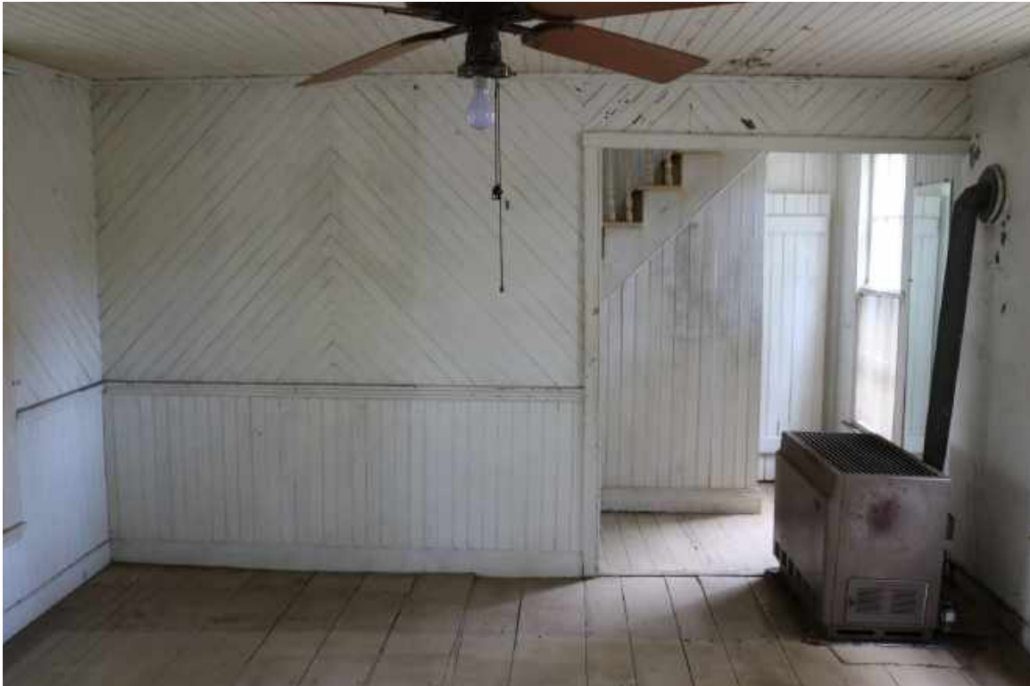
Figure 88: Room 103, Looking West towards the Stair-Hall. The opening between the rooms has been enlarged towards the north.
