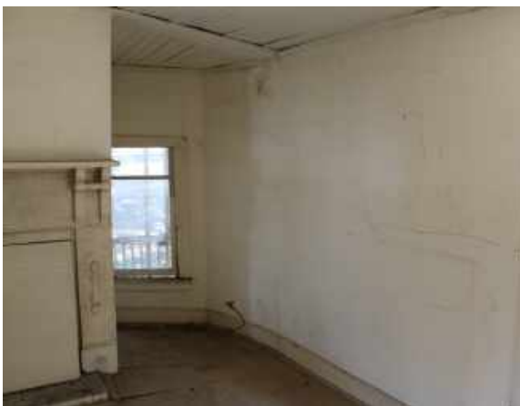
Figure 151: North wall within Room 101.
