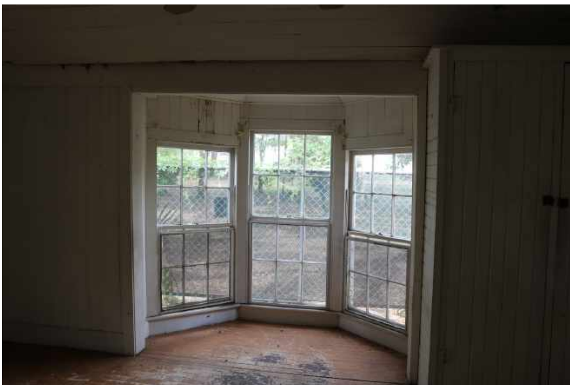
Figure 94: Room 107, Looking South: Detail of interior of the bay window. Note the separation of the floor below the windows.
