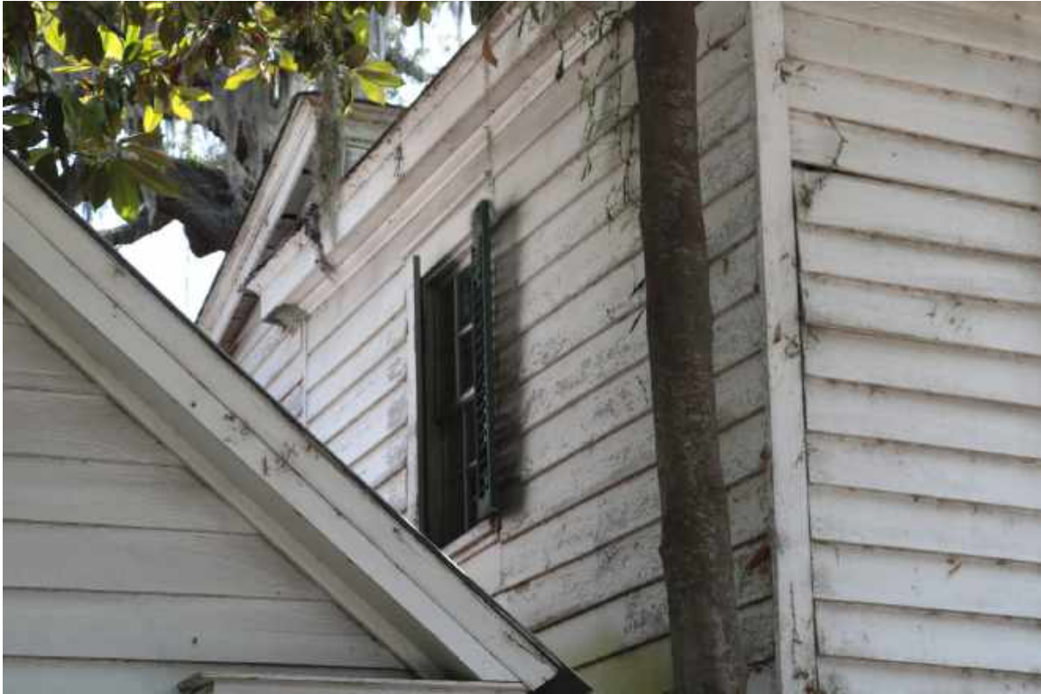
Figure 82: East Elevation of the Two-Story Building: Detail of the porch roof detail where it intersects the main roof at the southeast corner.
