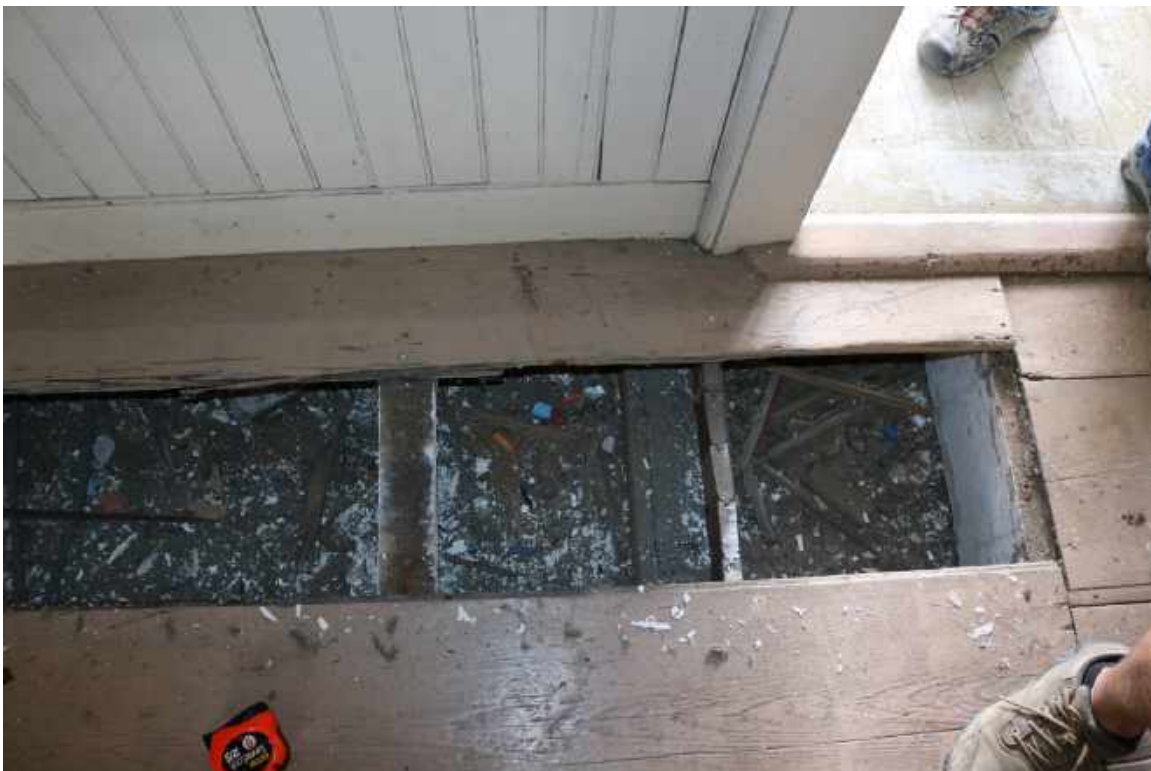
Figure 123: Second Floor, Room 204: Detail of framing conditions. A whitewash covers the exposed faces of the joists.
