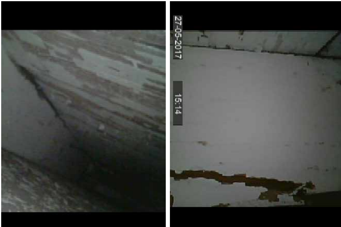
Figure 58: Second Floor Joists Below Room 202: One joist was cracked due to settlement. The joists are hidden due to ceiling paneling in Room 101. The floor joists are whitewashed, indicating they were likely exposed on the first-floor.
