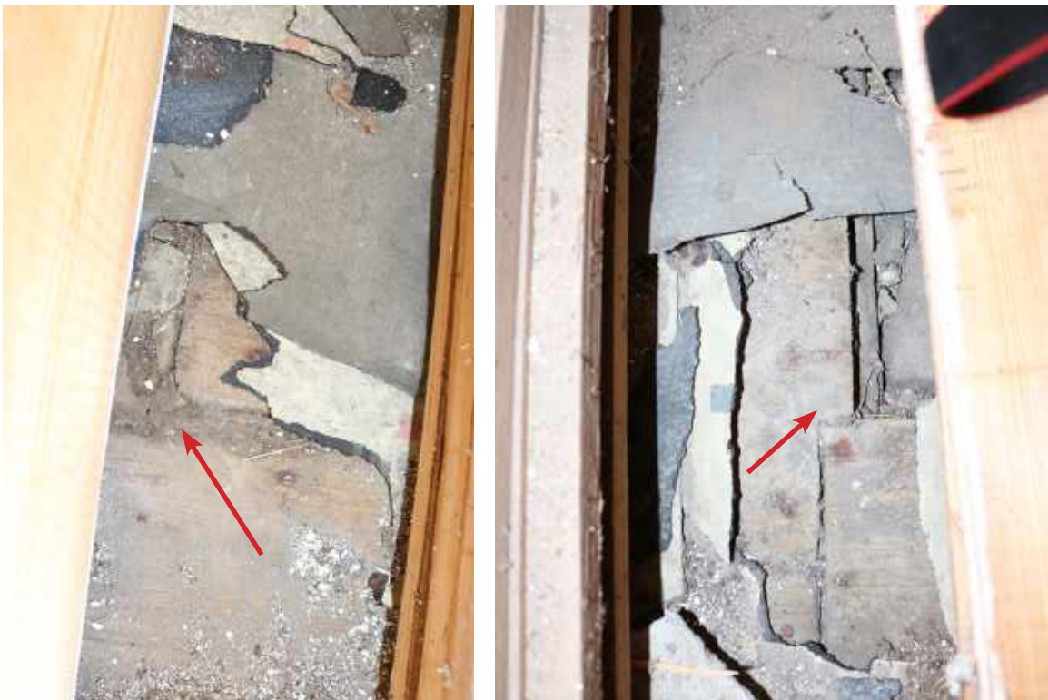
Figure 134: Detail of hearth floor detail at Friendfield Plantation (arrows). This detail is less decorative than that visible at Squire Pope.
