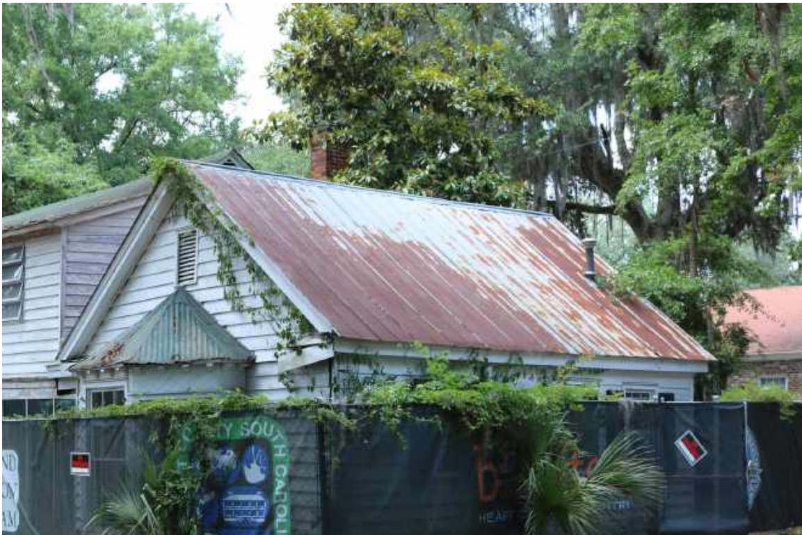
Figure 83: One-Story Building Roof: The roof is a modern 5V steel roof. This roof was likely installed in the 1990s. The coating has failed and the metal roofing panels are actively corroding.
