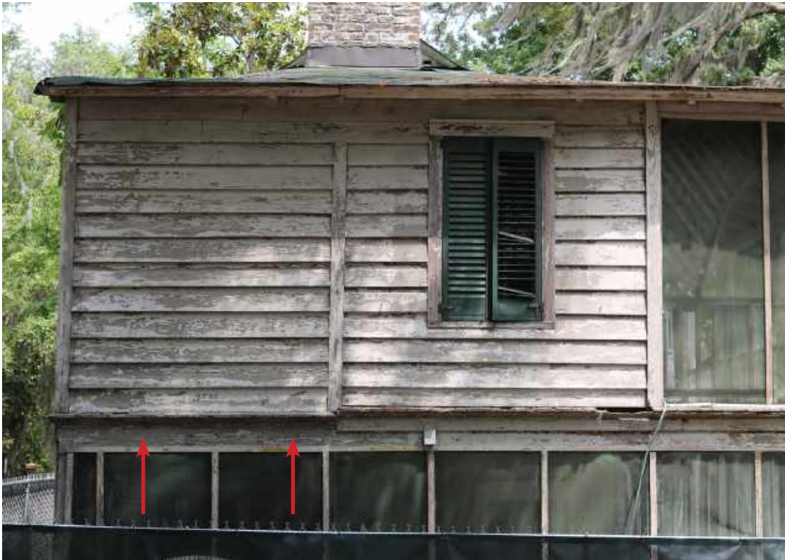
Figure 182: Detail of wood shake roof below the second floor bathroom infill (arrows). The corner siding boards also remain in place. The enlargement at right is later.
