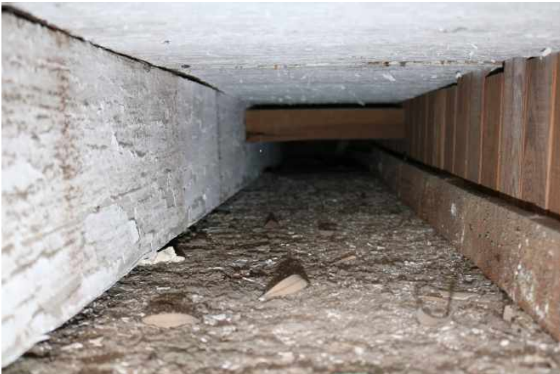
Figure 126: Second Floor, Room 204: Detail of the intersection between the first floor stair wall (at right) with the historic whitewashed framing material. The ceiling paneling of Room 103 is at bottom.
