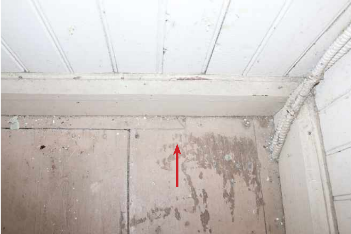
Figure 102: Room 204: Detail of matching floor detail found in Room 202 (arrow). All four corners of the second floor opening were identified, indicating there was likely a central opening in the structure.
