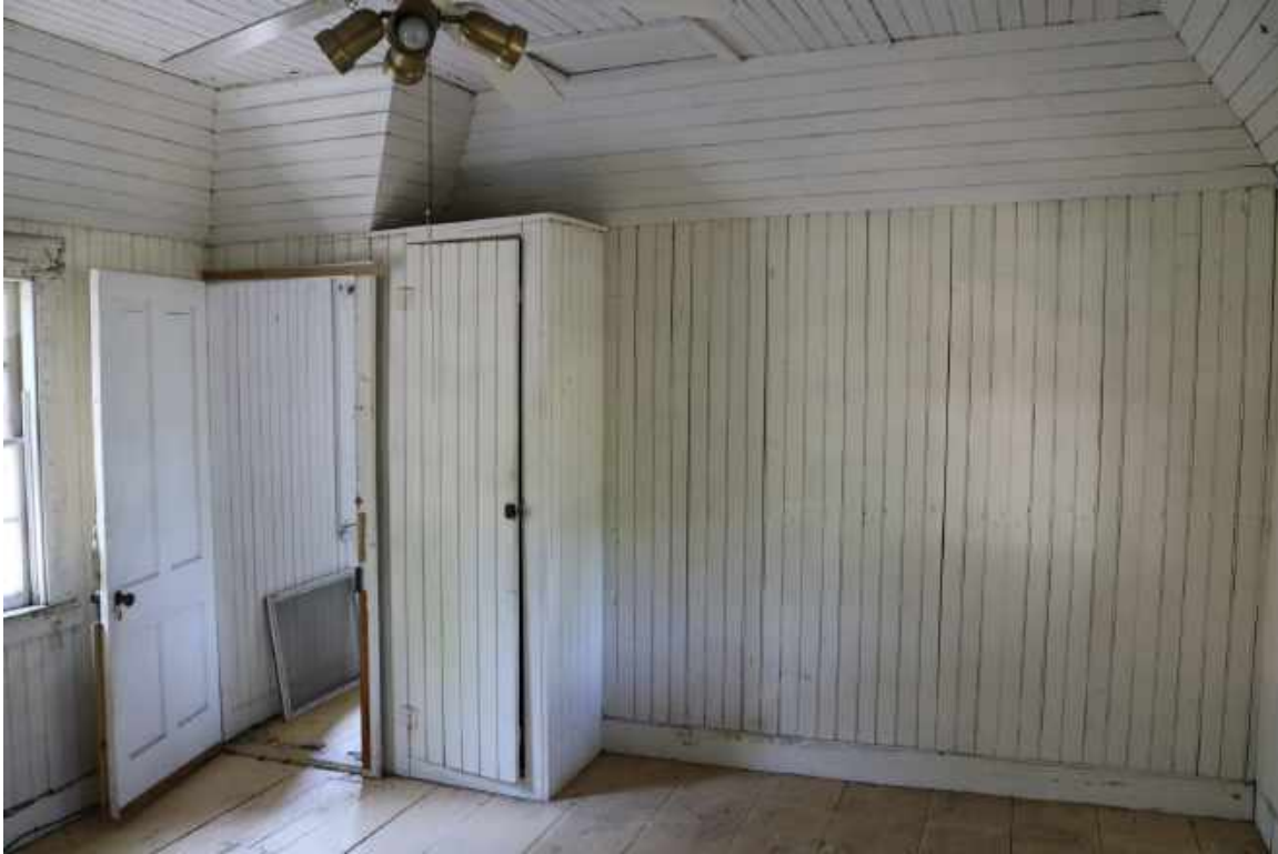
Figure 97: Room 202, Looking Northeast: Many of the rooms on the second floor feature a canted ceiling with beadboard installed at an angle. Note the differences in profile and size between the vertical and angled ceiling paneling.
