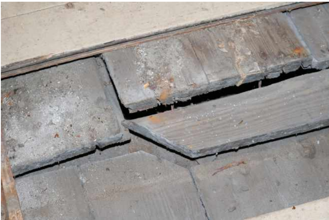
Figure 117: First Floor, Room 101: A similar flooring detail to that found in Rooms 202 and 204 was found at this location. This may indicate that the center of the original structure once contained a large two-story opening.
