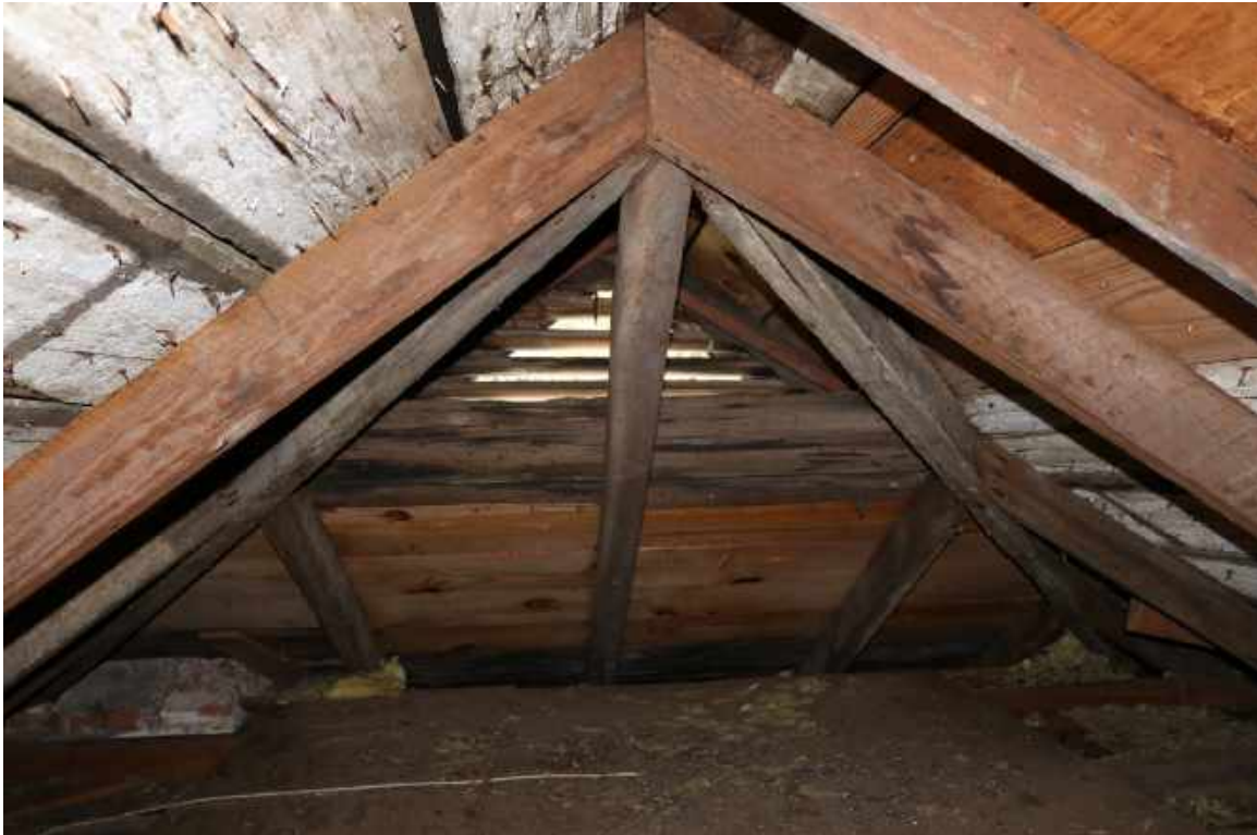
Figure 111: Attic of Two-Story Building, Eastern End: Detail of roof framing at gable vent. Note the absence of pegs at the rafter ridge.
