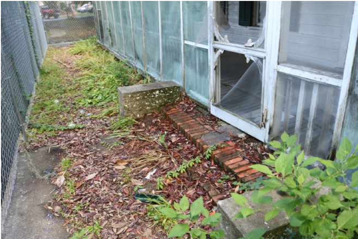
Figure 72: South Elevation of the Two-Story Building: Overview of the first-floor porch entrance concrete tabby and masonry steps.
