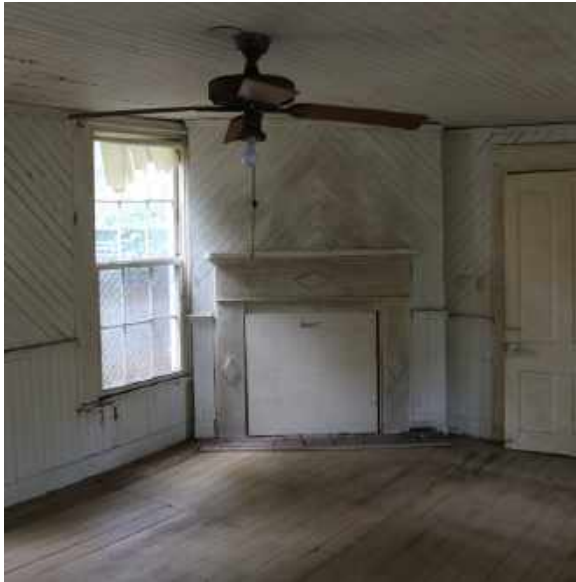
Figure 158: Photograph of Room 103. The fireplace mantel in the northeast corner of Room 103 was sampled to determine whether the diamond at the center of the apron was installed originally with the mantel or applied at a later date.
