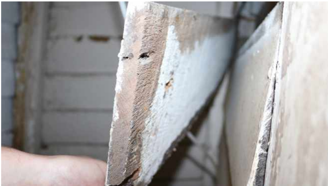
Figure 181: Hyphen, East Elevation of Two Story Building: Detail of whitewash on the backside of dislodged siding indicating the east enlargement of the two-story building was also whitewashed.
