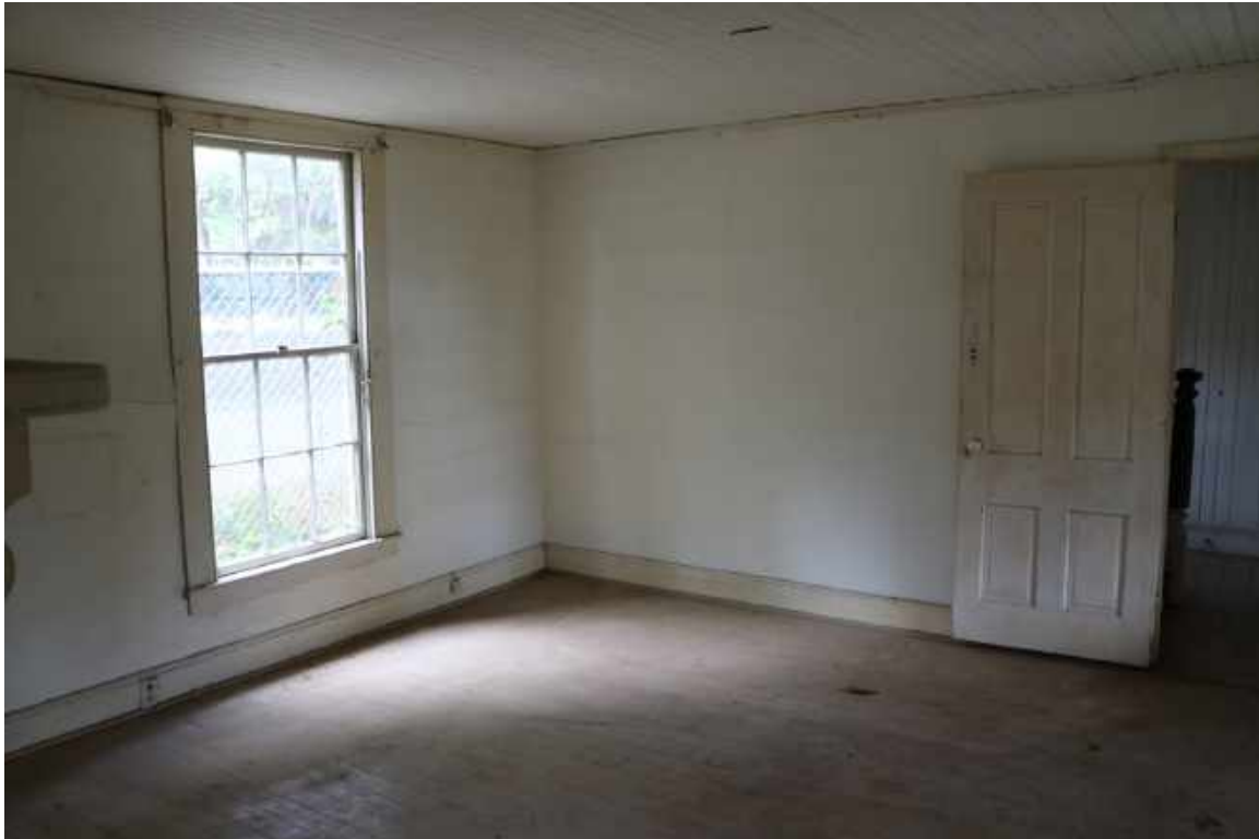
Figure 86: Room 101, Northeast Corner: Detail of interior conditions and the interior door.
