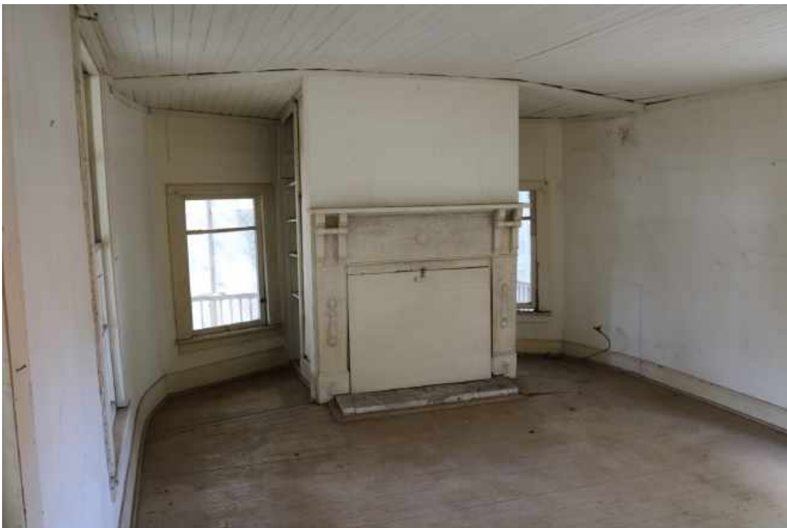
Figure 85: Room 101, Looking West: There is extensive settlement on either side of the masonry chimney. The ceiling visible bows downward on either side.
