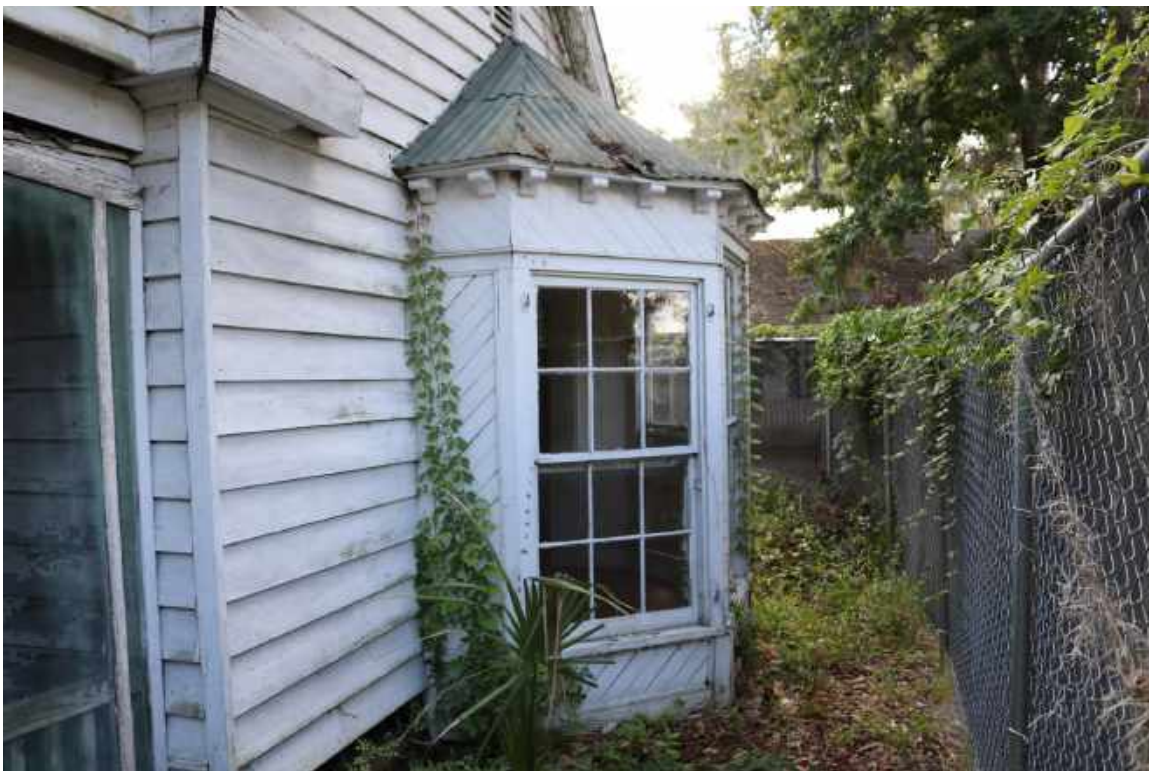
Figure 63: South Elevation, One-Story Building: Detail of bay window. The older corrugated roof visible on the historic photographs remains on the bay window.
