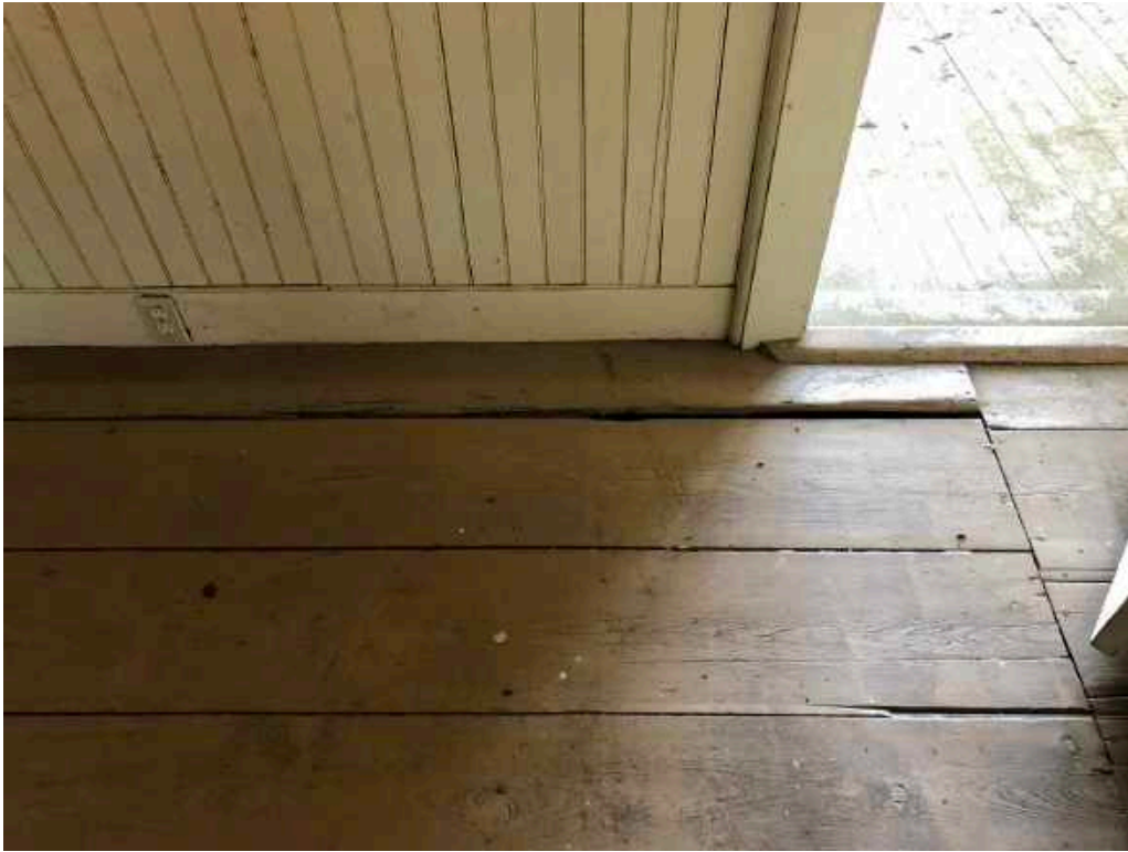
Figure 122: Second Floor, Room 204: Location of floor boards removed to investigate the second floor framing.
