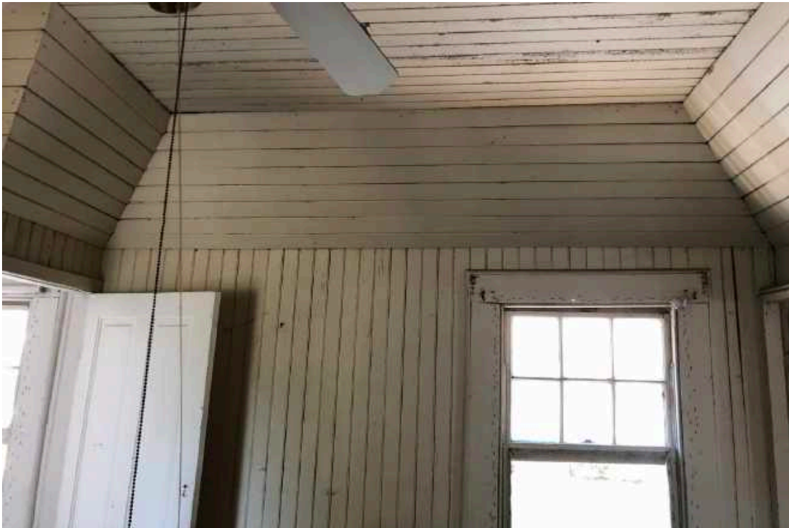
Figure 127: Second Floor, Room 204: The cant ceiling was removed along the north wall within this room.
