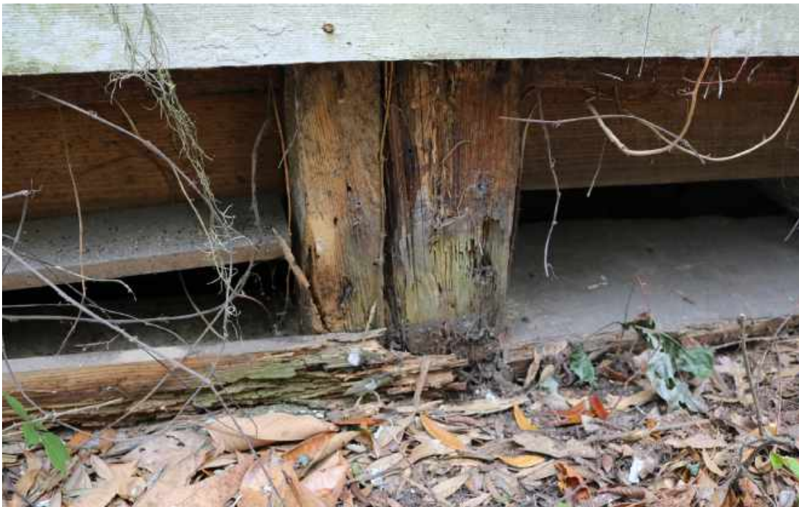
Figure 46: North Elevation of Two-Story Section: Detail of Eastern “Corner Post” with an additional stud added to the east (at left). The right vertical member appears to be the original corner post for the smaller structure prior to enlargement.
