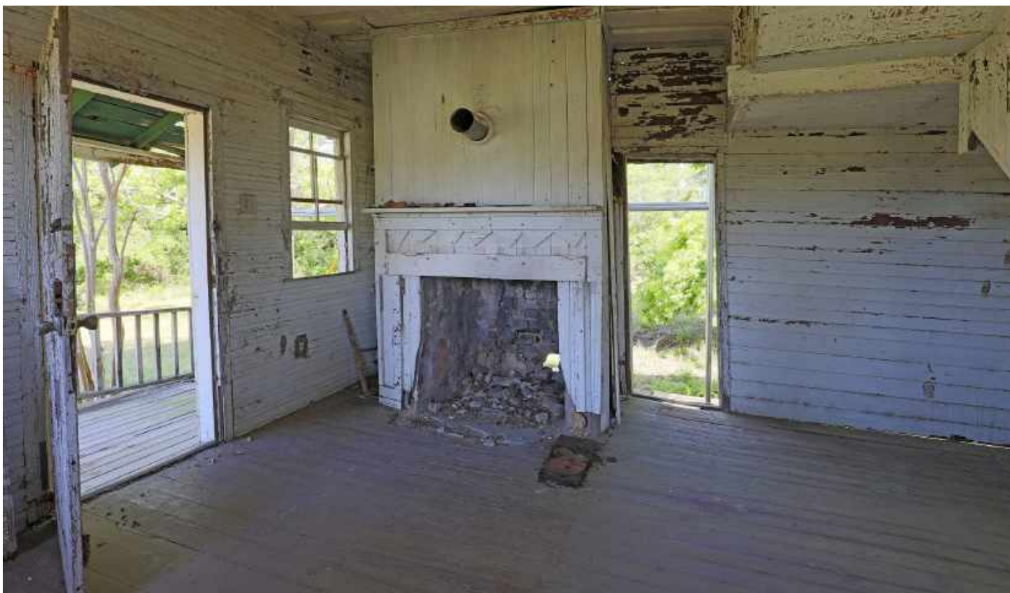
WEST ROOM - FIRST FLOOR
