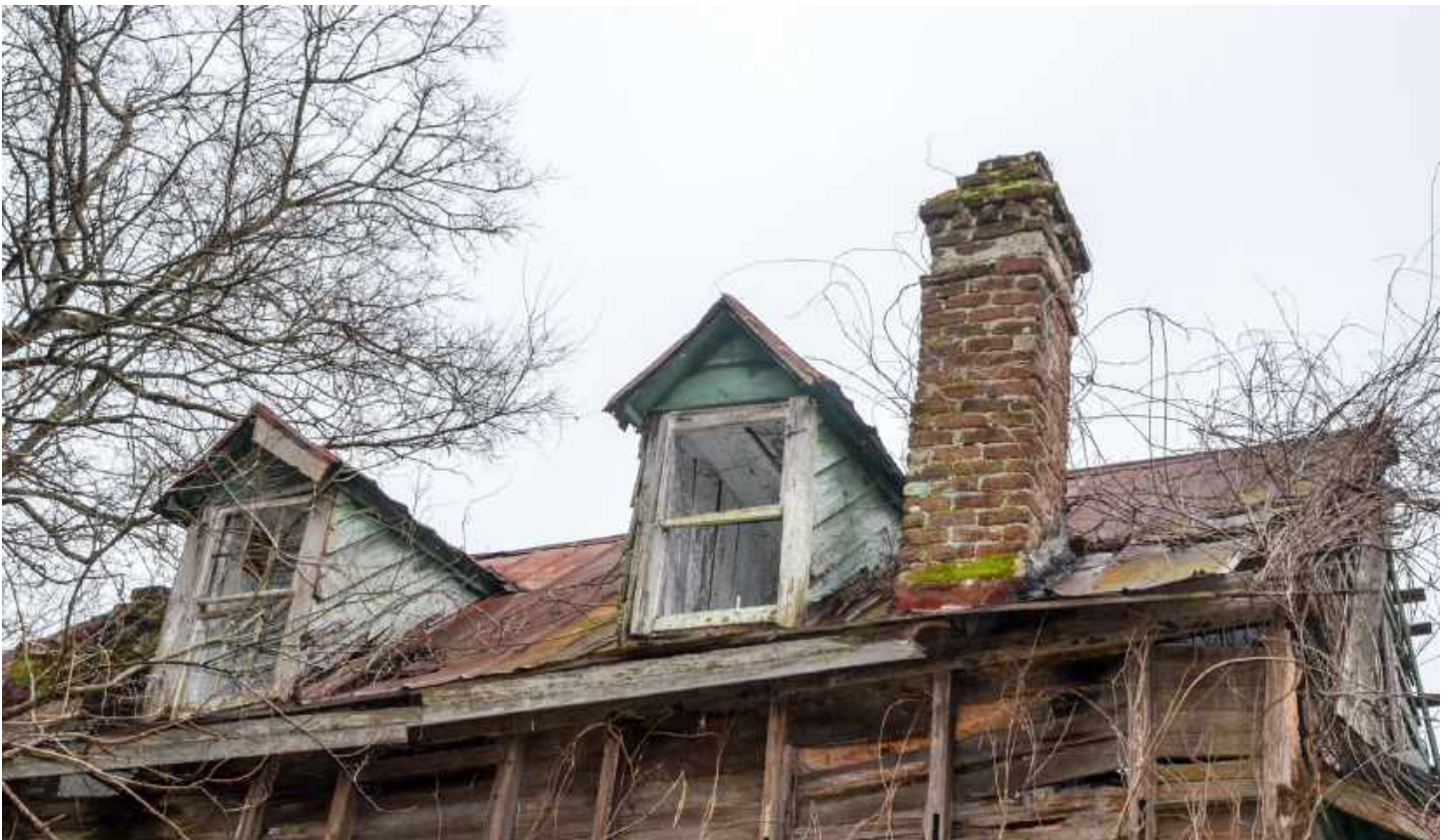
NORTH DORMERS AND CHIMNEY
