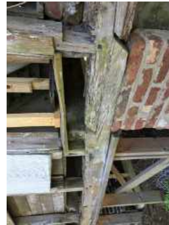
28 North wall of piers at splice with door openings above
