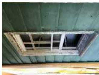
15 Window at west porch
