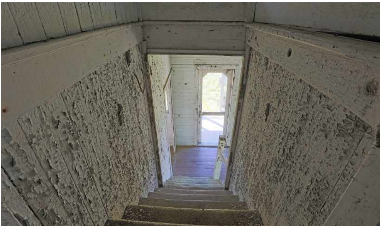
STAIR AND FRONT ENTRY DOOR TO PORCH
