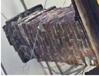
24 North wall of chimney
