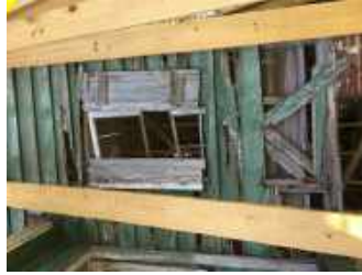
19 Window east of south porch
