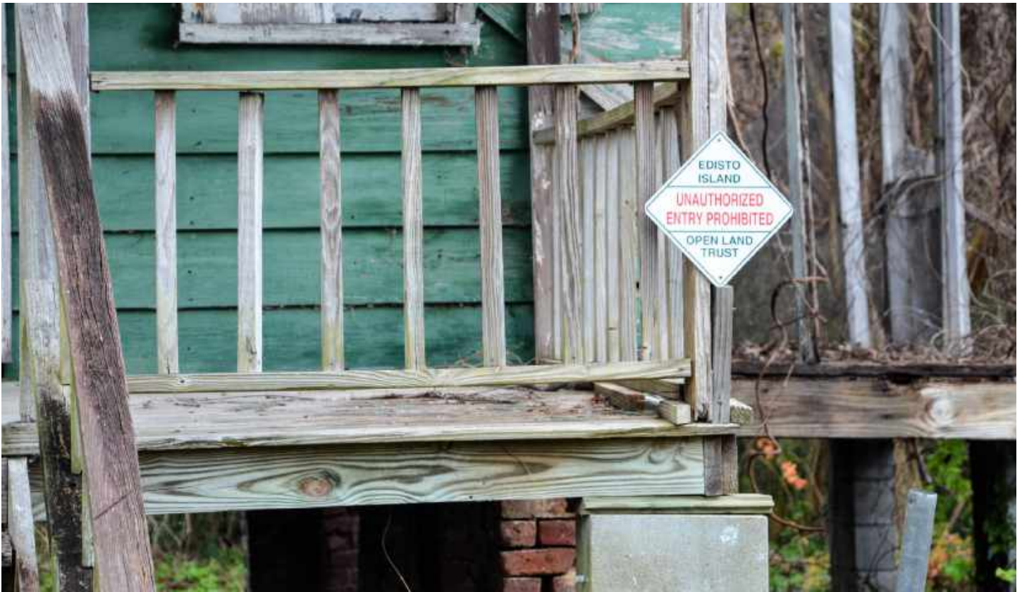
WEST PORCH RAIL, PIER, FRAMING
