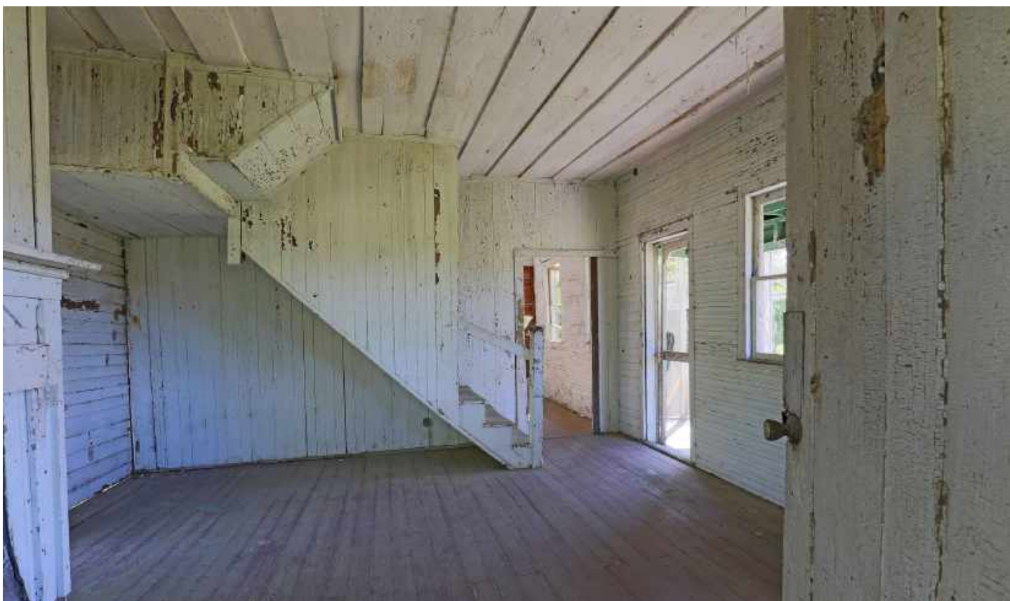
WEST ROOM - FIRST FLOOR
