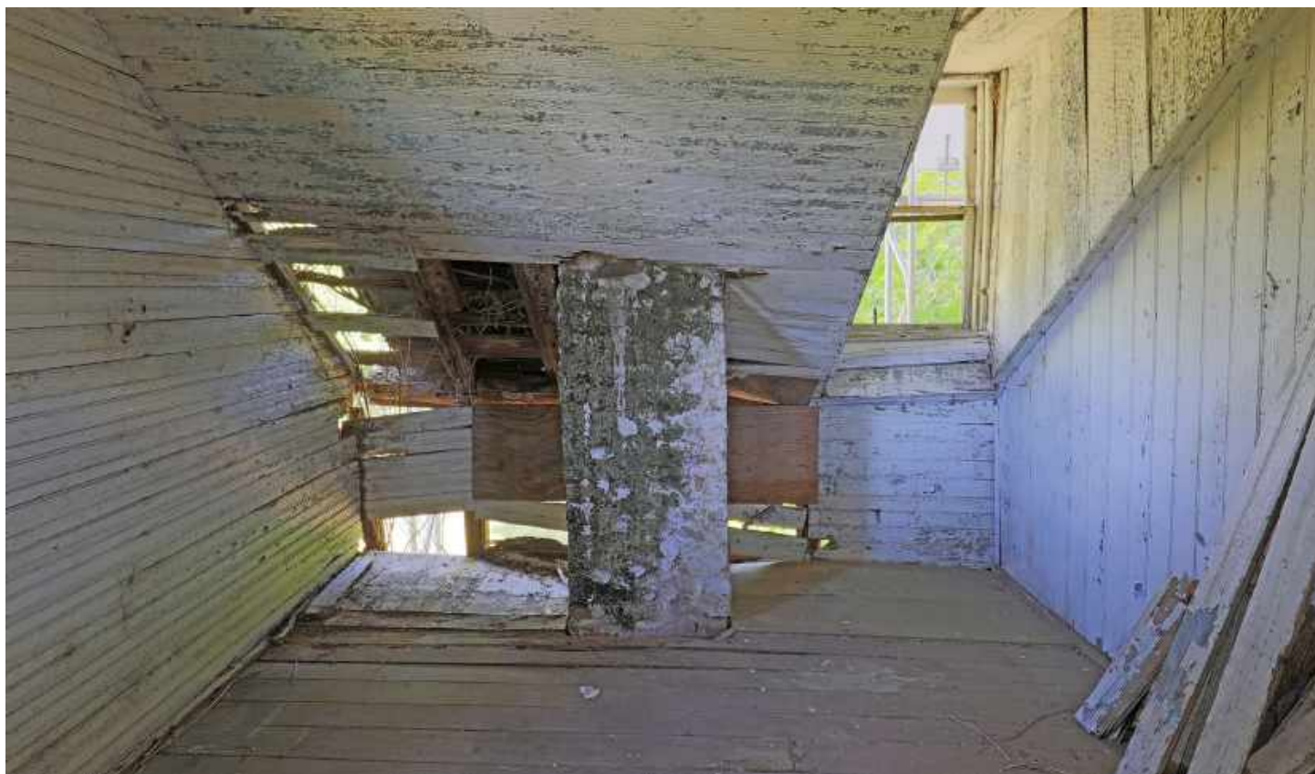
WEST ROOM - SECOND FLOOR
