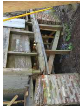
27 North wall of piers with door openings above brick piers
