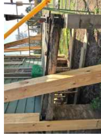
26 North wall of piers continues along west porch
