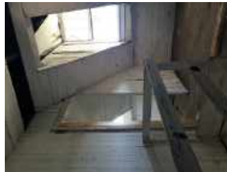
37 Second floor - star looking southeast
