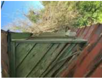
13 East wall of south end corner
