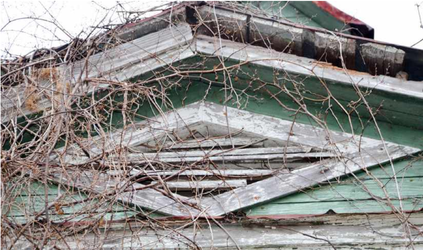
VENT AT FRONT PORCH
