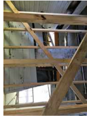
41 Second floor - west room looking north
