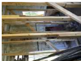
35 First floor - west room fireplace
