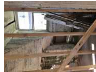
40 Second floor - west room looking north
