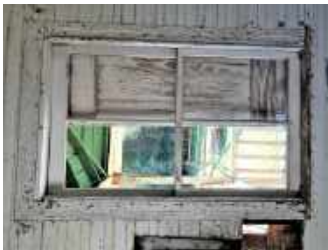
30 First floor window detail
