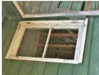
17 Window at south porch
