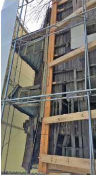
23 North elevation showing chimneys, chimneys are on raised joists at side wall
