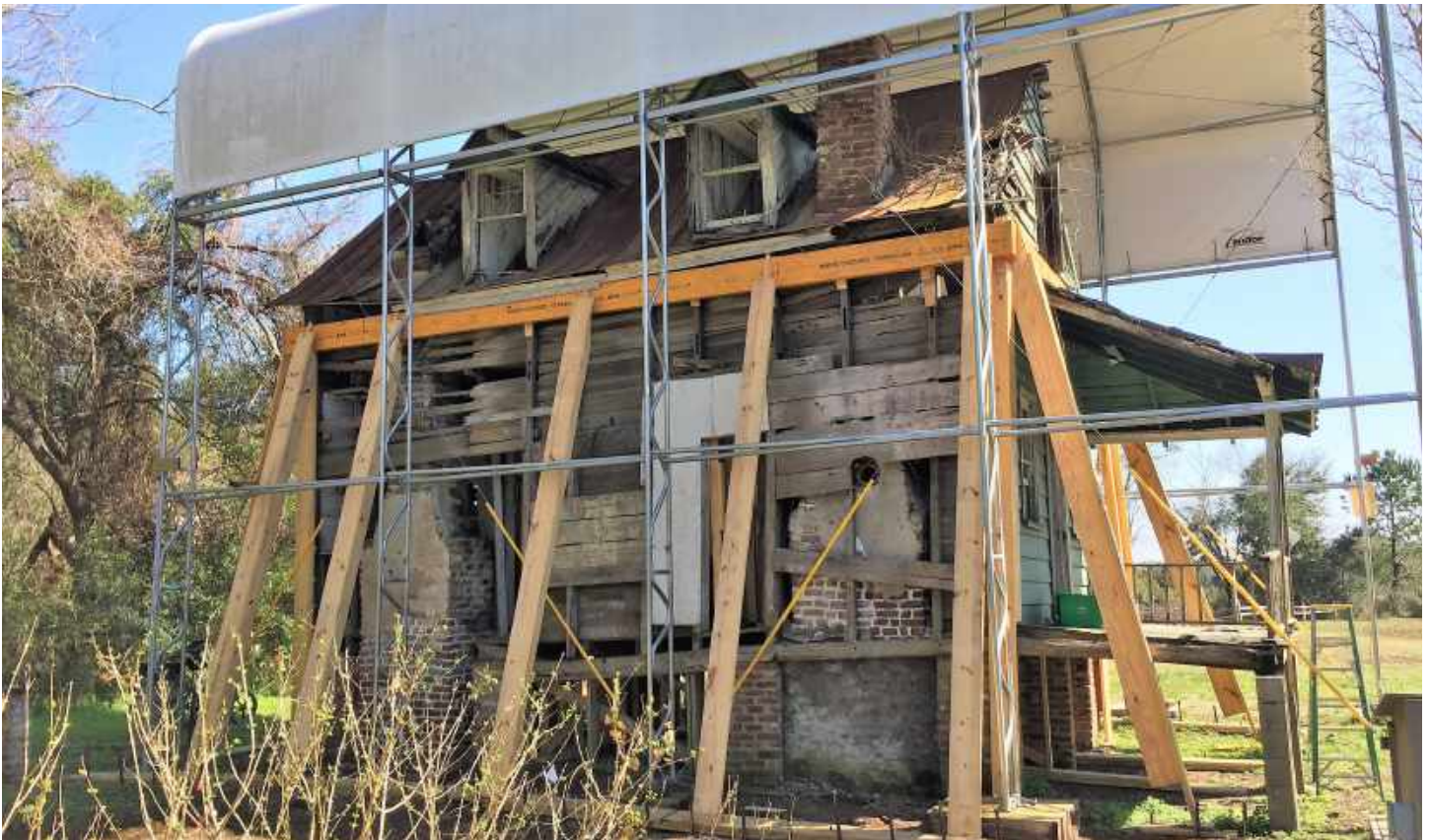
EXPOSED FRAMING FROM NORTHWEST
