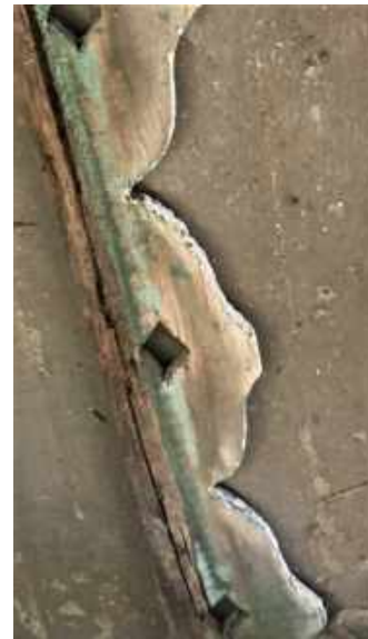
21 Detail of new trim photo taken with trim on roof
