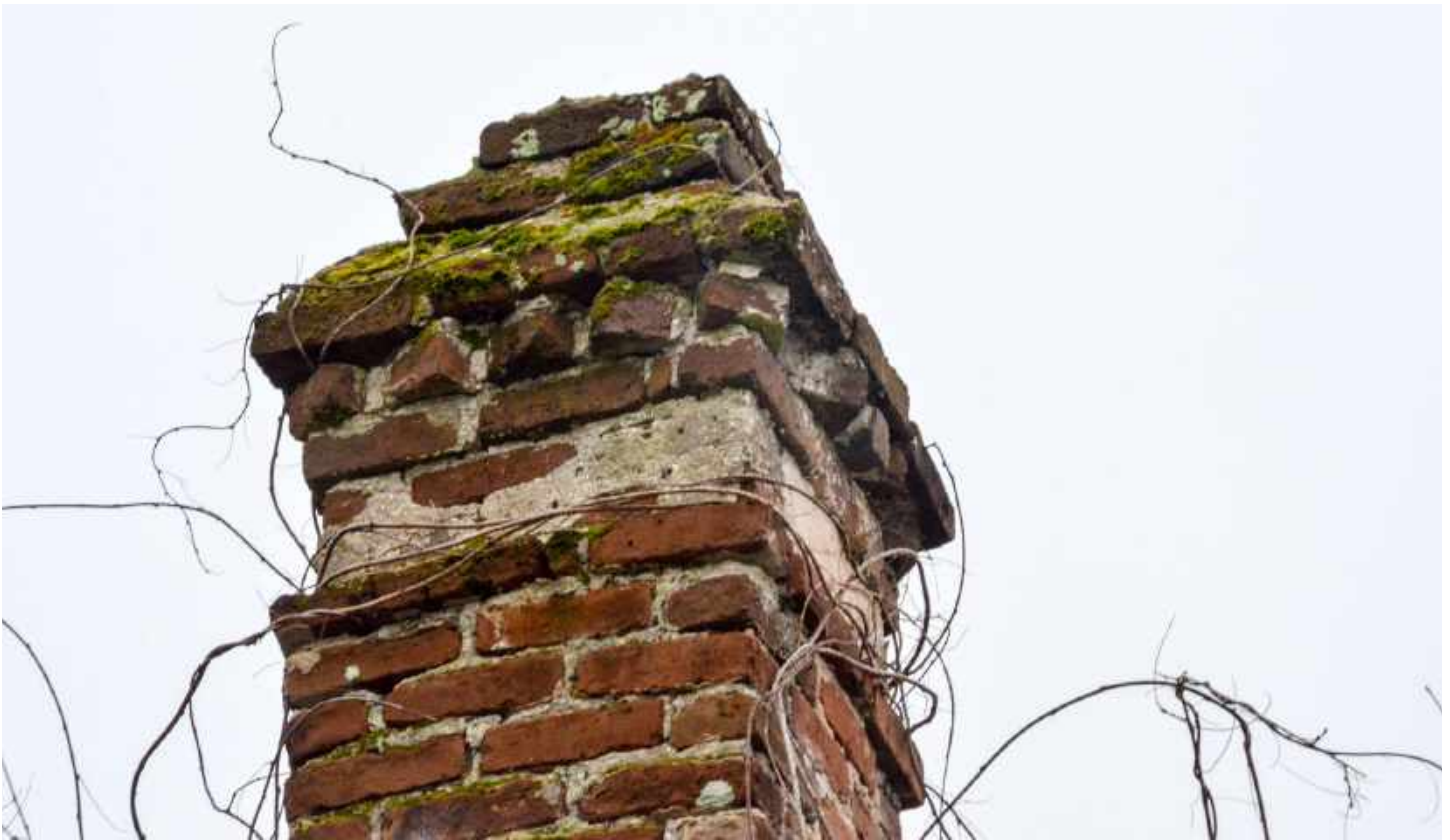
WESTERN VIEW OF CHIMNEY
