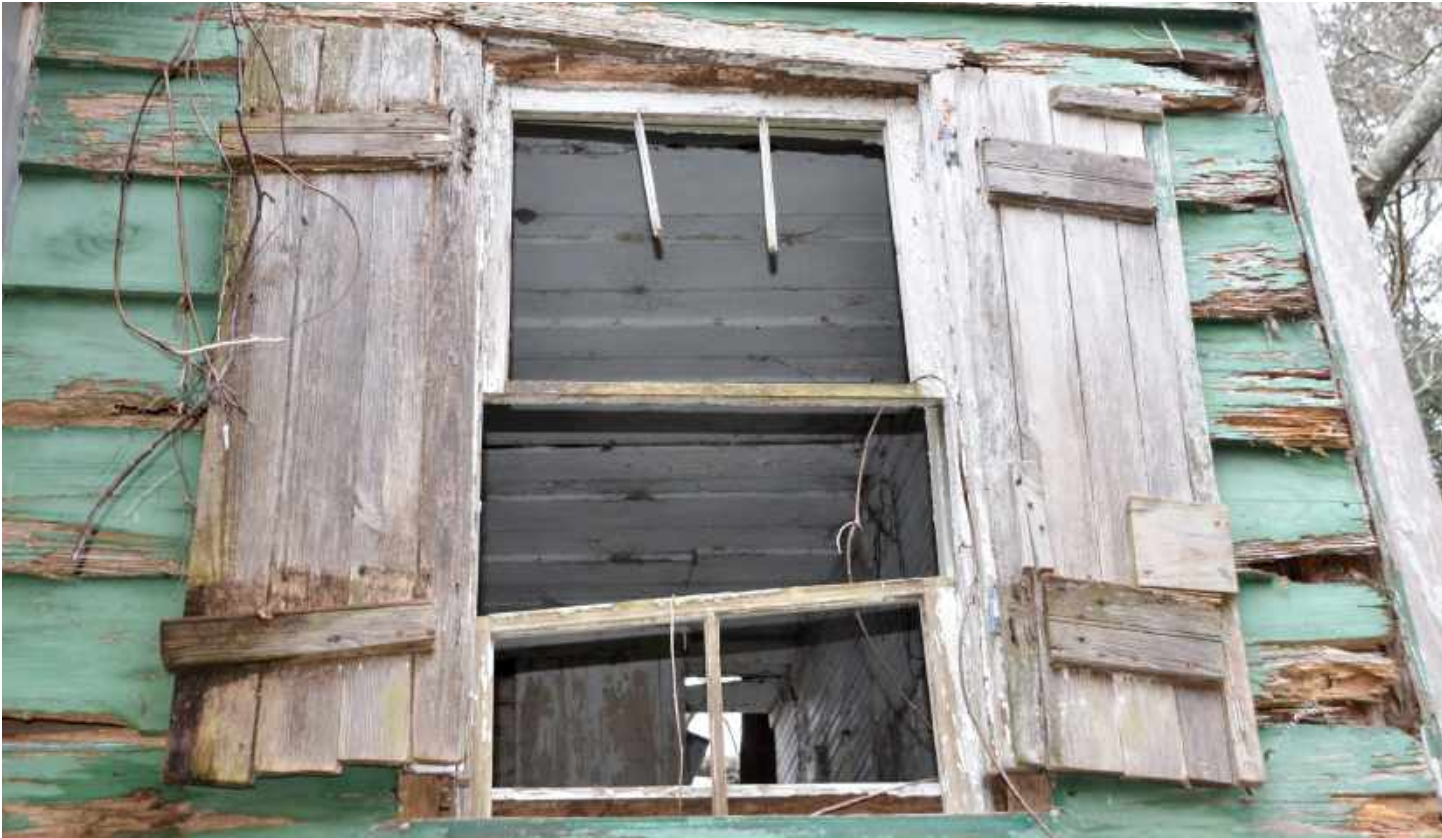
SHUTTERS AT WINDOW FRAME
