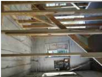
31 First floor - west room looking southwest
