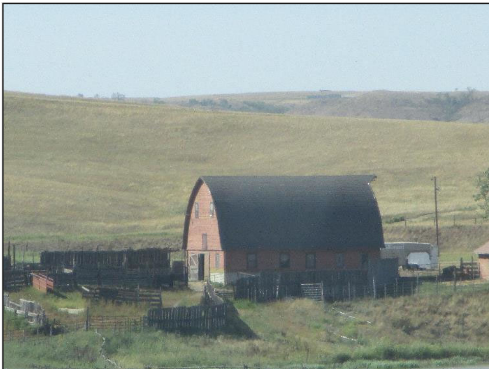
HK00400001 – Alleman Station – Gambrel Barn (Kirley Vicinity)
