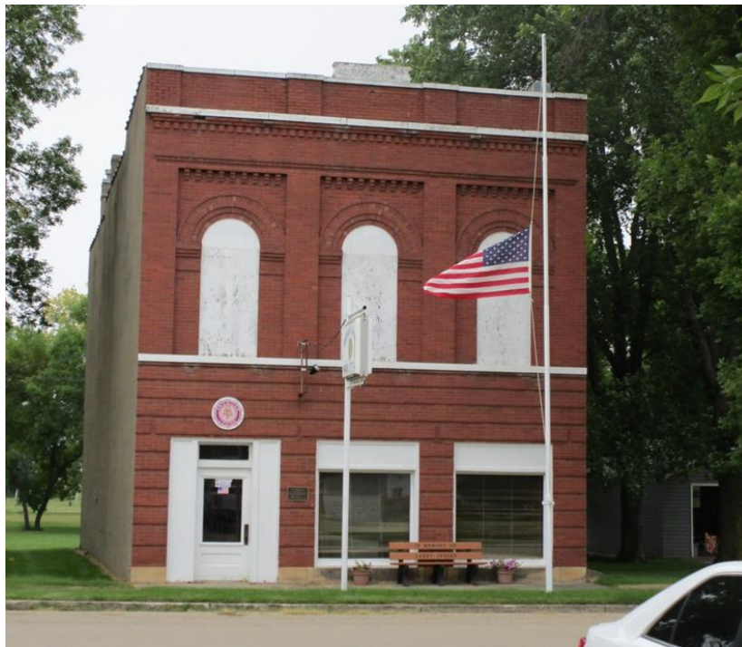
SD_Hamlin County_Byrant Masonic Temple_0001: View of south (main) façade, camera facing north.
