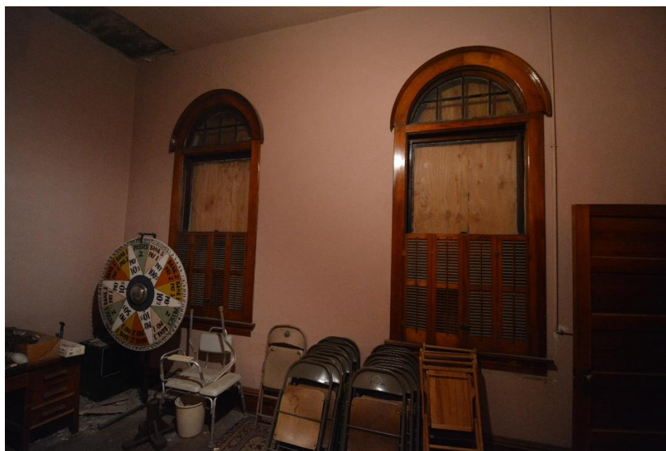
SD_Hamlin County_ Byrant Masonic Temple_0014: View of historic windows on second floor. Camera facing southeast.
