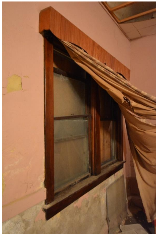
SD_Hamlin County_ Byrant Masonic Temple_0017: View of original window in the hall. Camera facing northeast.
