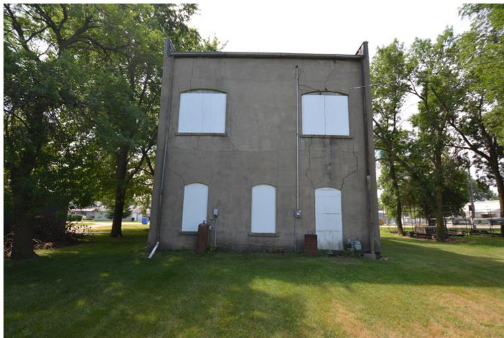
SD_Hamlin County_ Byrant Masonic Temple_0003: View of north (rear) façade, camera facing south.
