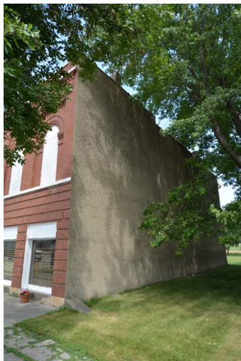
SD_Hamlin County_Byrant Masonic Temple_0002: View of east façade, camera looking northwest
