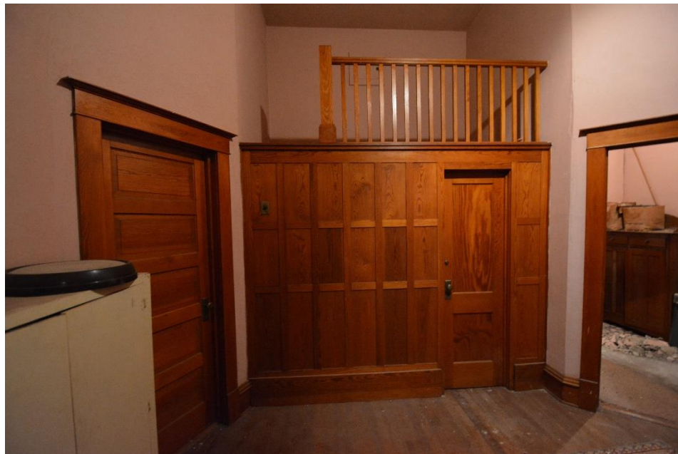
SD_Hamlin County_ Byrant Masonic Temple_0013: view of stage on second floor. Camera facing north.
