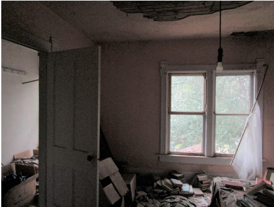
SD_Day County_Anderson House_0023: View of bedroom, camera facing southwest,
