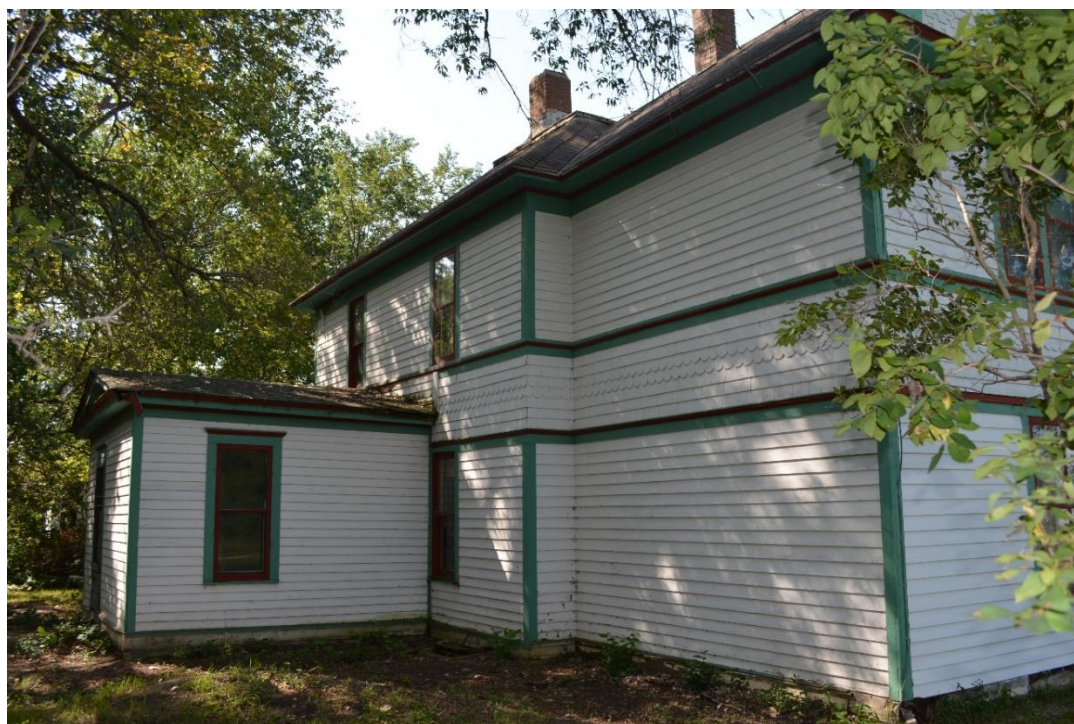
SD_Day County_Anderson House_0008: View of east façade, camera facing southwest.
