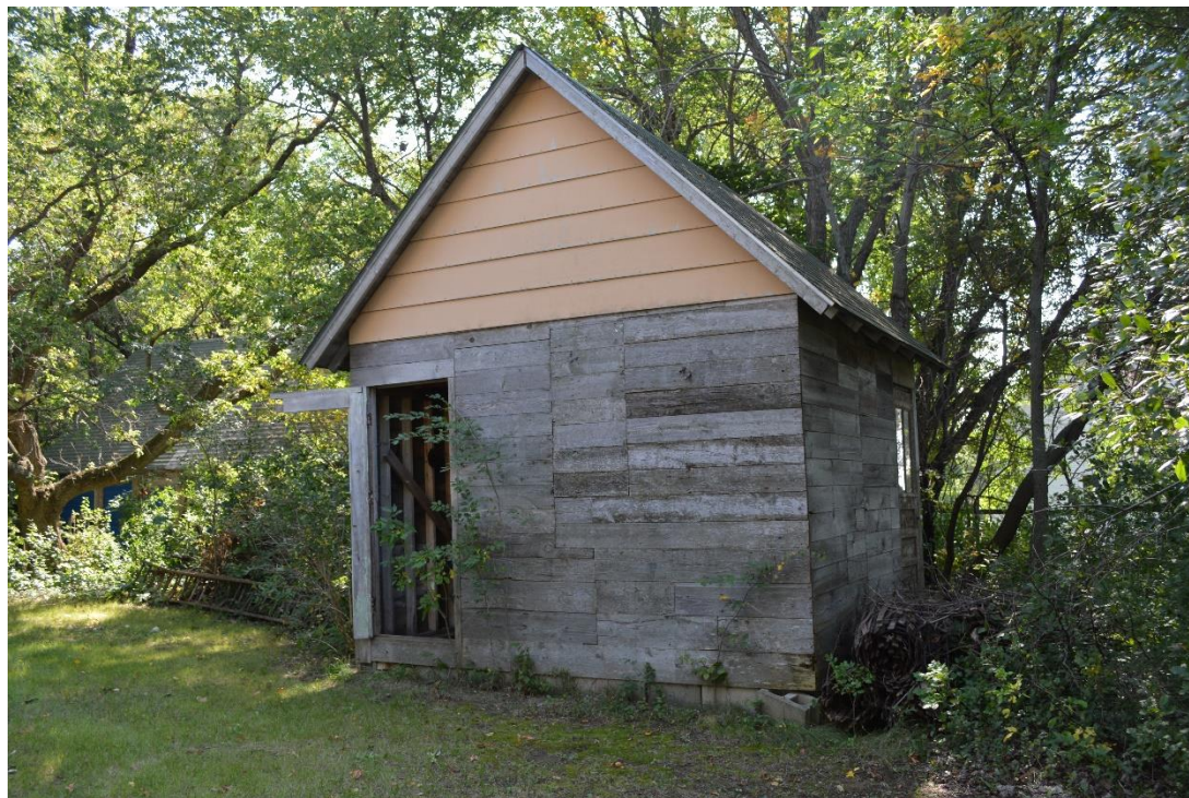
SD_Day County_Anderson House_0005: View of shed, camera facing southeast.
