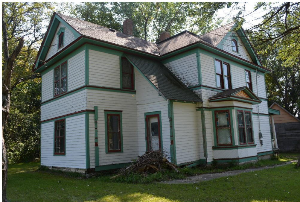
SD_Day County_Anderson House_0003: View of northwestern corner, camera facing southeast.
