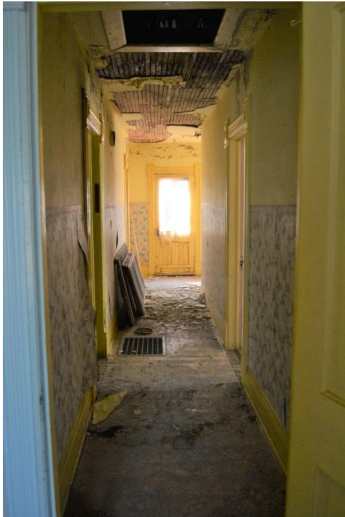
SD_Day County_Anderson House_0025: View of second floor hallway, camera facing north.
