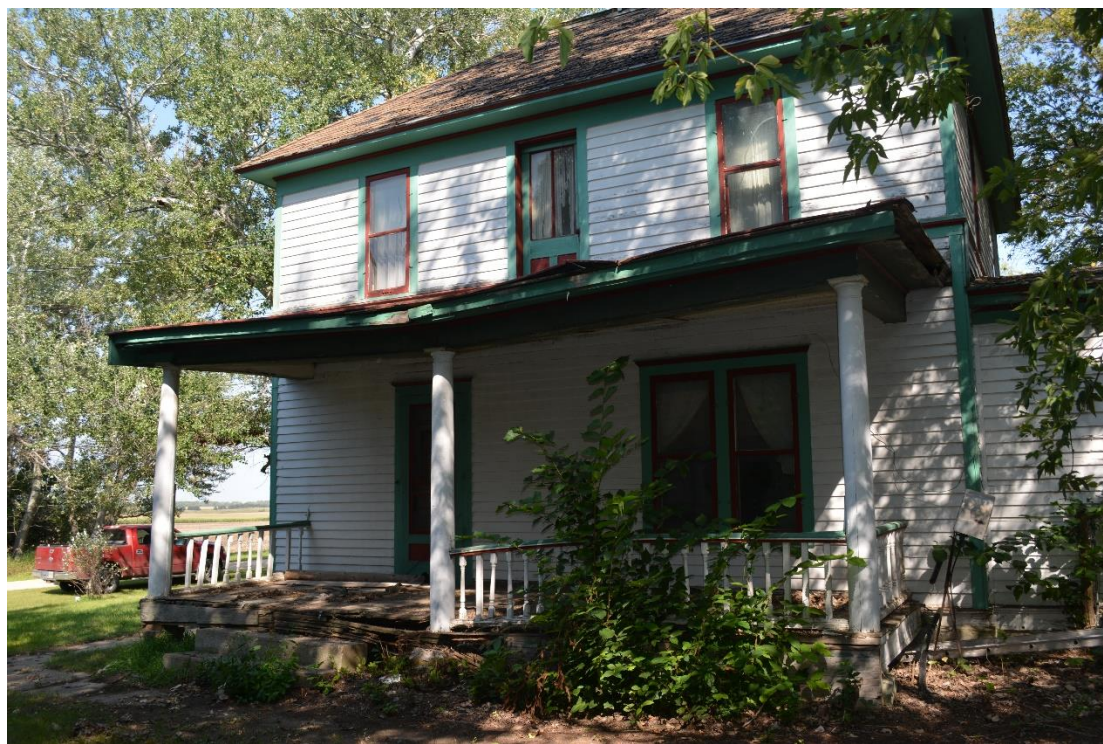
SD_Day County_Anderson House_0006: View of south façade and portico, camera facing northwest.
