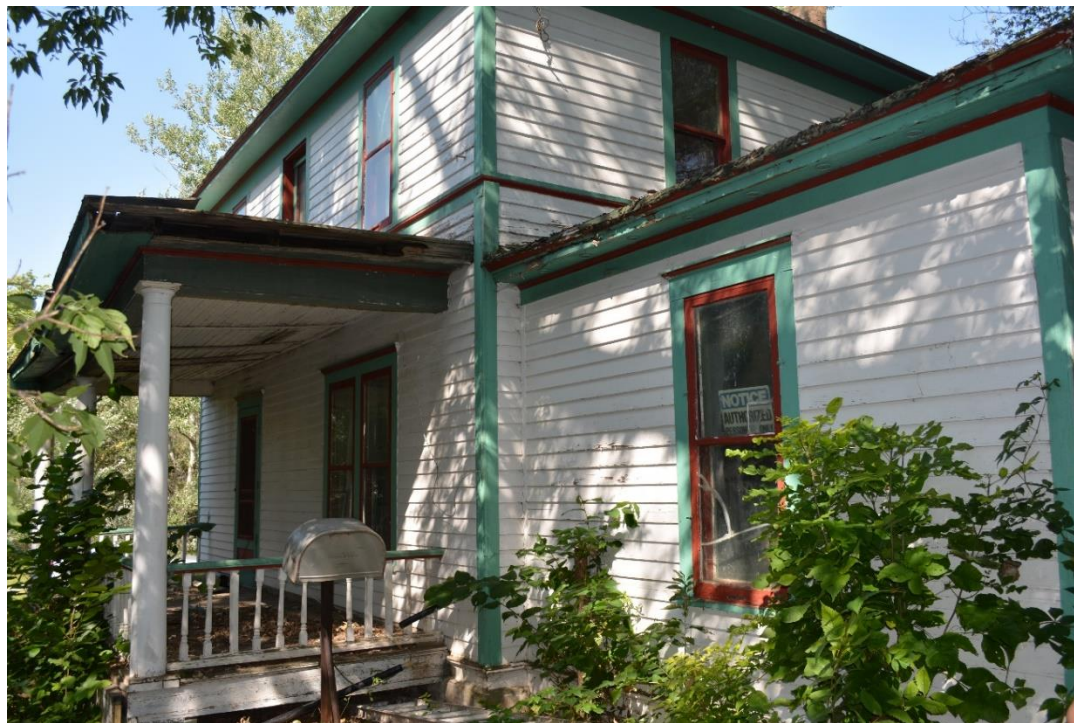
SD_Day County_Anderson House_0007: View of southeast corner, camera facing northwest.
