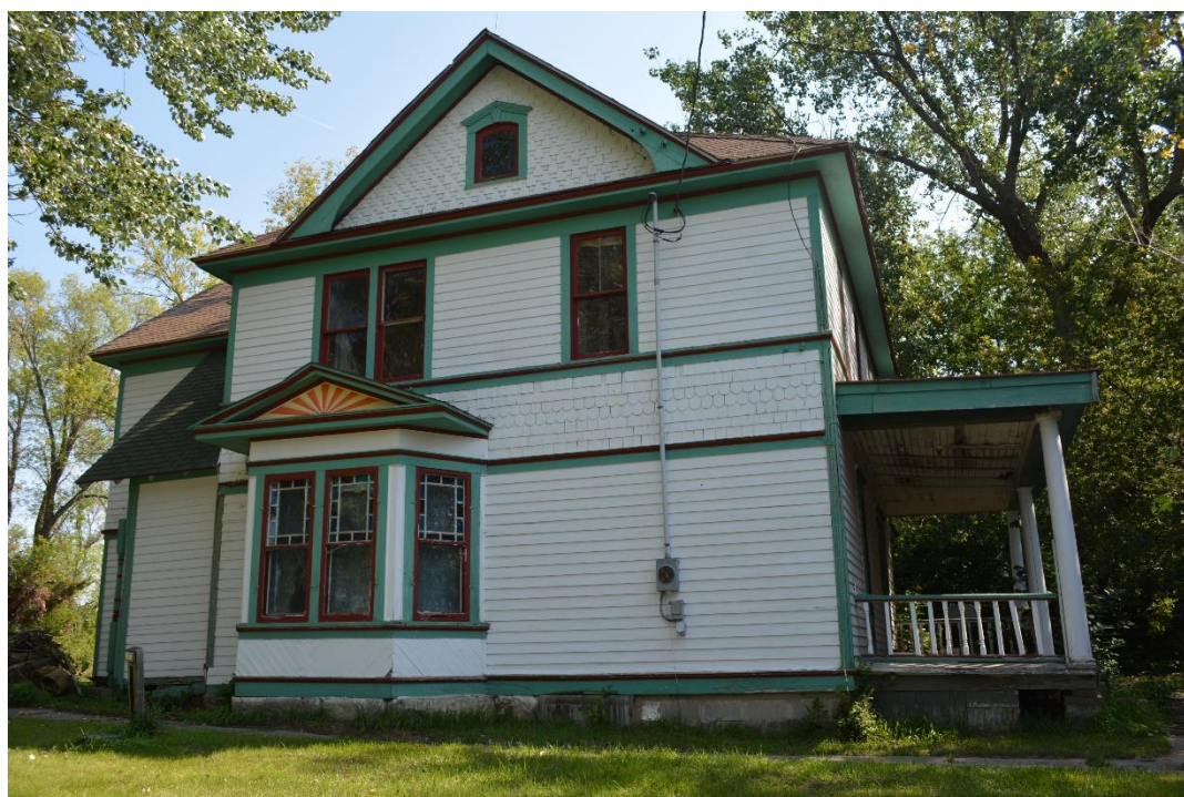
SD_Day County_Anderson House_0004: View of west façade, camera facing northeast.
