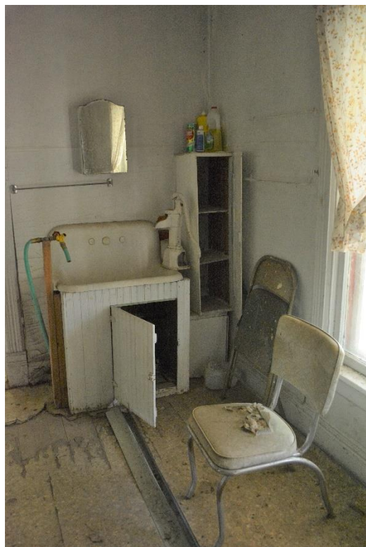
SD_Day County_Anderson House_0009: View of interior first floor (bathroom), camera facing southwest.
