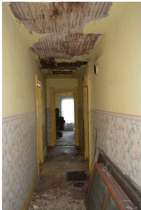
SD_Day County_Anderson House_0021: View of second floor hallway, camera facing north.
