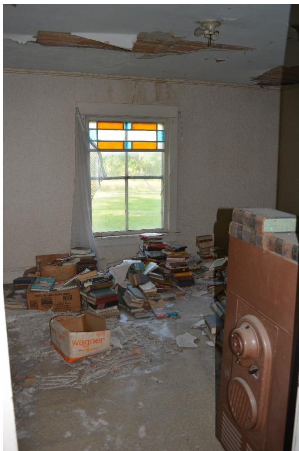
SD_Day County_Anderson House_0016: view of first floor interior, camera facing northeast.
