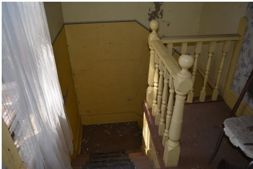
SD_Day County_Anderson House_0017: View of staircase, camera facing southwest.
