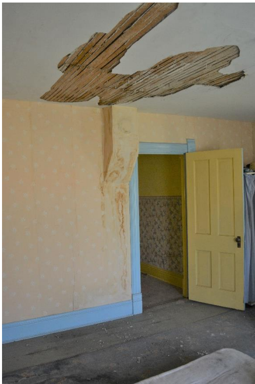
SD_Day County_Anderson House_0026: View of bedroom, camera facing southwest.
