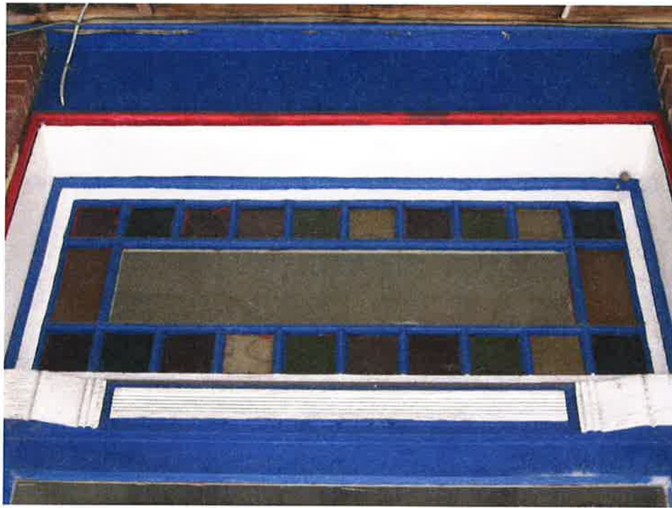
Preserve and maintain original transoms such as this border glass transom on the storefront at 6 Railroad Square.
