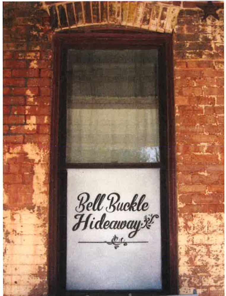
An original one-over-one wood-sash window at 3 Webb Road East.
