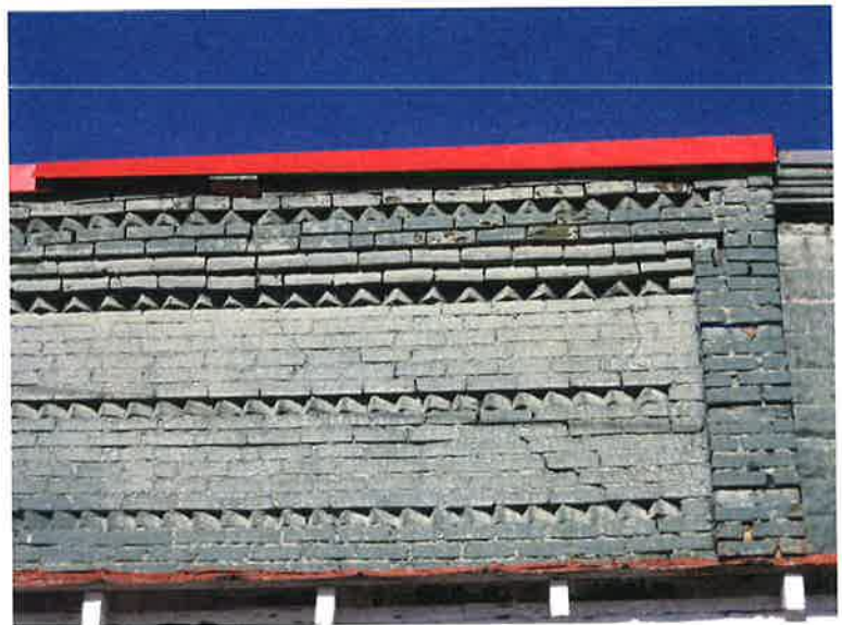
Masonry details such as corbelled brickwork can be found on many of Bell Buckle's commercial buildings (16 Railroad Square).
