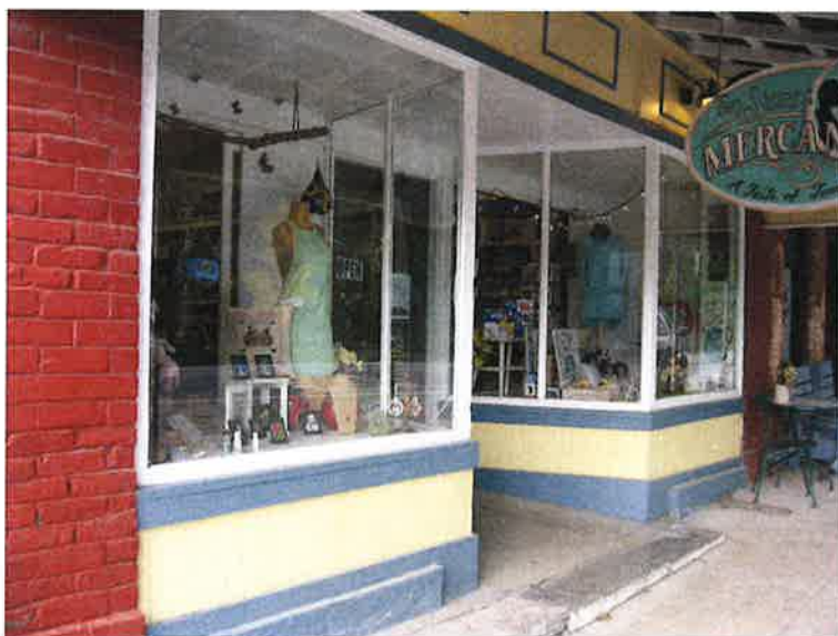
This original storefront at 3 Webb Road East retains its original frame bulkheads, display windows and recessed entrance.
