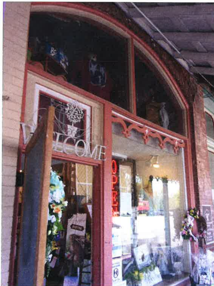
This arched two-light transom should be kept open and not covered or concealed (12 Railroad Square).
