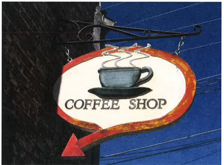
Projecting or "blade" signs are traditionally made of wood with metal hardware (2 Webb Road East).
