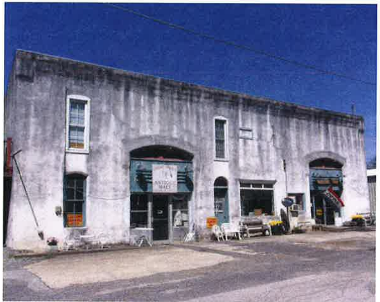
The 1899 livery stable at 107 Main Street has an added stucco surface which is now a historic feature of the building.
