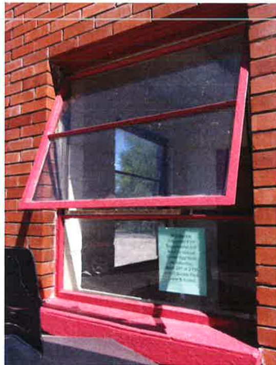
Mid-20th century metal windows should also be preserved and maintained (1 Webb Road East).
