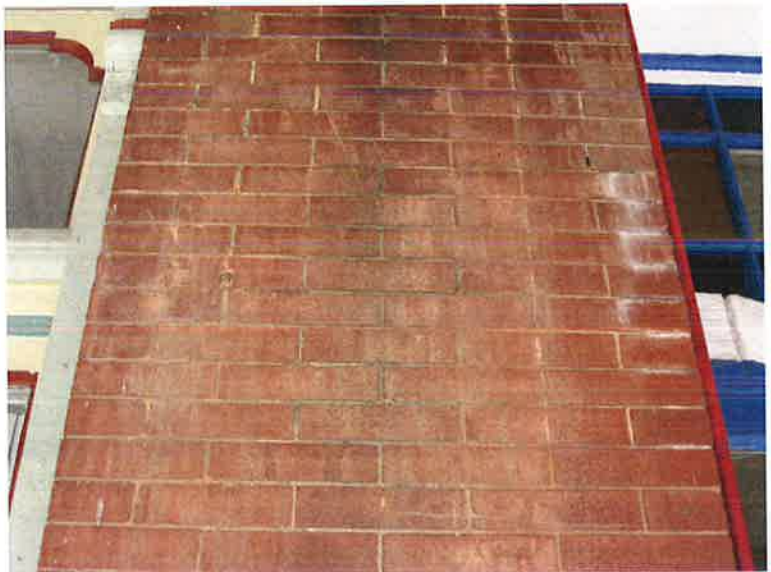
Maintain and preserve original brick walls and surfaces. Do not paint previously unpainted brick unless the brick is mismatched or deteriorated (8 Railroad Square).
