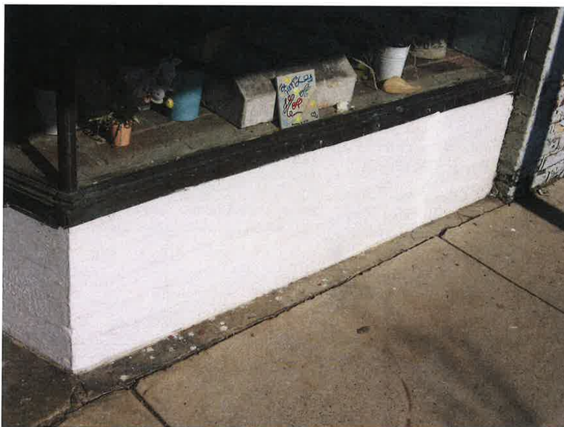
The storefront on the building at 2 Railroad Square has a bulkhead of poured concrete added ca. 1920.
