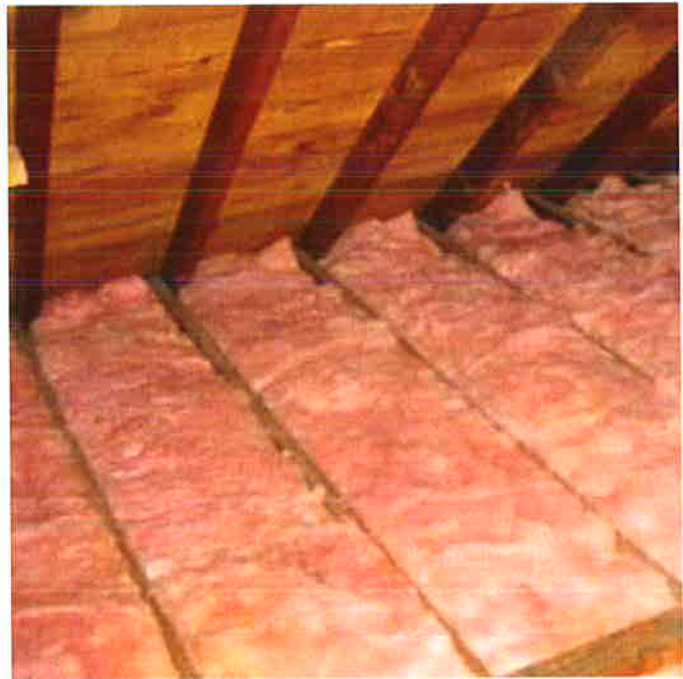
Adding ceiling insulation is one of the most cost effective methods of saving energy in commercial buildings.
