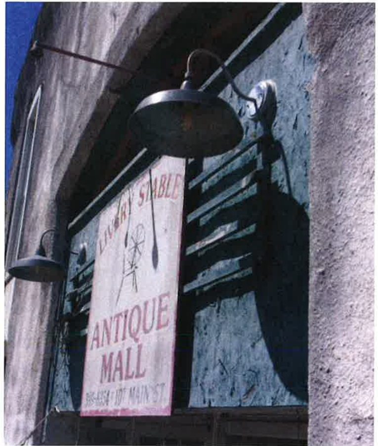
This traditional gooseneck light fixture provides illumination for the sign and storefront (107 Main Street).
