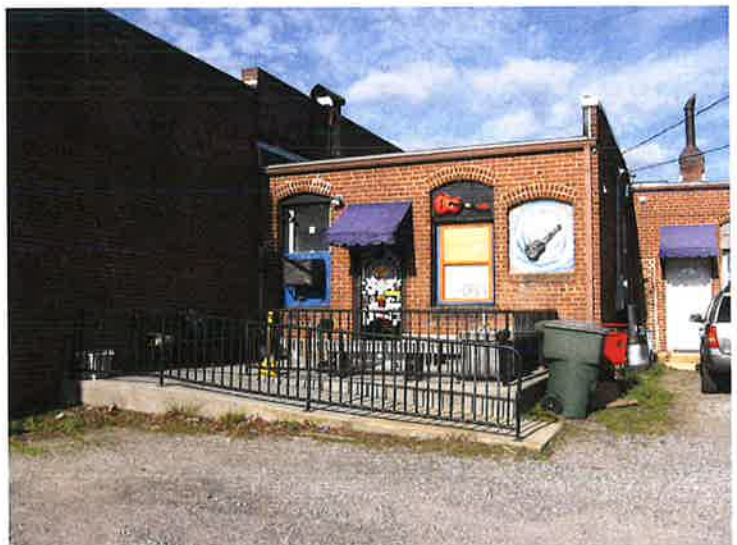
Example of a permanent ADA compliant ramp at the rear of this historic building.
