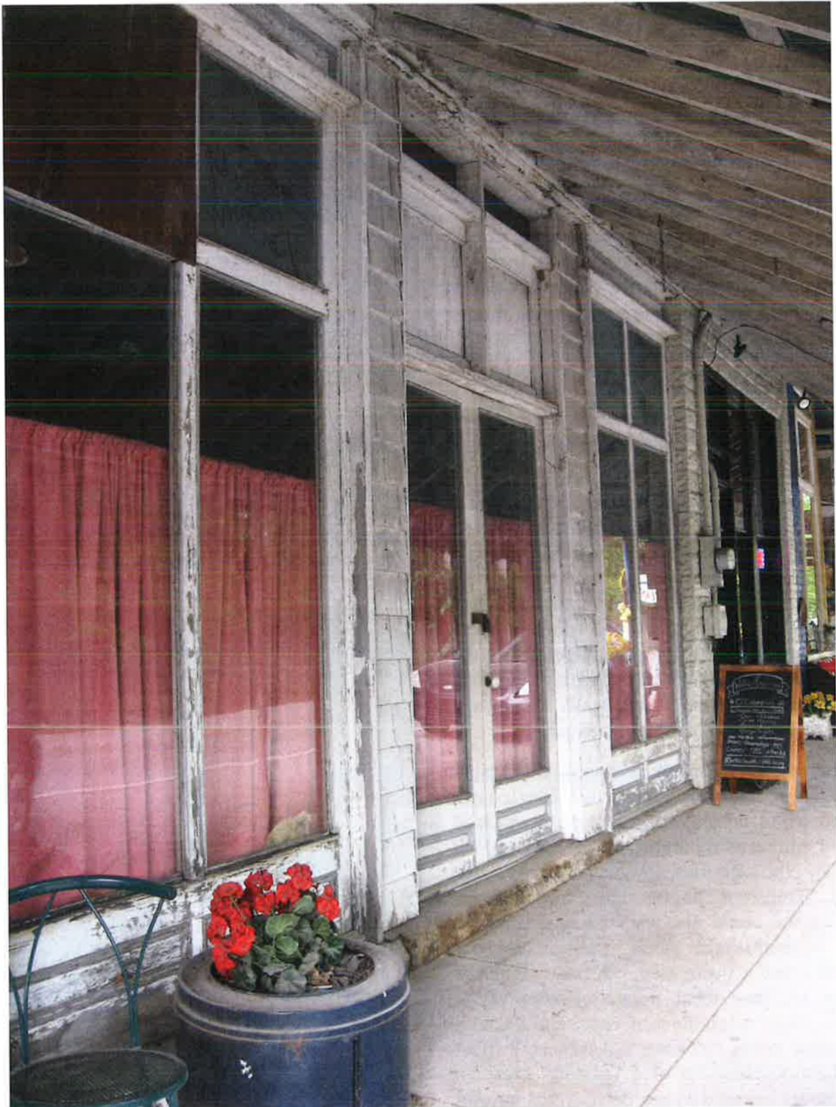
An example of an original storefront is the building at 5 Webb Road East which has its original display windows on frame bulkheads, transoms, and double door entrance.
