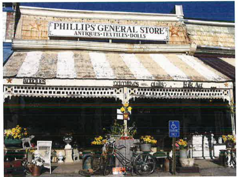
An example of a one-part commercial block is the building at 4 Railroad Square.
