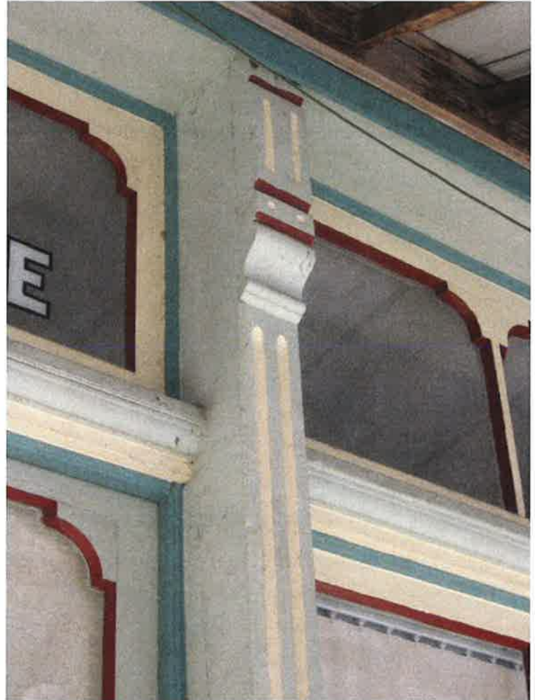
This original wood pilaster at 8 Railroad Square is a decorative element as well as providing structural support.
