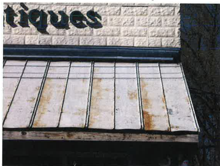
This crimped metal roof at 15 Webb Road East is typical of awnings in the downtown area.
