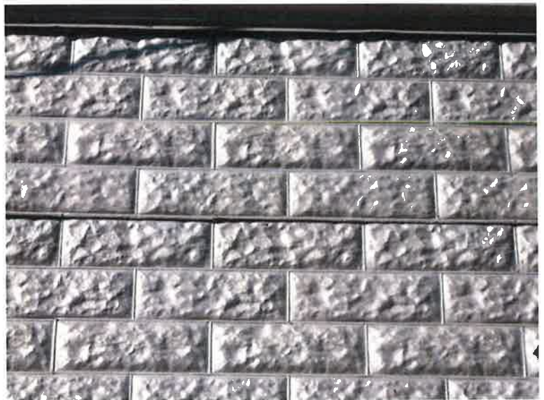
Pressed sheet metal adds a textured effect to some upper facades as at 5 Webb Road East.
