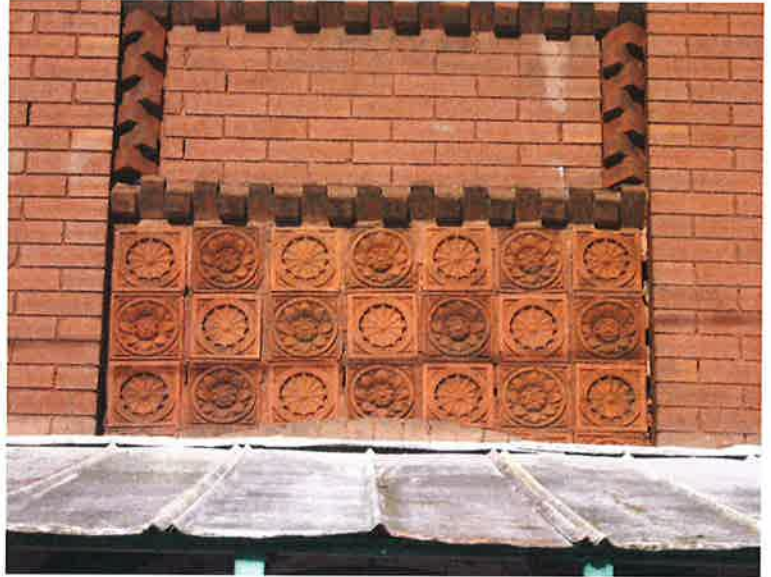
Brick and terra cotta masonry are decorative accents at 12 Railroad Square.
