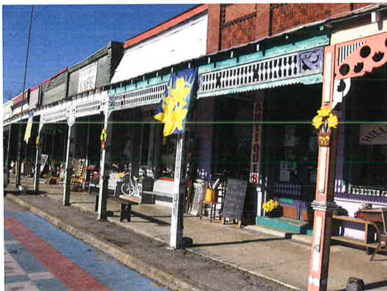
Row of metal and frame awnings on Railroad Square.
