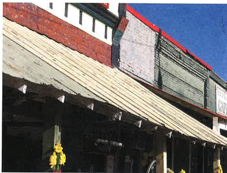
Awnings of wood with crimped or corrugated metal roofs are most common on Bell Buckle’s commercial buildings.
