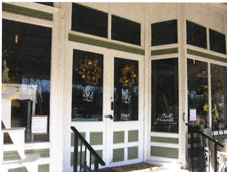
The commercial building at 24 Railroad Square has an original storefront with double doors flanked by display windows resting on bulkheads.
