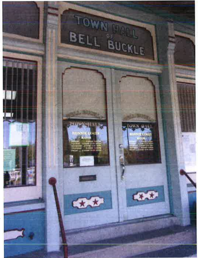
Town Hall of Bell Buckle offices are housed in a historic commercial building on Railroad Square.
