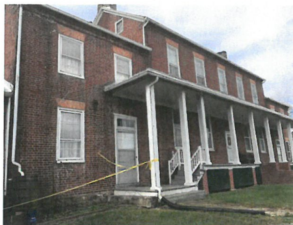
Right Rear Showing Back Porch
