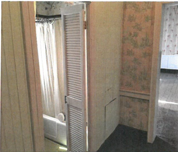
Stair 203 – Looking into Bathroom
