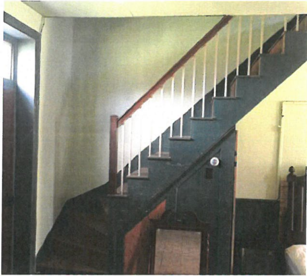
Room 105 – Stair to 205
