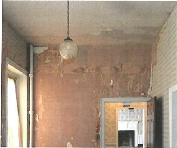
Anteroom 202 – Connector to Nursery and Stairway 203
