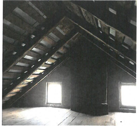
Attic Above Room 205 – End Wall/Chimney
