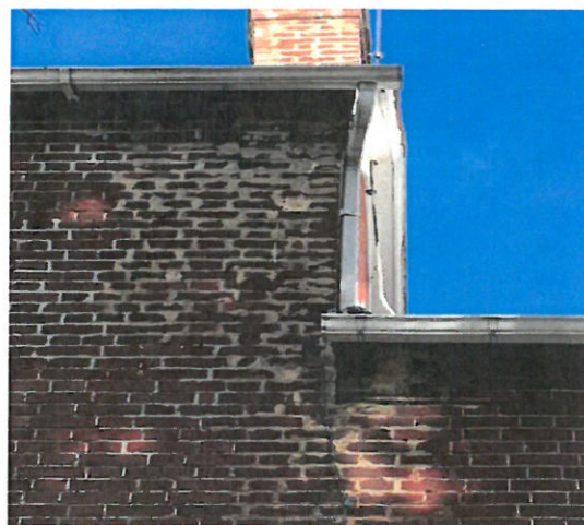
Close up of Previous Repointing
