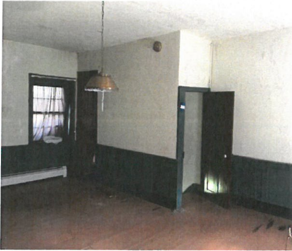
Bedroom 205 Male Wing – Showing Stair Down To Bedroom 105 and Attic Stair at Rear Wall
