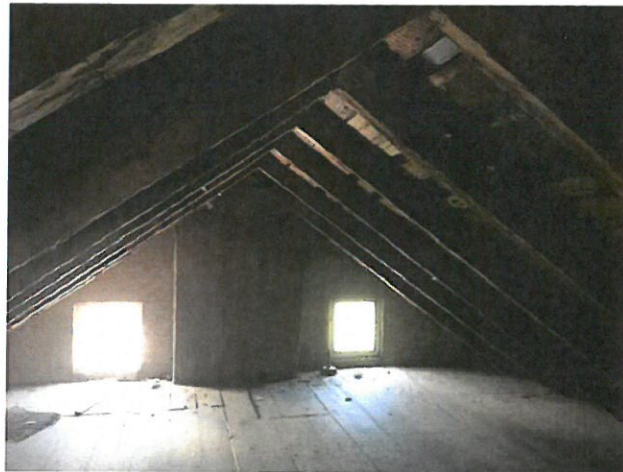
Main Attic – Left End and Room Framing
