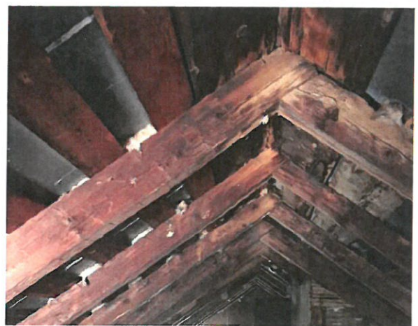
Main Attic – Looking Through to Left End
