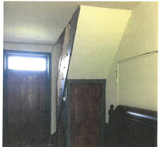
Room 105 – Rear Entrance and Under Stair Closet
