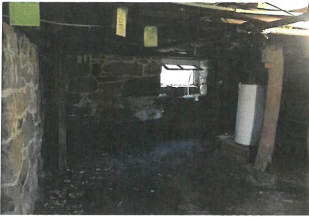
Basement Room 1 – Front Wall
