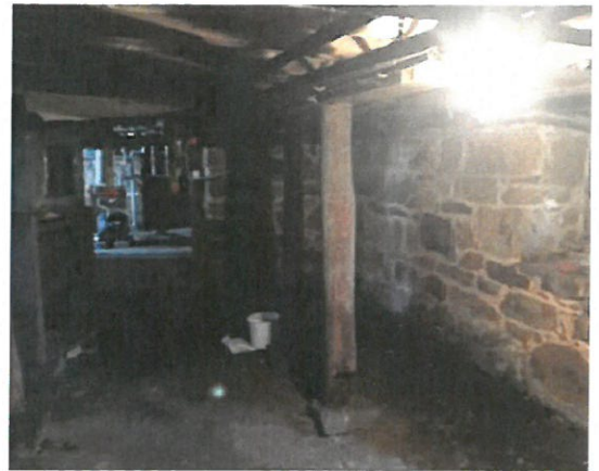
Basement Room 1 – Looking Down Rear Passage to Room 2
