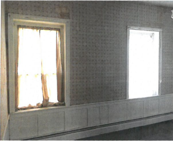
Nursery Room 202 – Rear Wall
