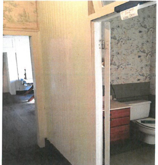
Stair 203 – Looking into Bathroom
