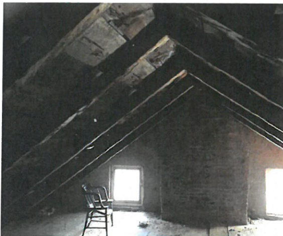
Main Attic – Right End and Roof Framing
