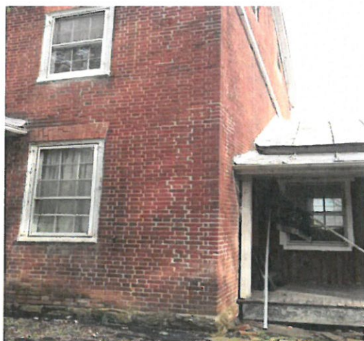
Right Front Kitchen End – Previous Repointing From Foundation to Roof
