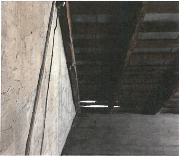
Attic Above Room 205 – Front Wall Eave Room Framing
