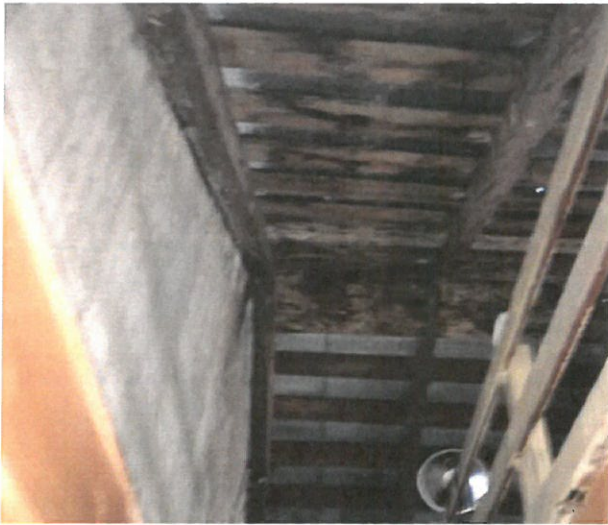
Attic Above Room 205 – Stair
