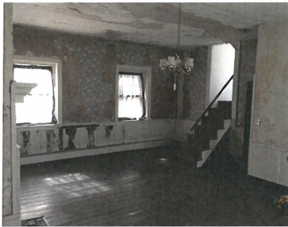
Bedroom 201 – Front Wall and Steps up to Room 202
