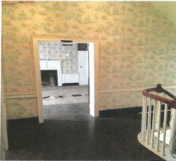
Stair 203 – Looking into Bedroom 204
