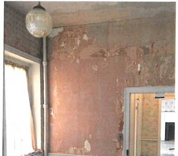
Anteroom 202 – Doorways to Stair and Room 204
