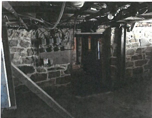
Basement Room 2 – Looking at Passage to Room 1
