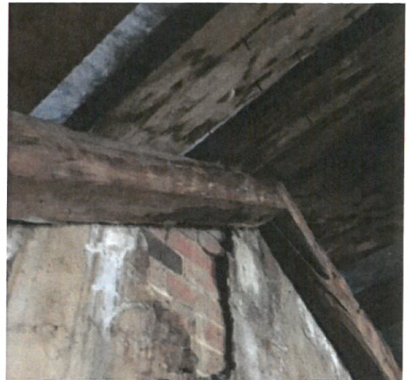
Attic Above Room 205 – End Wall
