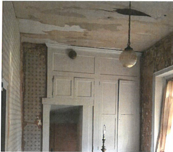
Anteroom 202 – Cabinetry and Passage Down to Room 201
