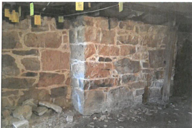
Basement Room 1 – Right End Foundation Wall
