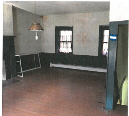
Bedroom 205 – Rear Wall and Stair Down to Room 105
