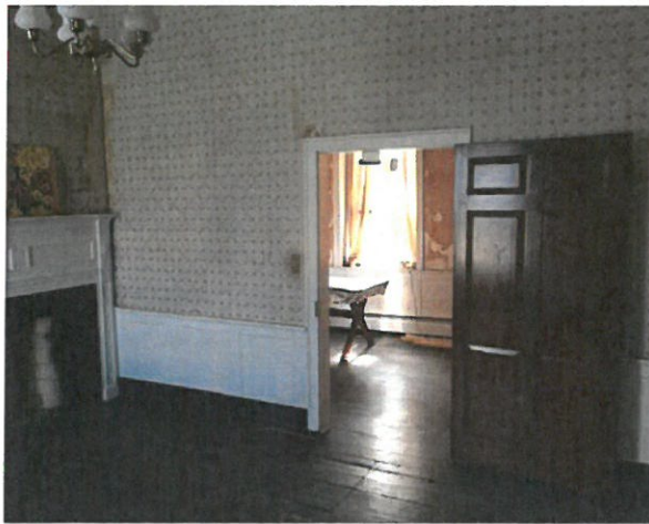
Nursery 202 – Interior Partition with Door to Anteroom
