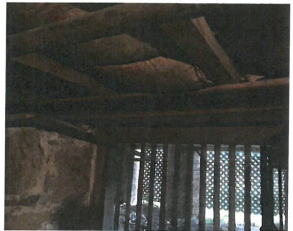
Basement Room 2 – Grated Window Under Rear Porch
