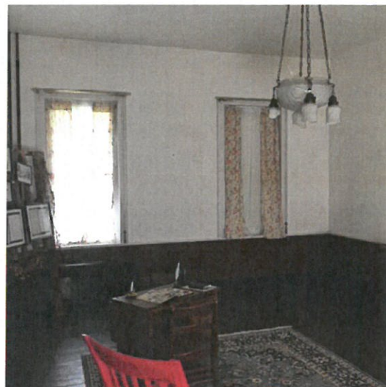
Parlor 104 – Rear Wall
