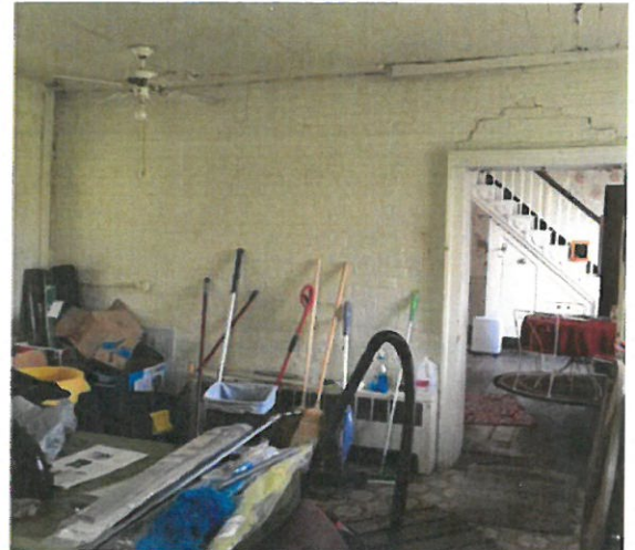
Kitchen – Inside Wall
