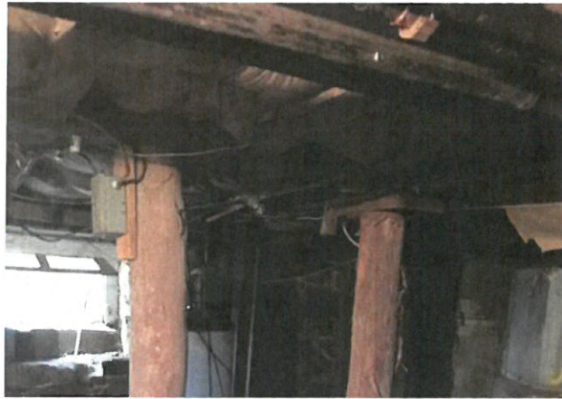
Basement Room 1 – Supplementary Timber Support Columns
