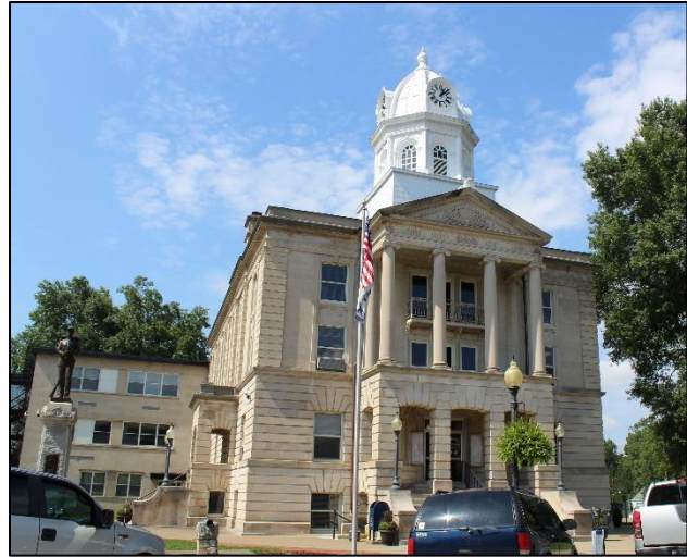
Figure 8. HPI Site Number: JA-0005-0001, Jackson County Courthouse, Ripley.
