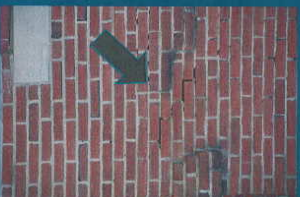
Minor masonry tuckpointing
