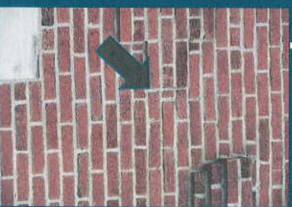
Minor masonry tuckpointing
