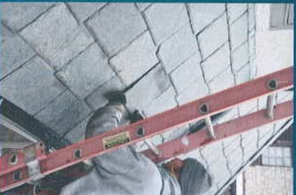
Replacement of individual shingles
