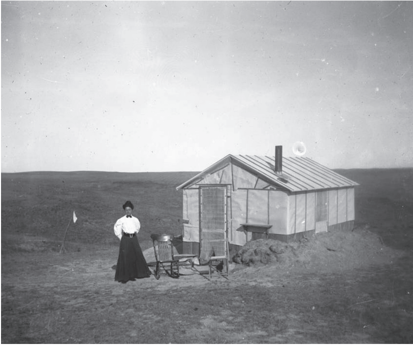
Like many tar-paper shacks, this one was partially sodded for extra insulation.
