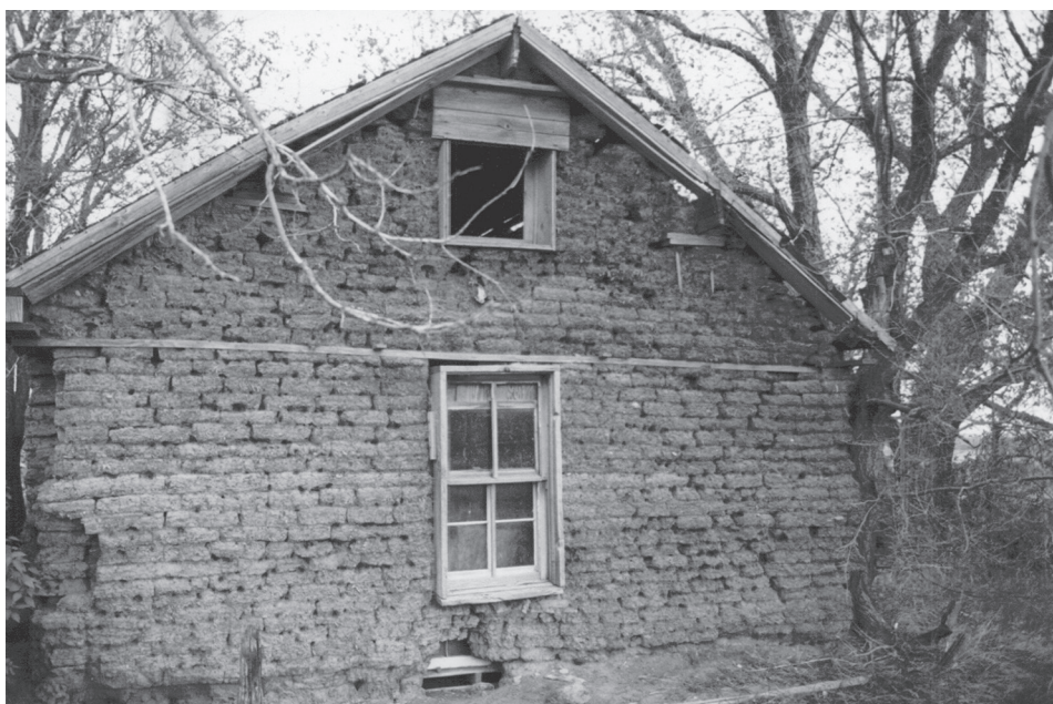
The west facade of the Dragoo soddy featured both double-hung and half windows. Also visible are the lumber planks staked in the sod, on which the plank purlins rest, and the eave plate board that runs across the wall above the lower window.
