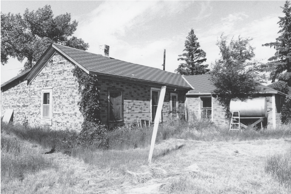
This 1990 view of the northeast side of the Penor sod house shows the two-room frame house added on in 1911 and the shed-roofed kitchen addition built in the 1940s.
