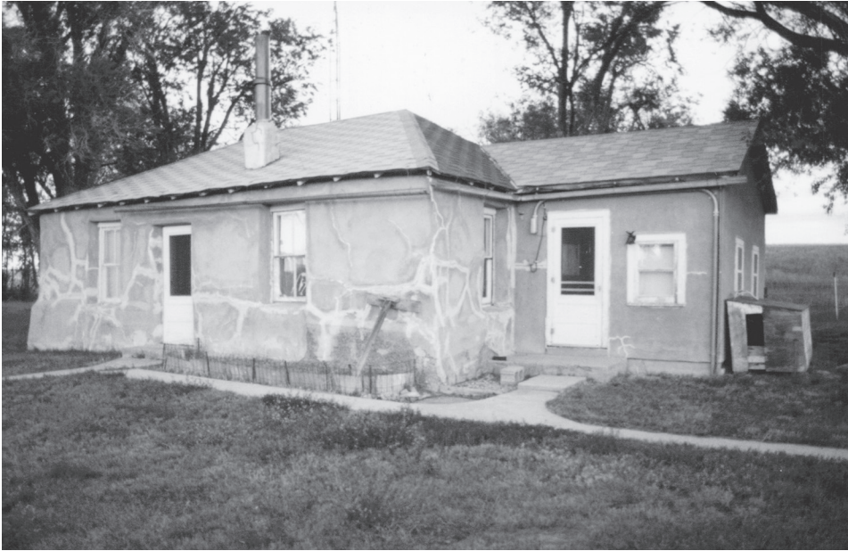
Cracking stucco, as seen on the Bekken sod house, meant continual patching and other maintenance chores for owners.
