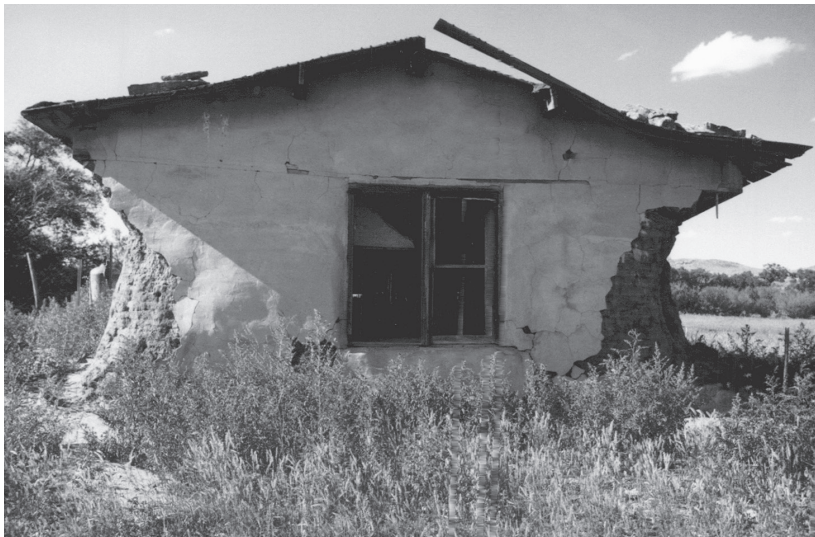
The deterioration of sod structures can be accelerated by numerous factors, including damage caused by cattle rubbing against the building's corners.
