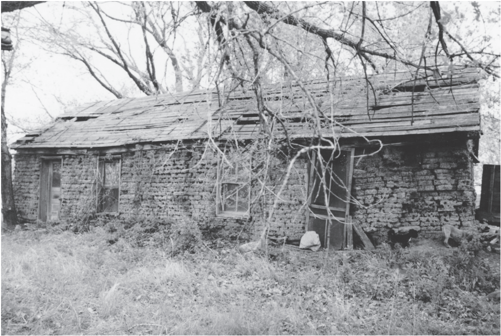
This south view of the Dragoo soddie, photographed in 1990, highlights the extensive use of lumber in the roof.
