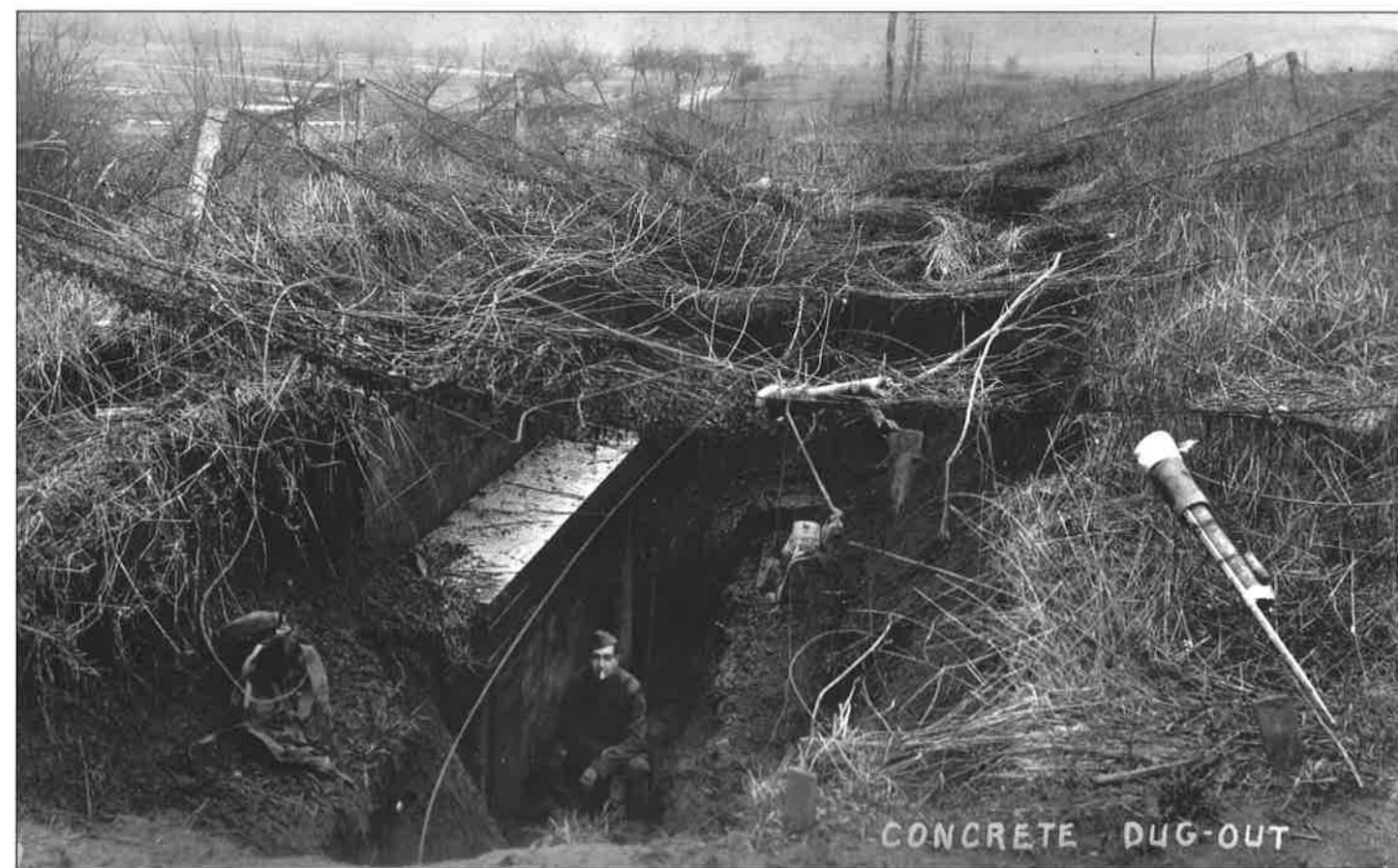
Concrete dugout, France, 1917–19. SHSND SA 00171-00009
