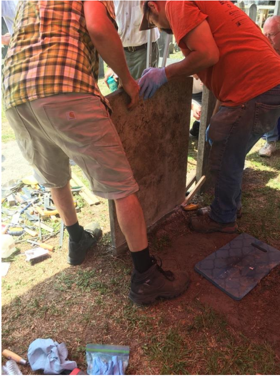
Repinning (graphite pins) and epoxy repair demonstrations
