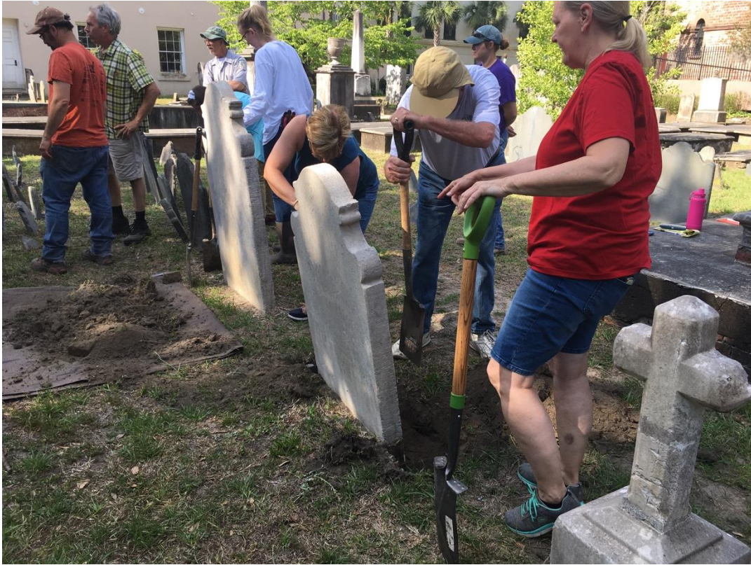
Workshop attendees reset a series of settling/crooked monuments, working with line levels and plumb lines
