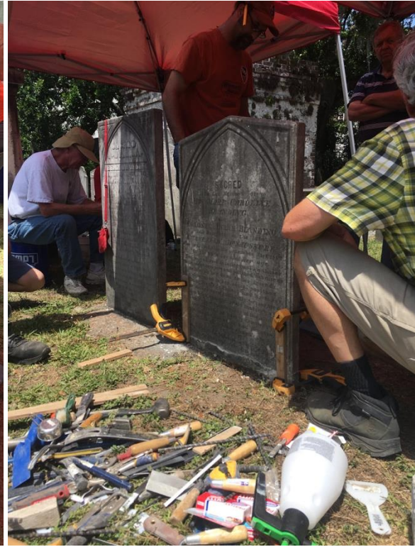
Repinning (graphite pins) and epoxy repair demonstrations
