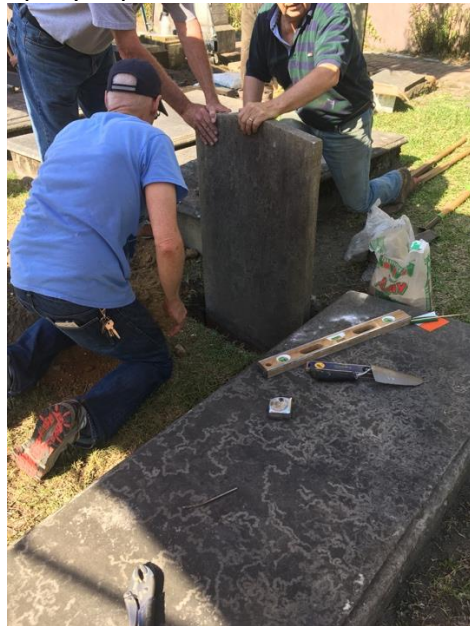
Resetting work, on gravel and with mortared brick below grade independent foundations.
