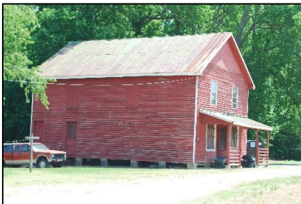
Photograph 30. Willie B. Hopkins Store (WA1879)
