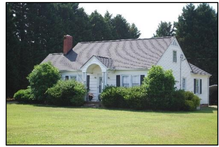
Photograph 17. Daniel House (WA7842)
