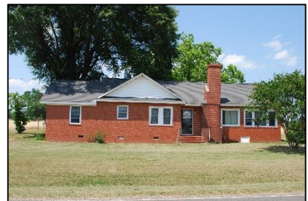
Photograph 20. Charlie Debham House (WA8175)
