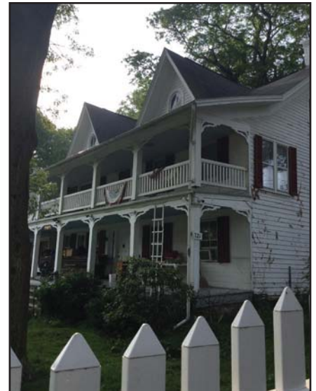
721 Fifth Avenue 66-003-109 Springside / Woodward-Glosser House
