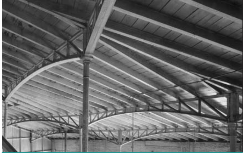
B&O Roundhouse roof system Martinsburg, Berkeley County
