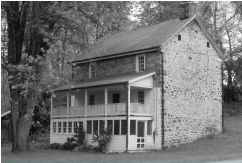
Switzer House, Wardensville Hardy County
