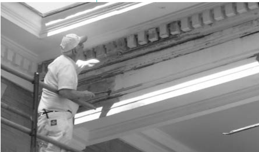
Capito House (now Jarrett Construction offices) Charleston, Kanawha County - in progress (tax credit)
