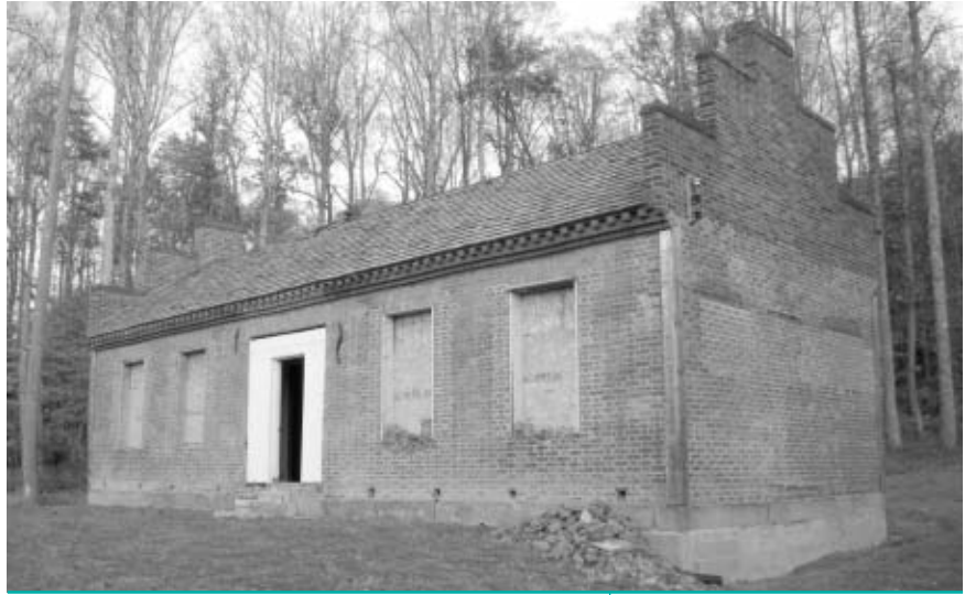
Hoge House, Winfield Putnam County during restoration
