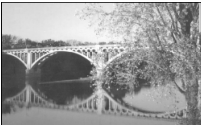
The George Rogers Clark - Lincoln Memorial Bridge spans the Wabash River at Vincennes. This finely detailed bridge was built with concrete open-spandrel arches in 1932. (Indiana Scenic Images)
