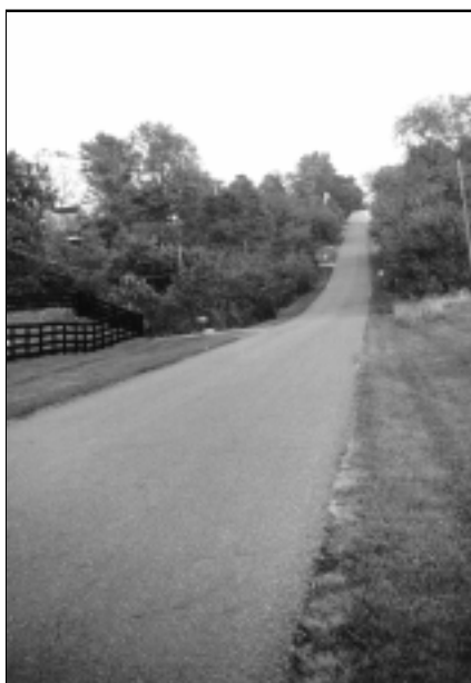
A section of the National Road rolls through Henry County. The DHPA is assisting the Indiana National Road Association with the designation of the Old National Road (U.S. 40) as a scenic byway. (DHPA files)
