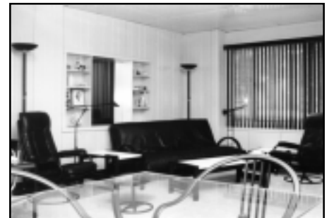
An interior view of the Coombs House shows that this 1950 Lustron home is remarkably intact. The walls and ceiling are composed of metal panels, like the exterior of the house. (DHPA files)
