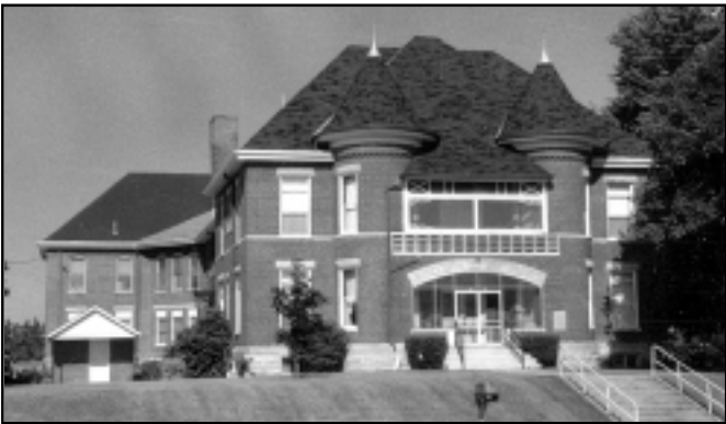
The Randolph County Infirmary near Winchester was built in 1899. This impressive, architect-designed building was the third infirmary built in the county. This building is unusual in that it still serves its original purpose. (DHPA files)
