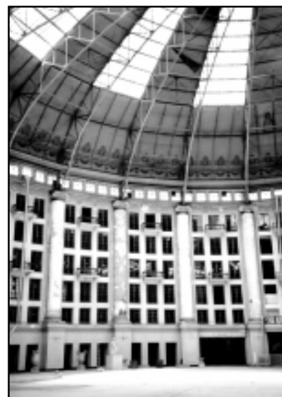
Once a grand and elegant resort, the former West Baden Springs Hotel sat vacant and deteriorating during the 1980s. Recent restoration work, coordinated by Historic Landmarks Foundation of Indiana, has begun to return the hotel and grounds to their former glory. (Amy Johnson)
