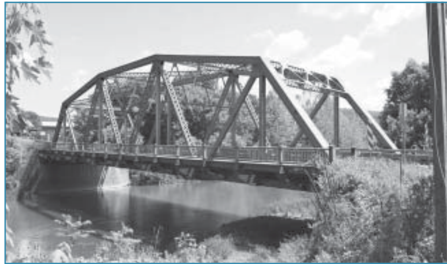
1941 steel truss bridge, Steuben County.
