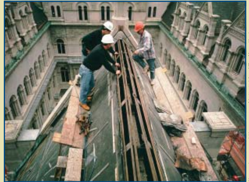
In-kind roof replacement has been one of the most important elements of the State Capitol's ongoing restoration. Photograph: Bernstein Associates.
