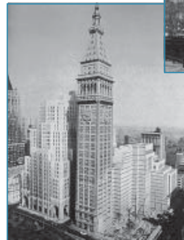
Metropolitan Life Insurance Company headquarters c.1958 — North and Tower Buildings with the South Building under construction.
