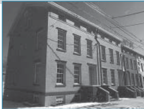
175 Lander Street before and after rehabilitation.
