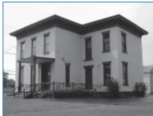
Harriet May Mills House.
