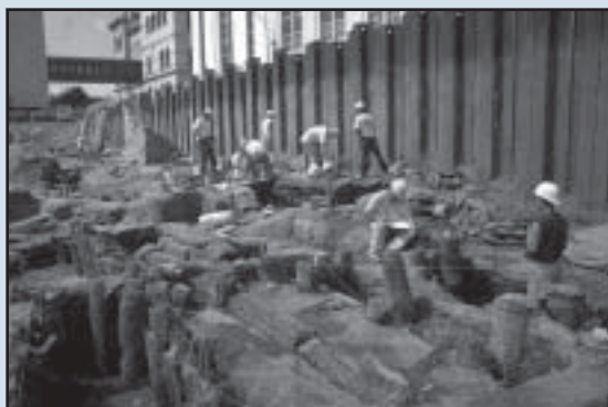
The excavation revealed a wide range of features, including the remains of the city's early waterfront.
