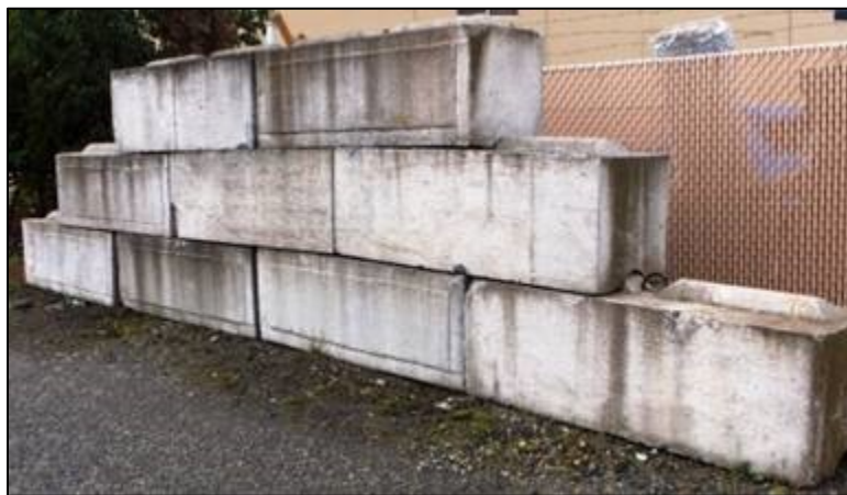
Figure 12: Example of an ECO Block wall that could be stacked up to provide greater protection to homes/values at risk below the burned area.
