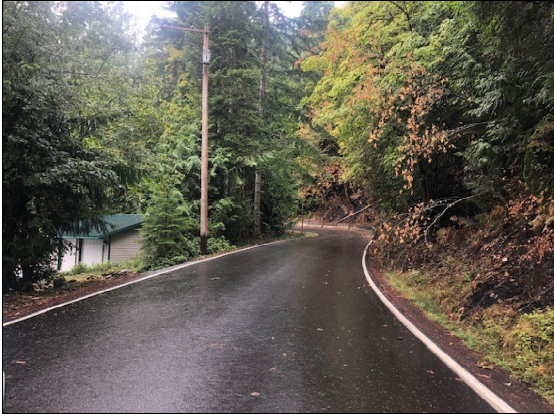
Figure 10: Picture of private home and utilities at risk from rockfall and treefall.
