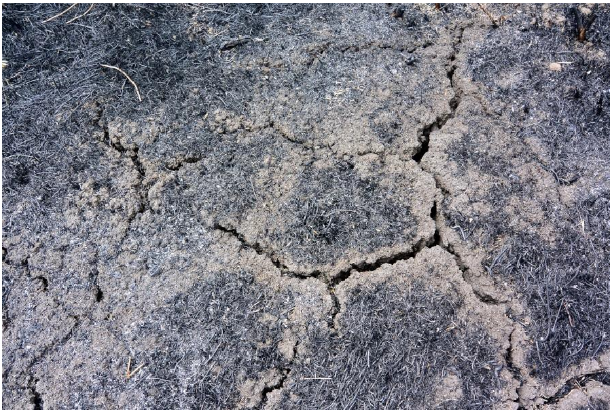
Photo 8 – Cracked Vertisols in the burn area containing high clay content.
