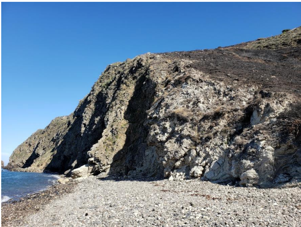
Photo 2 – Burned slope above coastal cliff at Scorpion Anchorage vulnerable to rock-fall.
