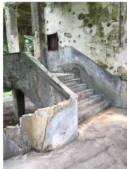
Figure 17. Interior Staircase at Japanese Air Headquarters
