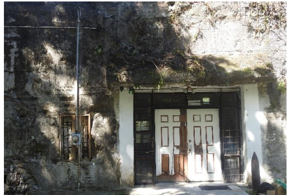
Figure 10. Exterior Conditions of Museum Building
