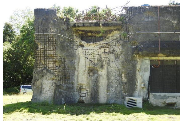
Figure 9. Exterior Conditions of Museum Building
