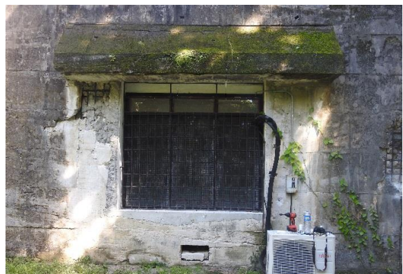
Figure 11. Exterior Conditions of Museum Building
