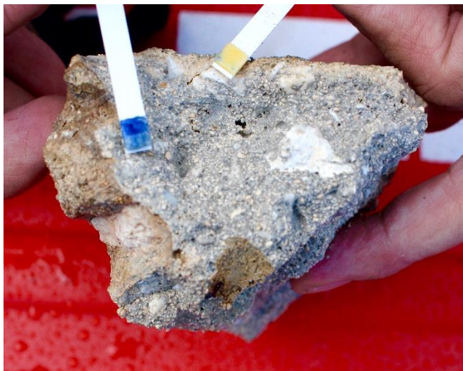
Figure 22. Freshly broken concrete sample taken at parapet, showing carbonated and non-carbonated zones. The carbonated zones can be identified by the warm color tone of the cement matrix (yellow litmus) and non-carbonated by the gray-tone cement matrix (blue litmus)
