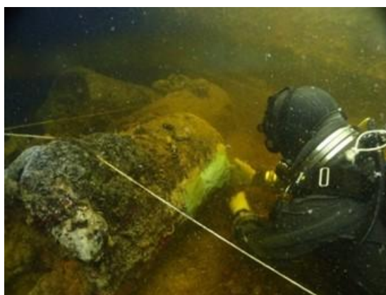
2. Sealing operation by a JMAS diver
