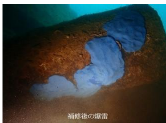
4. After sealing with epoxy resins
