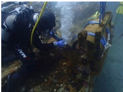
5. Removal work with an air saw
