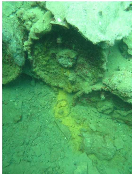
Figure 6-6. Picric acid leaking observed during 2015 diving investigation
