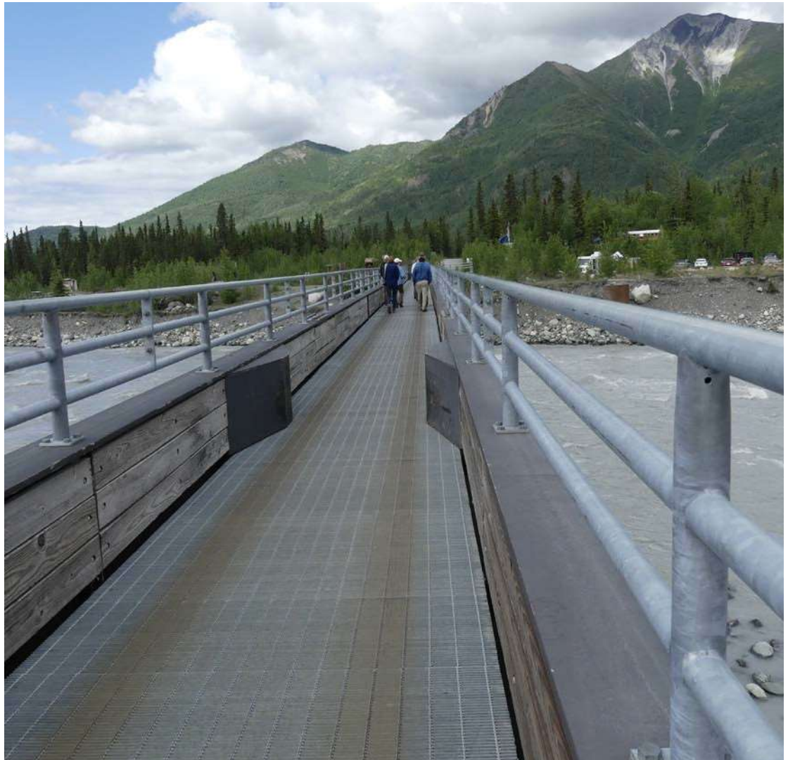
The West Footbridge over the Kennicott River to McCarthy.
