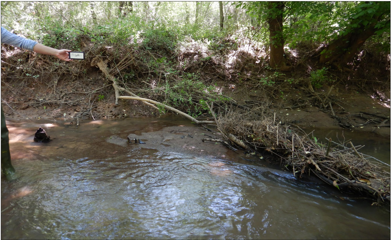
Figure B-4. Photograph taken on OCMU001 looking at the left bank on T1 (detailed transect 1).
