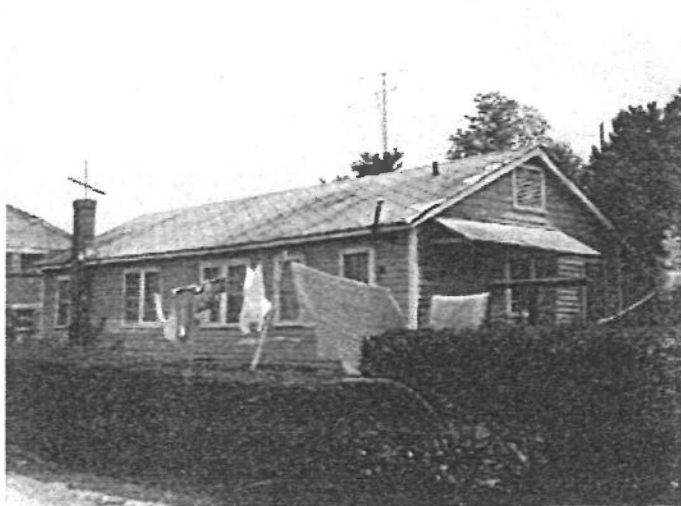
Figure 5: 1977 photograph of the west rear and north side facades of the Army Supply Building. Booker Conley's Files, Physical Plant, Tuskegee University.
