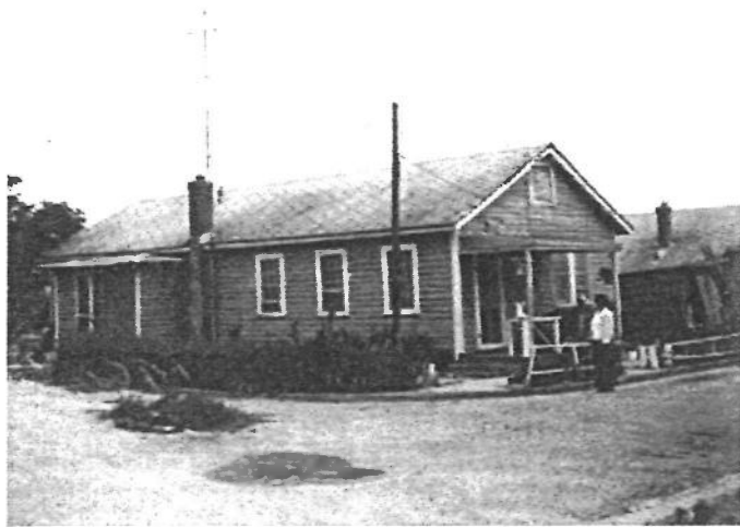
Figure 4: 1977 photograph of the east front and south side facades of the Army Supply Building. Booker Conley's Files, Physical Plant, Tuskegee University.
