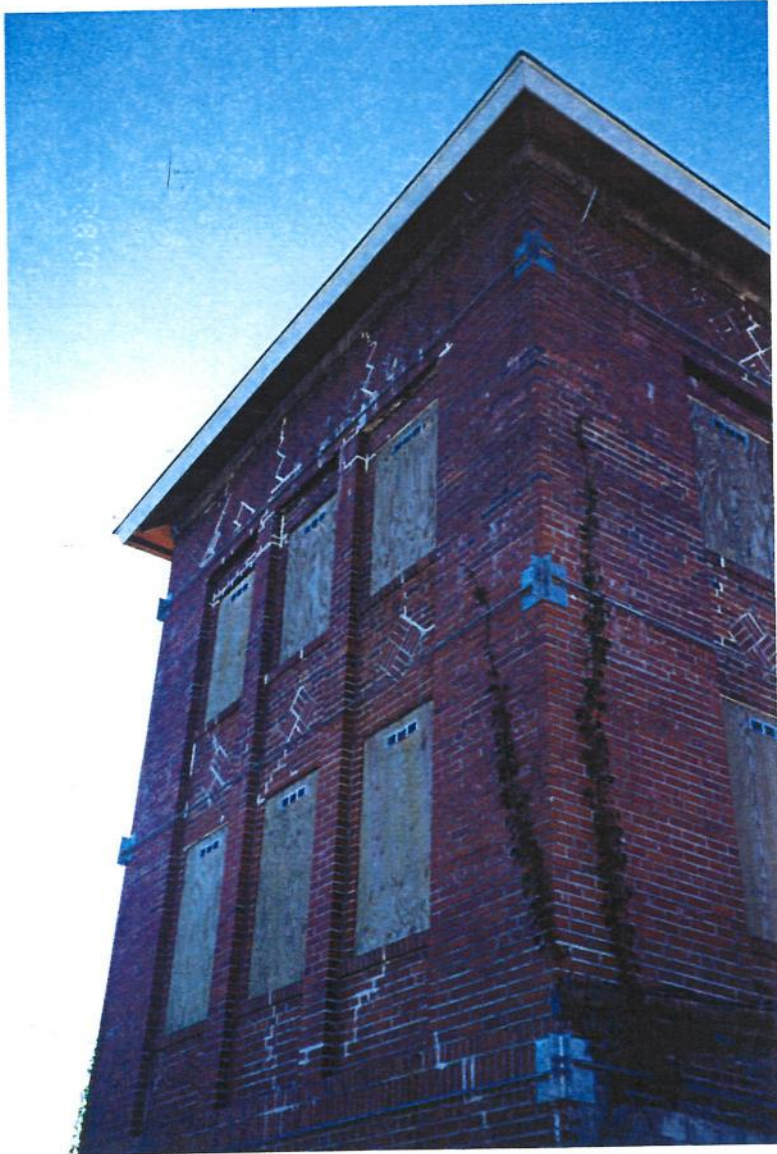
Photo 2. Control Tower Building – West Face
