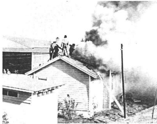
Figure 4: Working to put out the fire on the heater room roof circa 1944. Historic Photograph Collection, Howard University.
