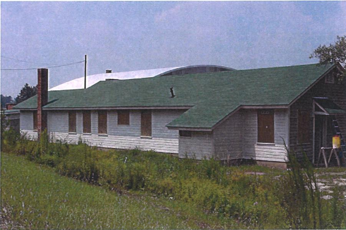
Figure 9: Existing south rear facade.
