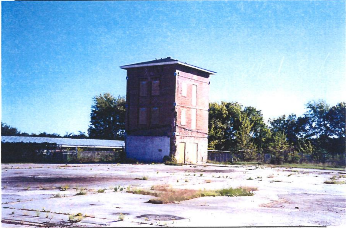
Photo 1. Control Tower Building
