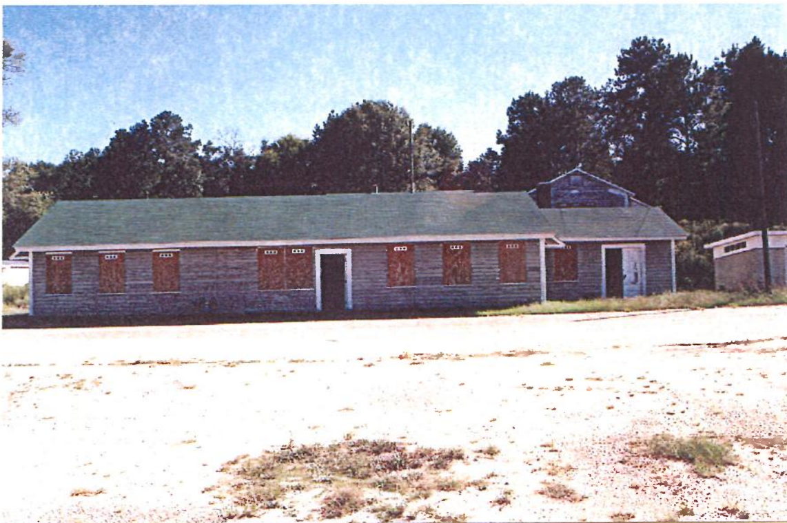
Figure 8: Existing north front facade.
