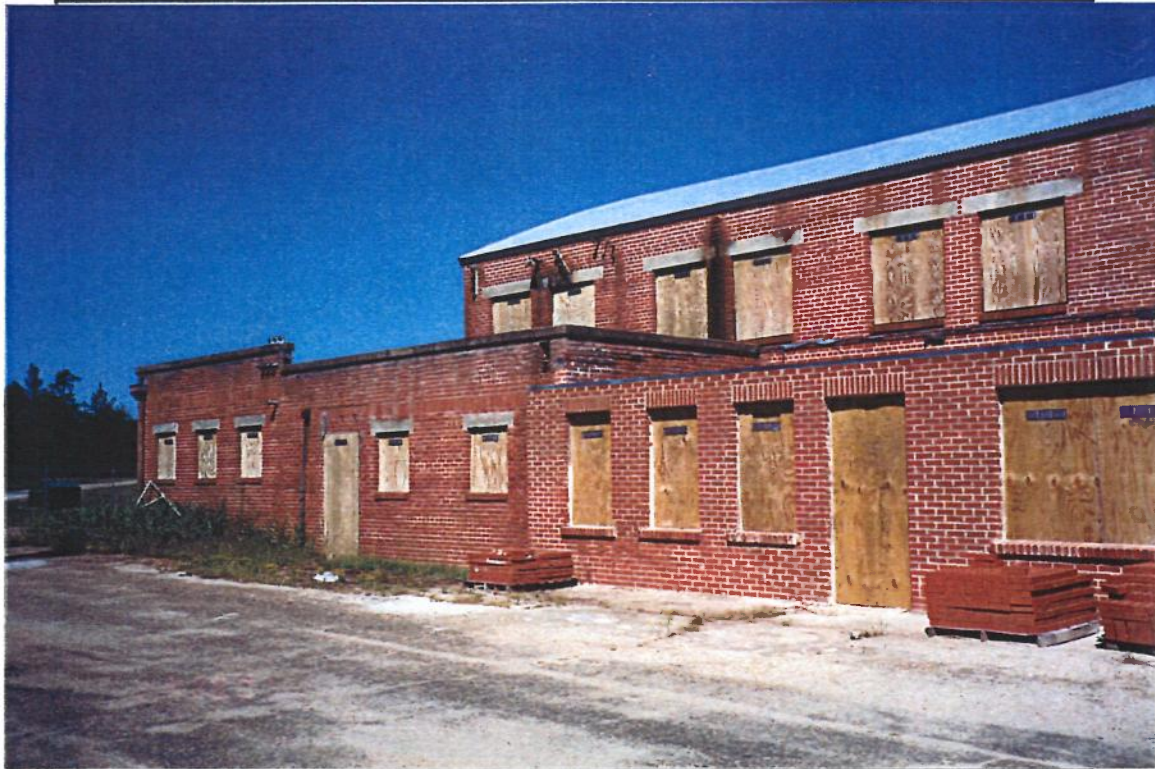
Photo 9. Hangar No. 1 – South Face
