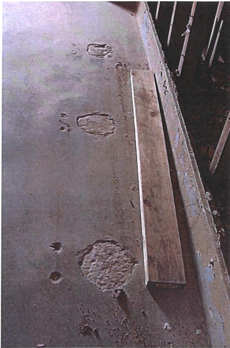
Figure 10: Former location of toilets in men's toilet room.
