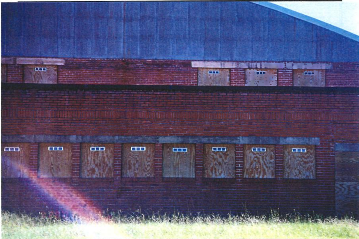
Photo 8. Hangar No. 1 – West Face
