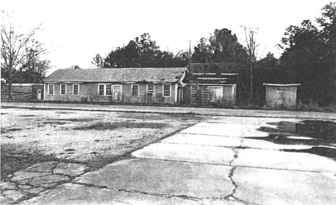
Figure 6: North facade in 1997 prior to stabilization. National Park Service, SERO, Atlanta, Georgia.
