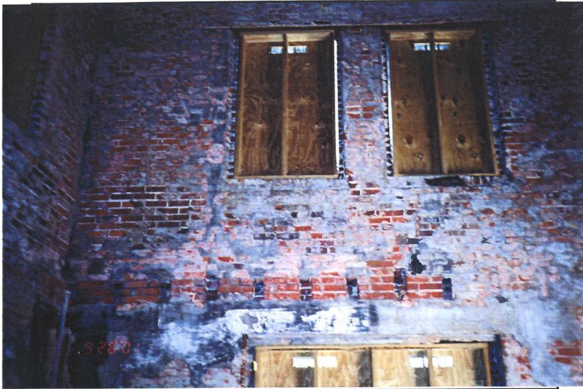
Photo 3. Control Tower Building – Interior North Face
