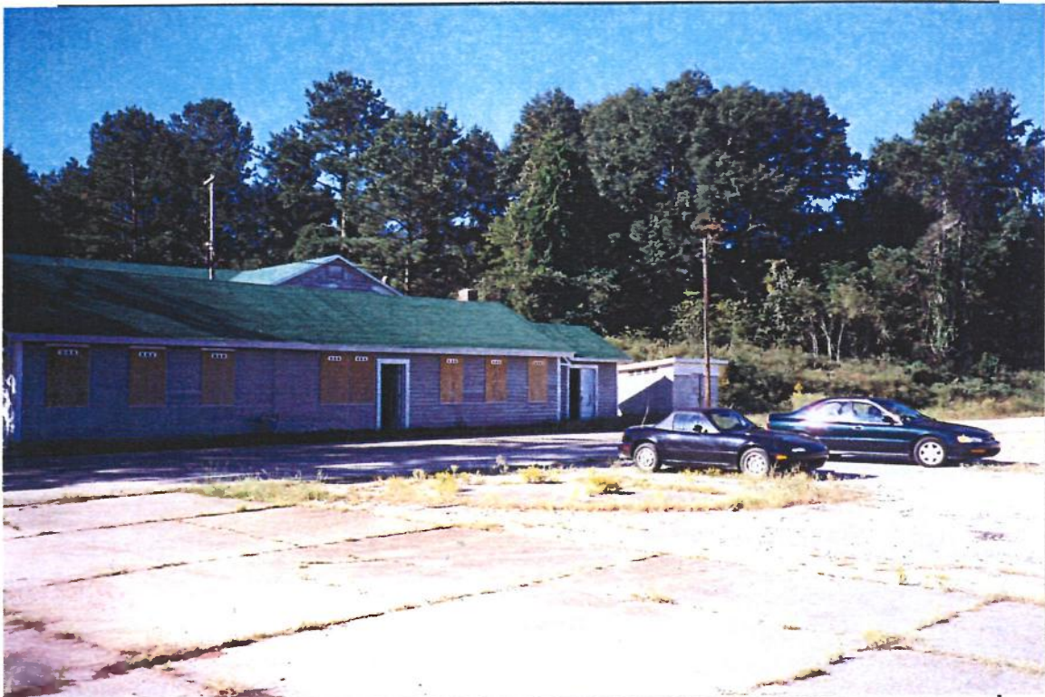
Photo 18. Bath and Locker House – East Face
