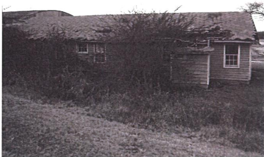
Figure 7: South facade in 1997 prior to stabilization. National Park Service, SERO, Atlanta, Georgia.
