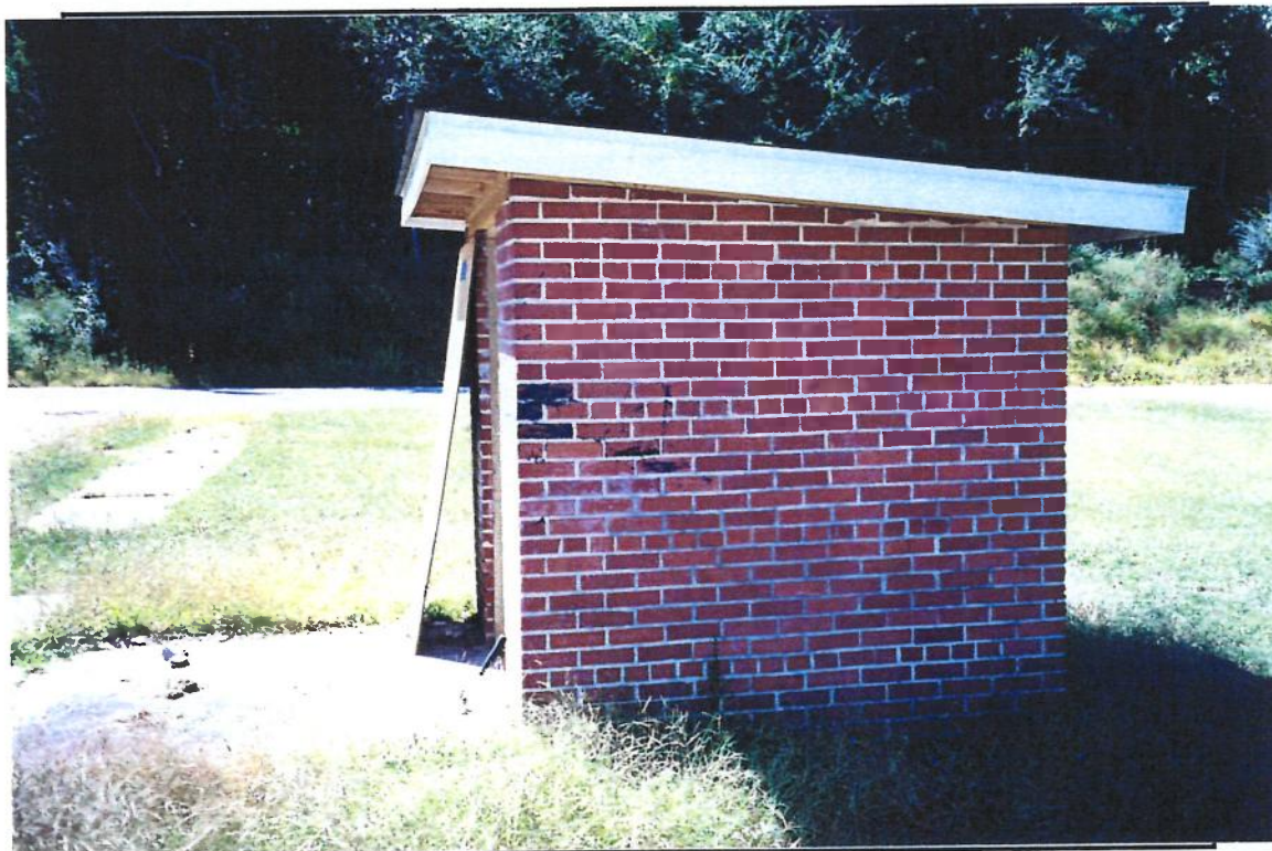
Photo 14. Fire Protection Shed – East Face
