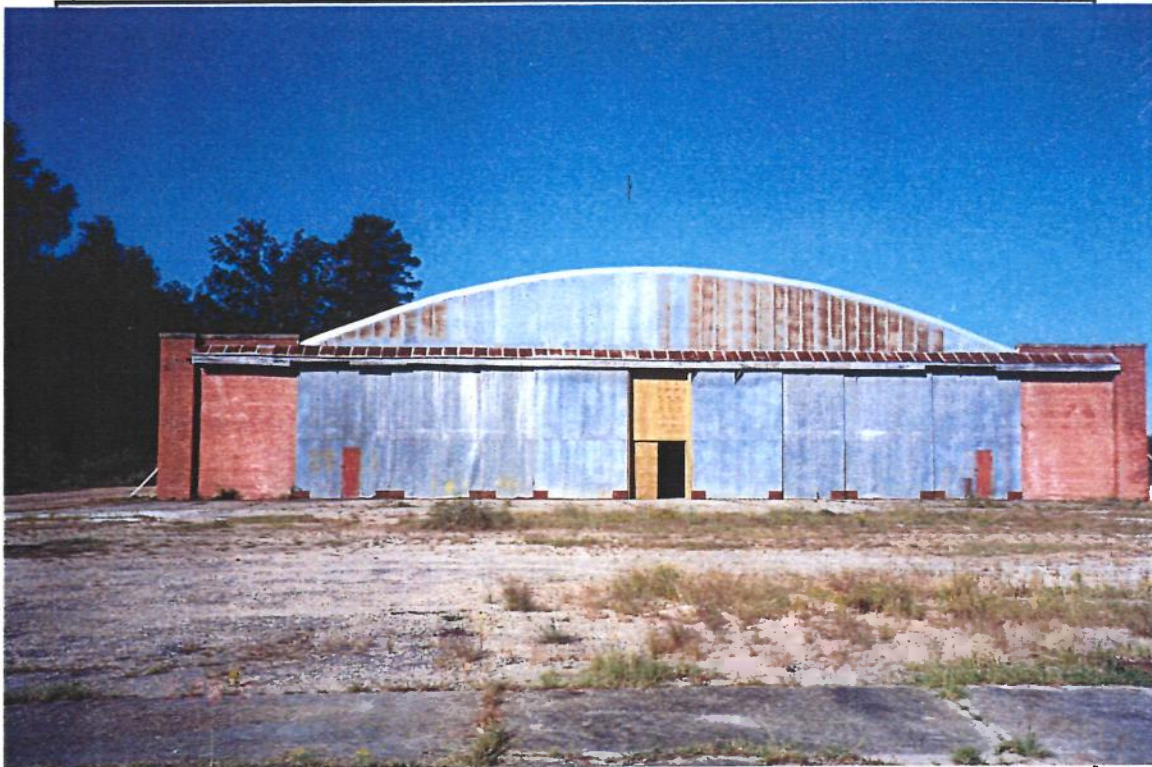
Photo 7. Hangar No. 1 – East Face
