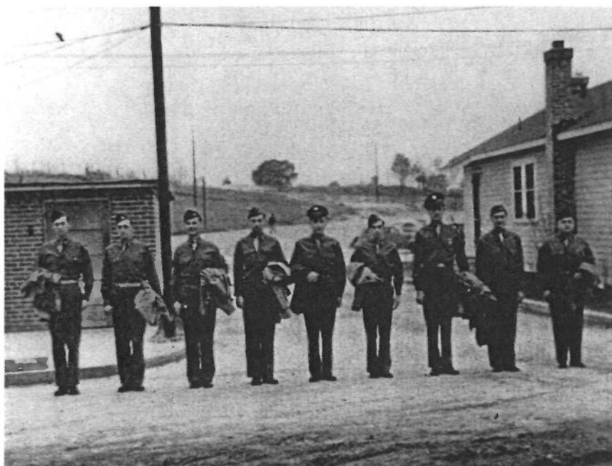
Figure 6: Historic photograph showing the south facade of the Cadet Class and Waiting Room (far right). Historic Photograph Collection, AFHRA, Maxwell AFB.
