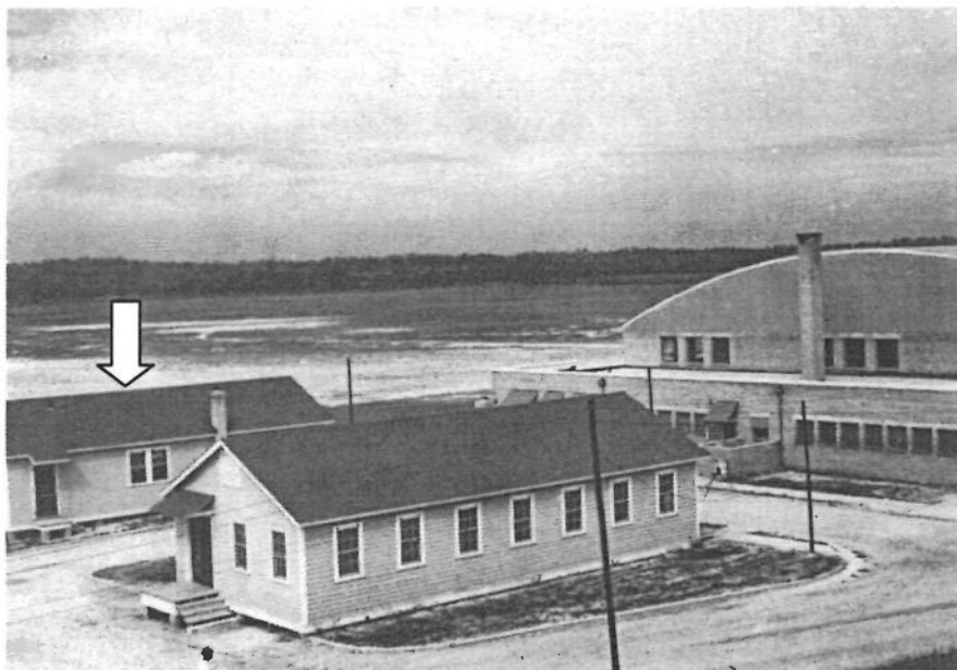
Figure 5: Historic photograph of the Cadet Class and Waiting Room (far left) behind Hangar Number One. Historic Photograph Collection, Howard University.
