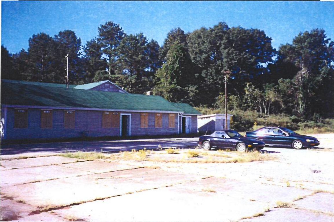
Photo 18. Bath and Locker House – East Face
