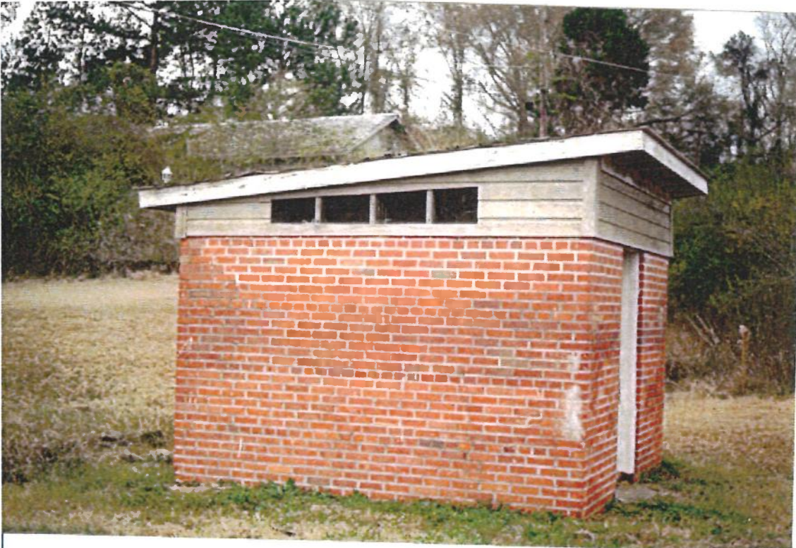
Figure 4: East elevation of structure prior to reconstruction of the wood siding and roof. Pond & Company.
