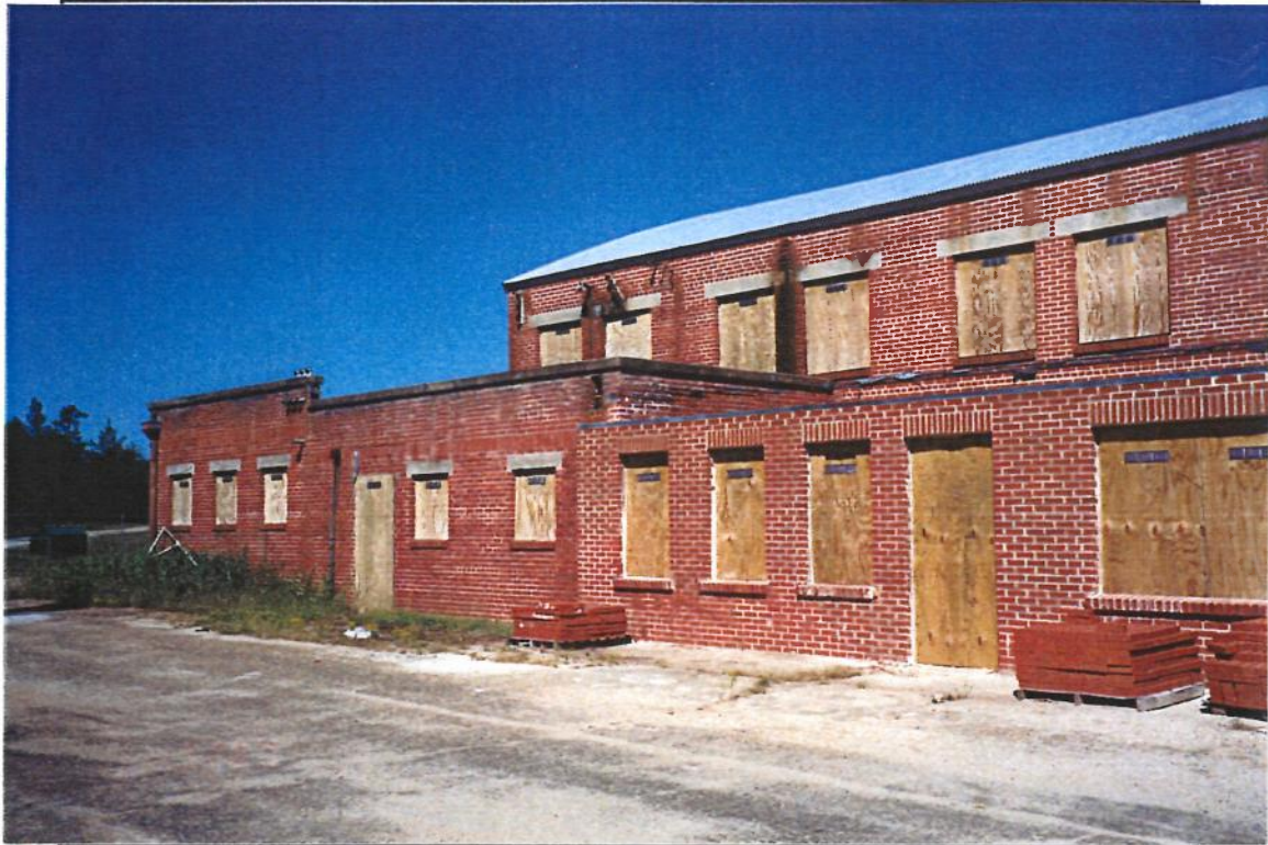
Photo 9. Hangar No. 1 – South Face
