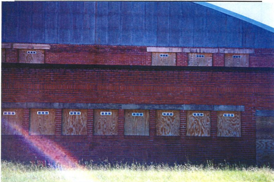
Photo 8. Hangar No. 1 – West Face
