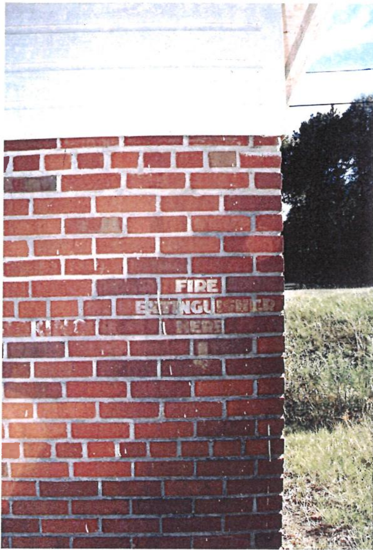
Figure 7: Fire safety indicator on north elevation.
