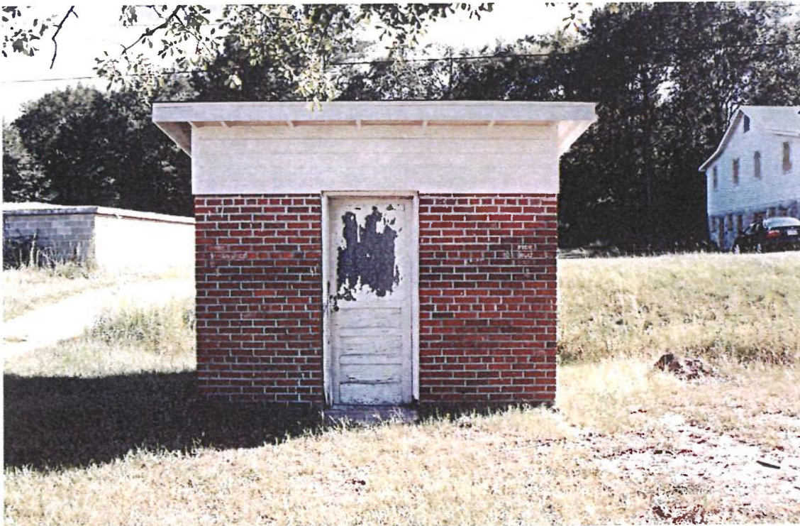
Figure 5: North elevation after reconstruction of wood siding and roof structure.
