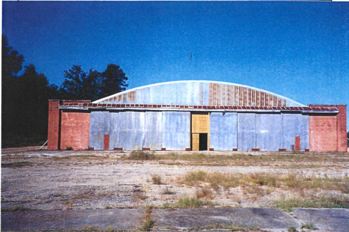
Photo 7. Hangar No. 1 – East Face
