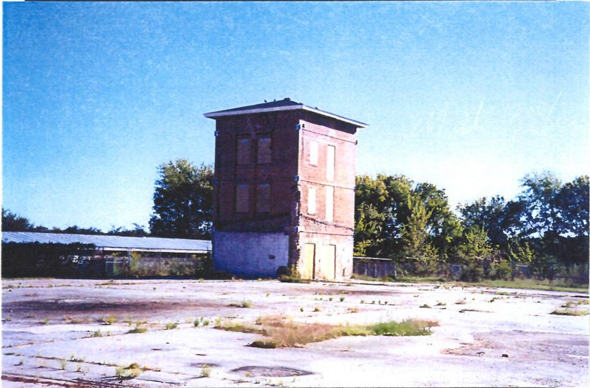
Photo 1. Control Tower Building
