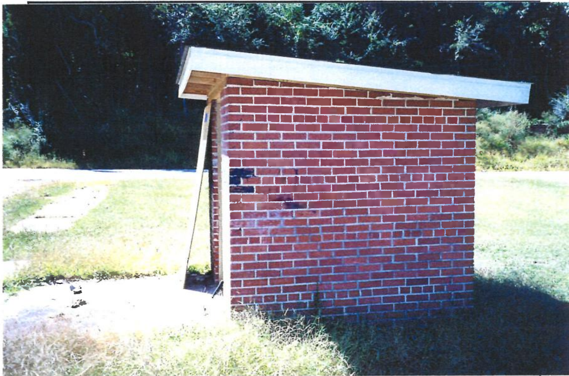
Photo 14. Fire Protection Shed – East Face
