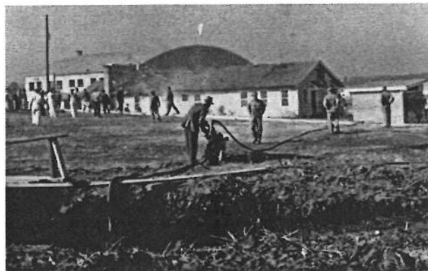
Figure 3: Looking south at the Bath and Locker House. The Dope Storage Shed is on the right. Historic Photograph Collection, Howard University.
