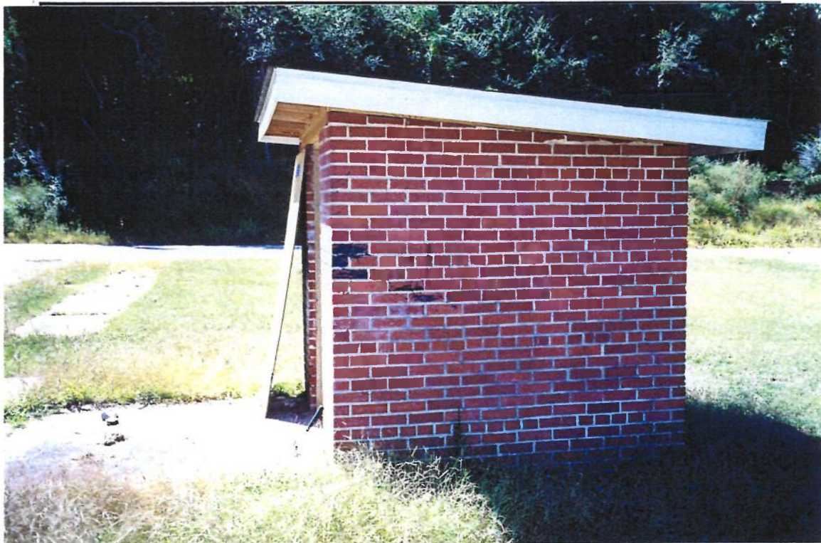
Photo 14. Fire Protection Shed – East Face
