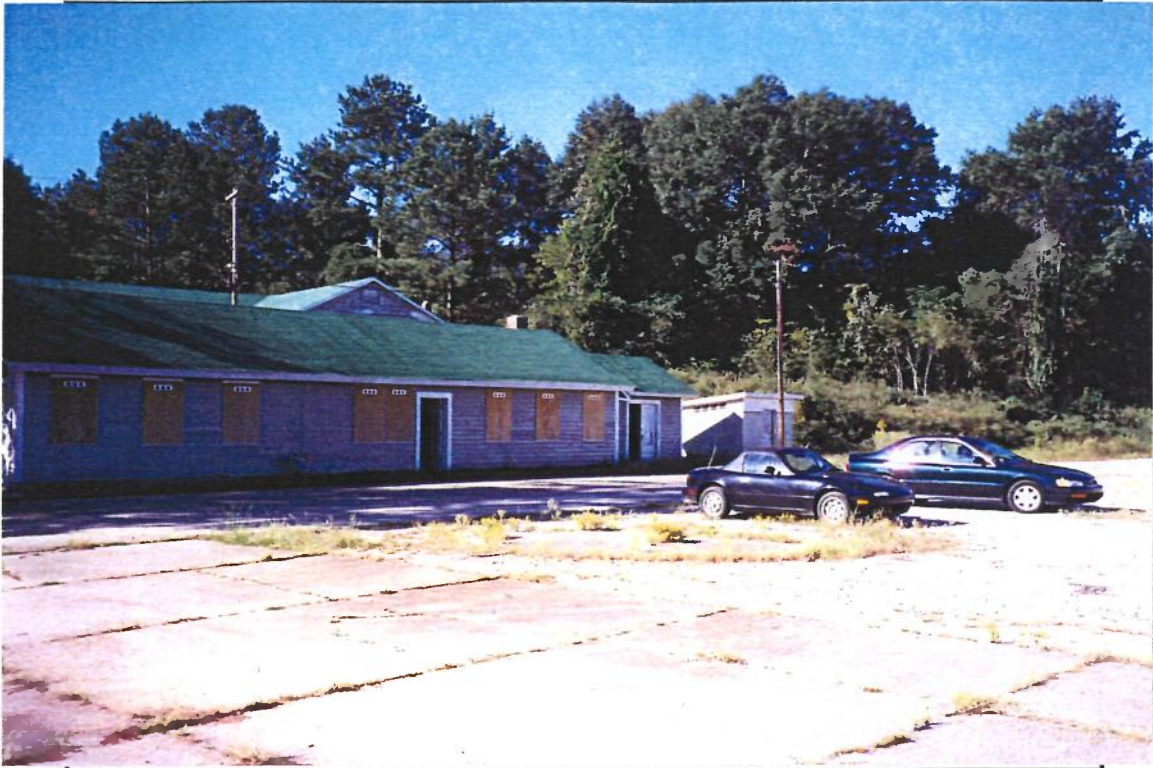
Photo 18. Bath and Locker House – East Face
