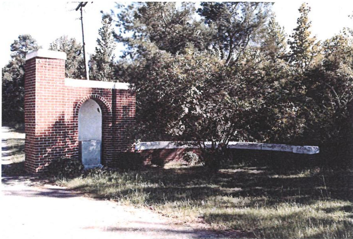
Figure 7: South Wall of Entrance Gate.
