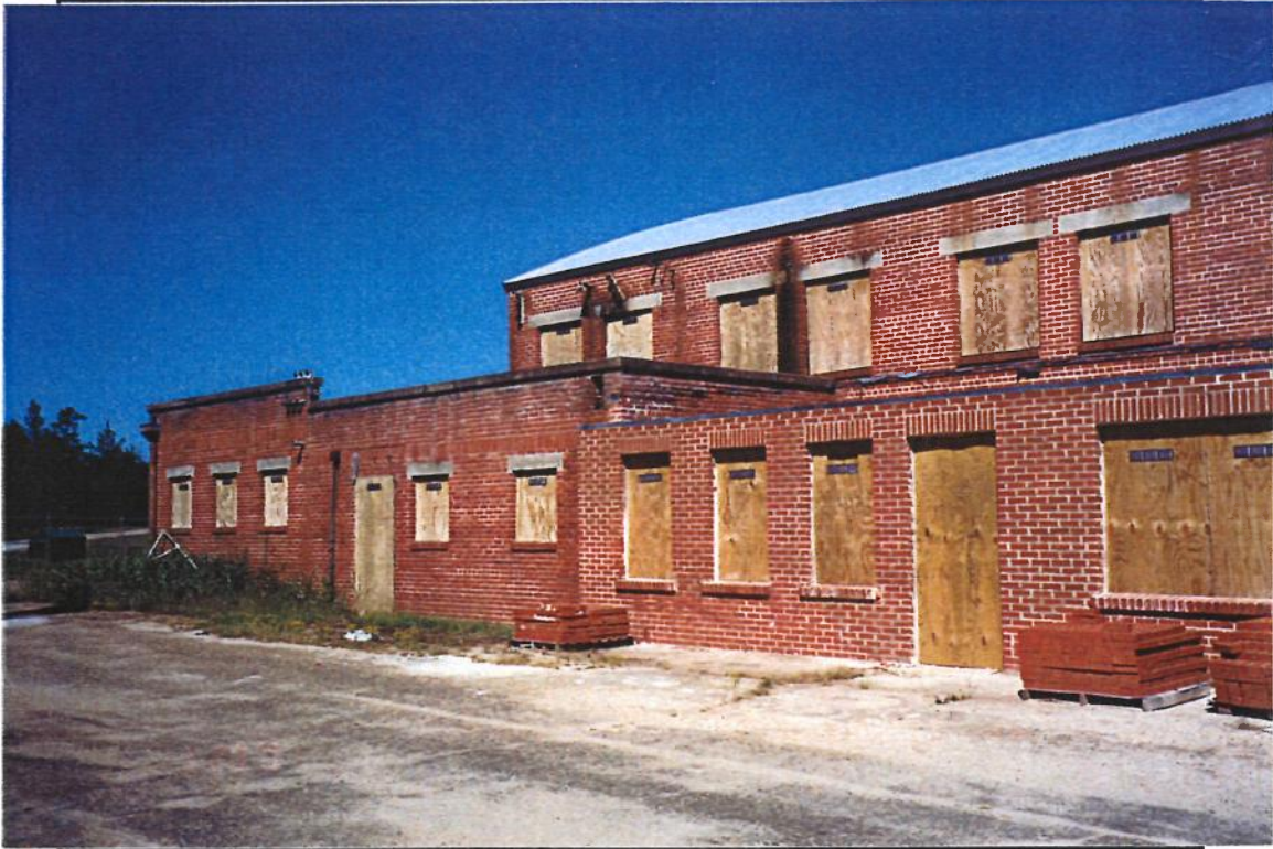
Photo 9. Hangar No. 1 – South Face
