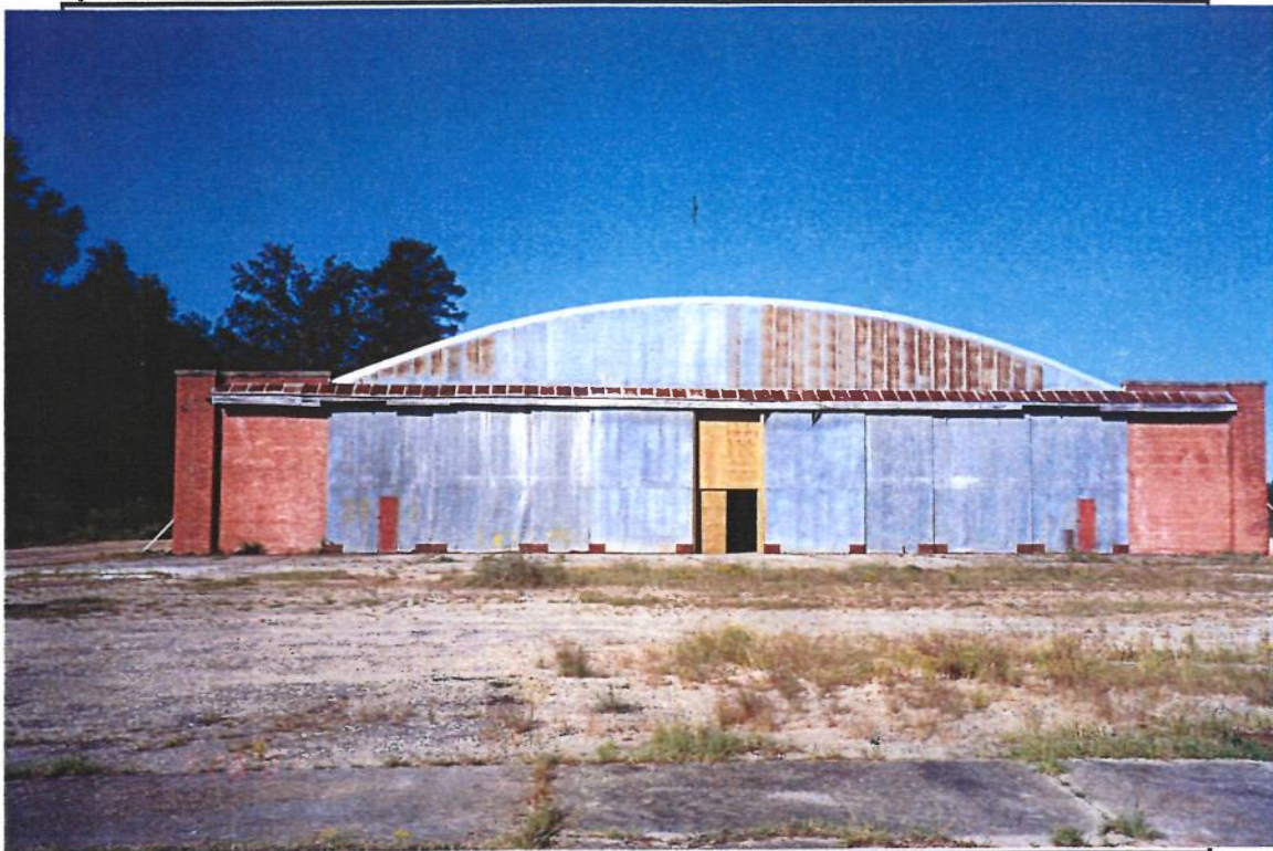
Photo 7. Hangar No. 1 – East Face
