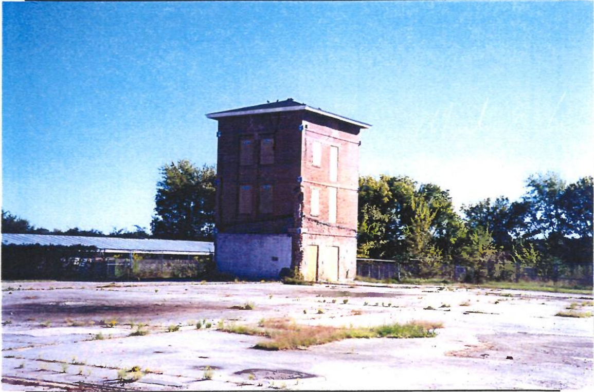
Photo 1. Control Tower Building
