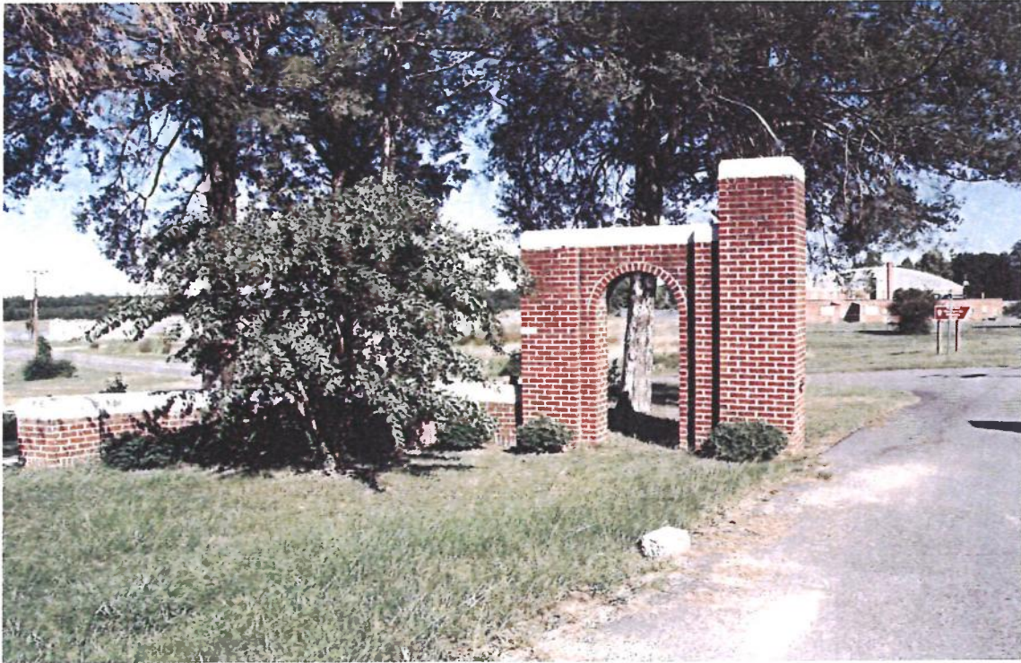
Figure 5: North Wall of Entrance Gate.
