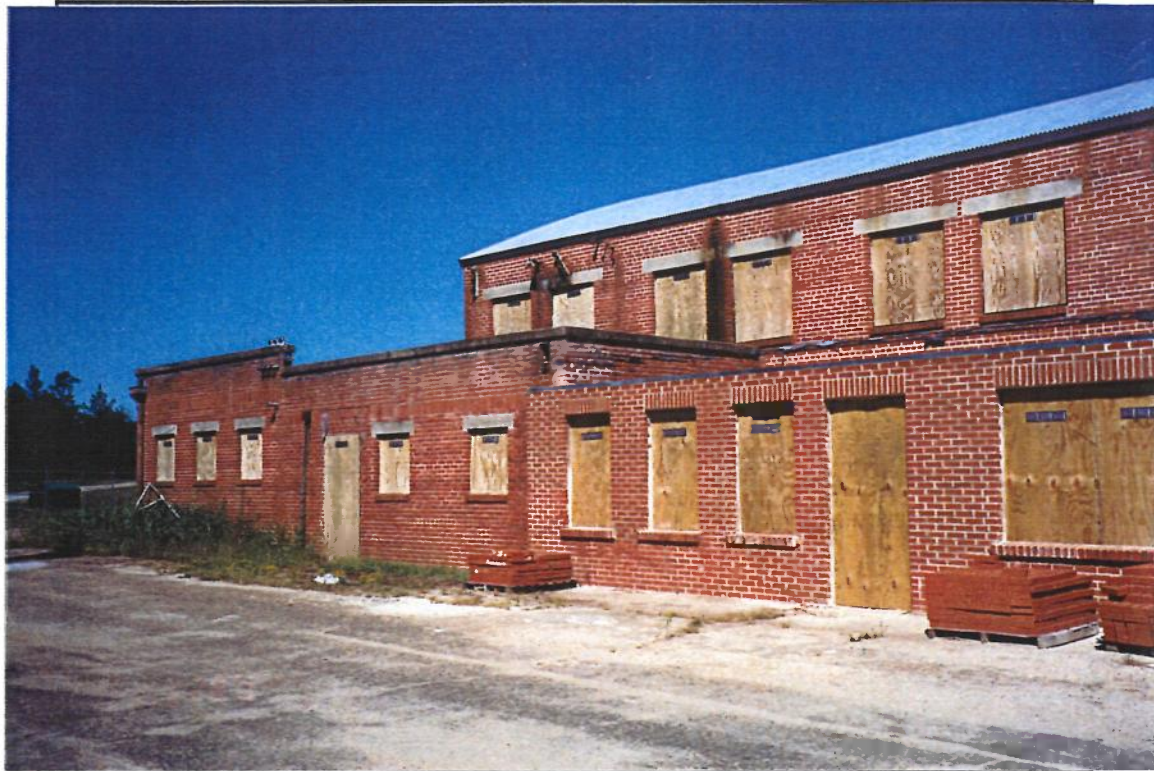
Photo 9. Hangar No. 1 – South Face
