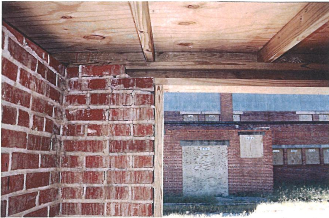
Figure 8: Interior of the Fire Protection Shed.
