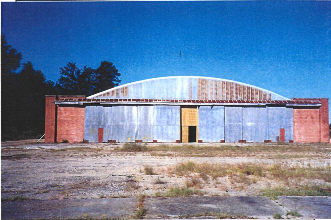
Photo 7. Hangar No. 1 – East Face
