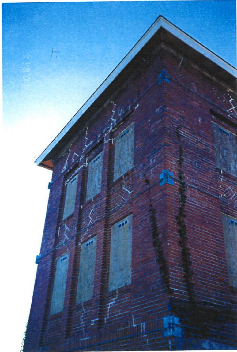
Photo 2. Control Tower Building – West Face
