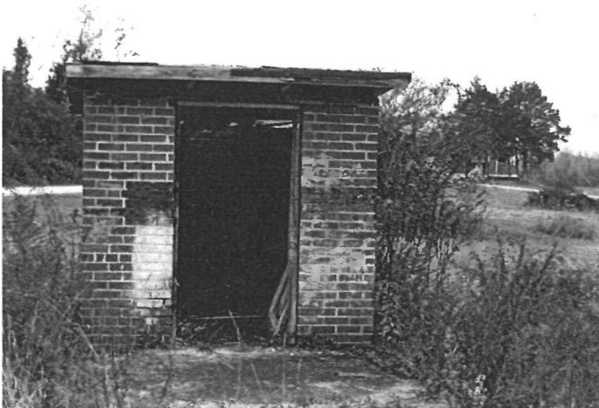
Figure 5: Fire Protection Shed in 1997 prior to stabilization. National Park Service, SERO, Atlanta, Georgia.
