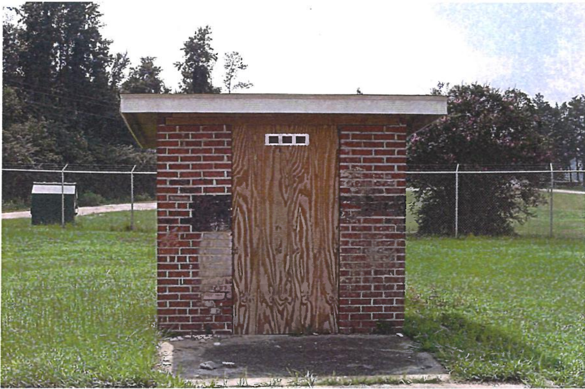
Figure 6: East elevation of the Fire Protection Shed in the fall of 2001 after stabilization.
