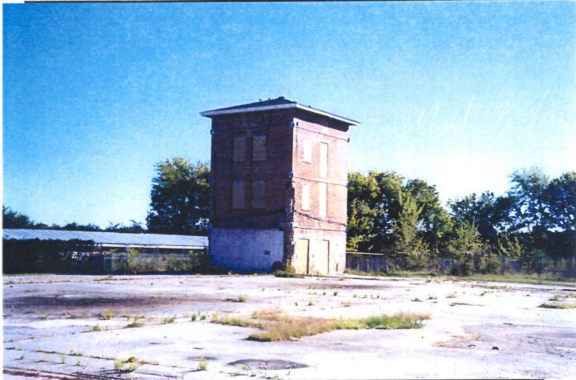
Photo 1. Control Tower Building
