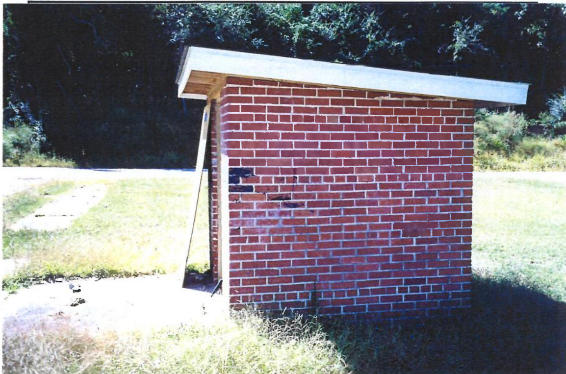
Photo 14. Fire Protection Shed – East Face
