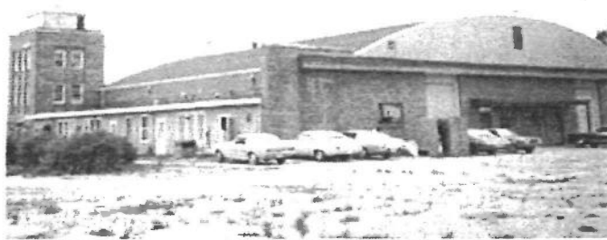
Figure 9: 1977 photograph of Hangar Number Two showing alterations made by the Tuskegee University Veterinary School. Booker Conley's Files, Physical Plant, Tuskegee University.
