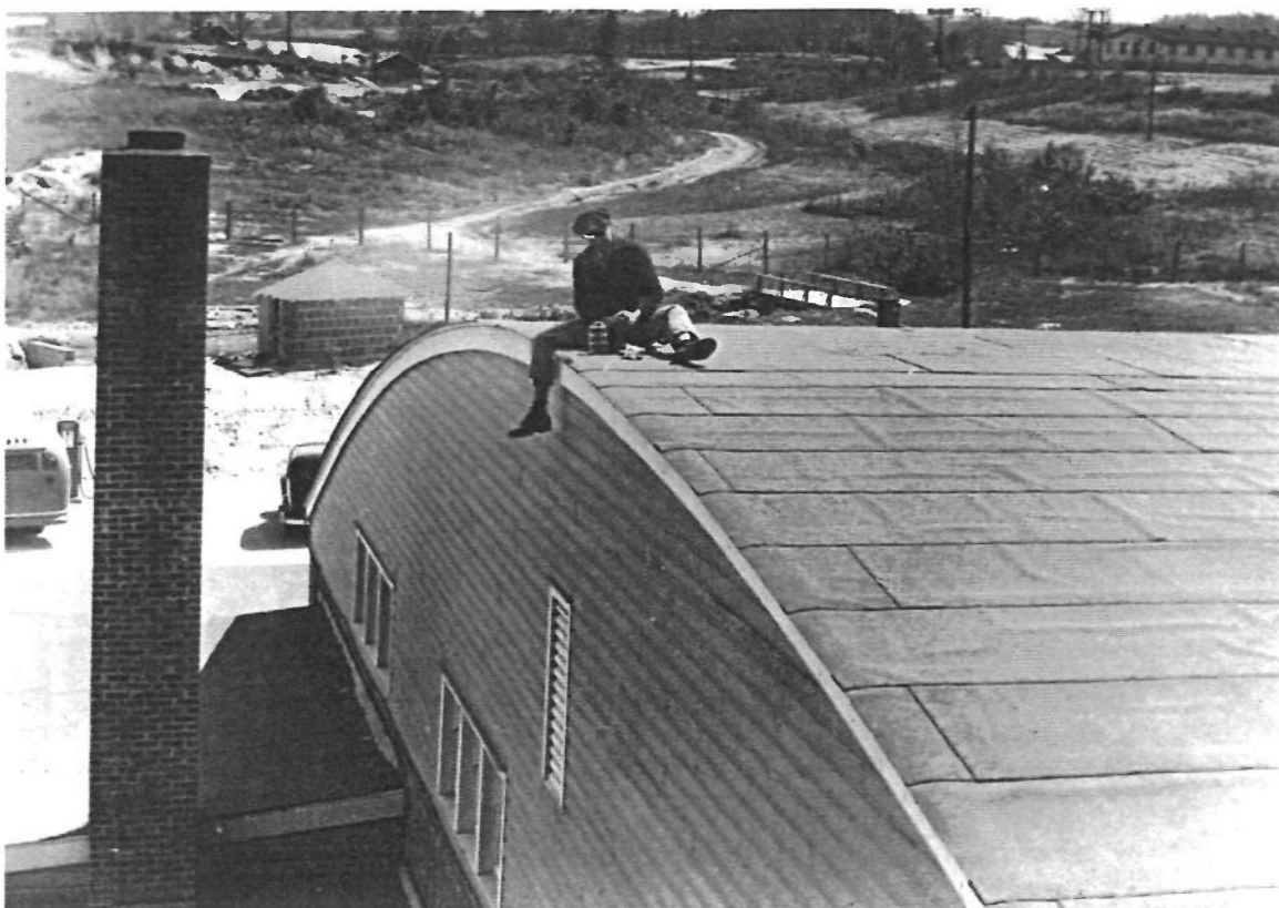
Figure 7: Historic photograph documenting the roof of Hangar Number Two. Historic Photograph Collection, Howard University.
