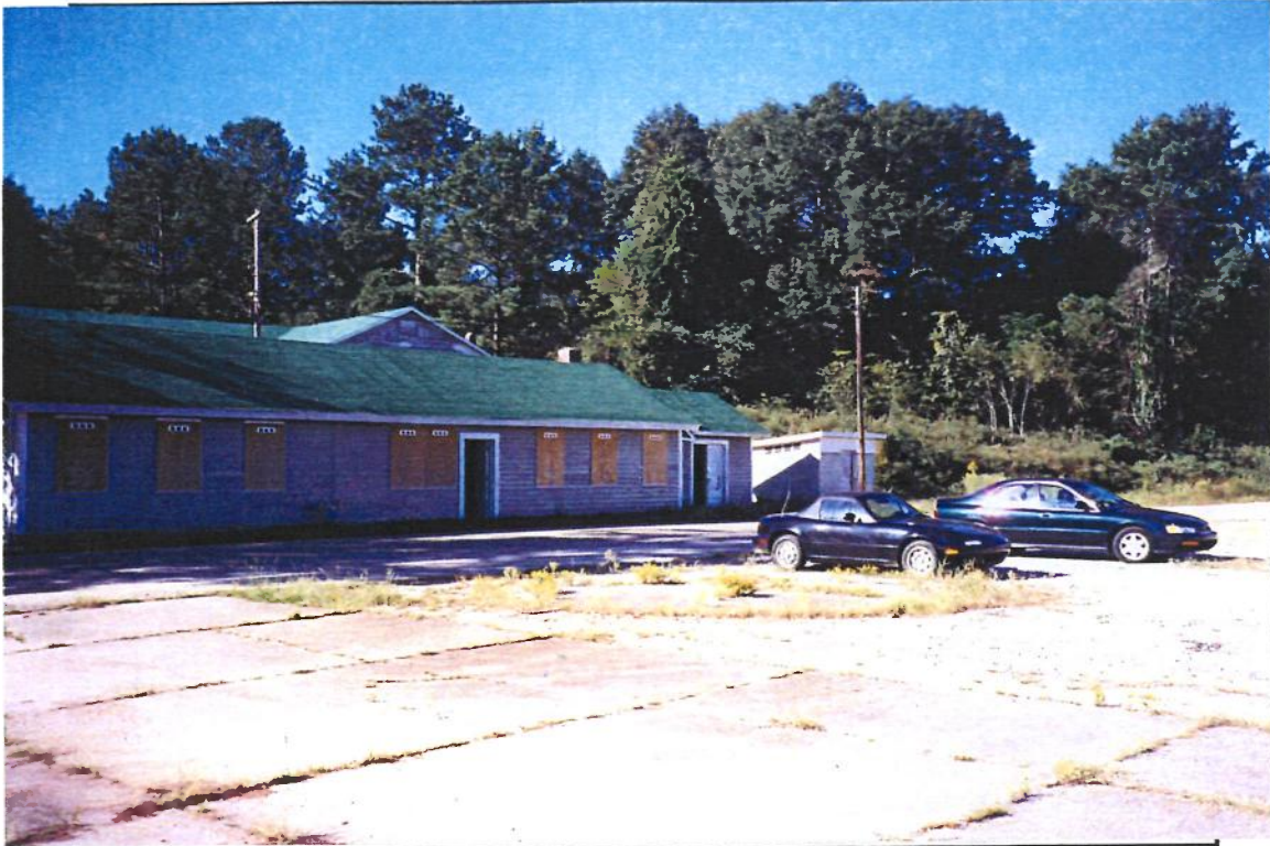
Photo 18. Bath and Locker House – East Face
