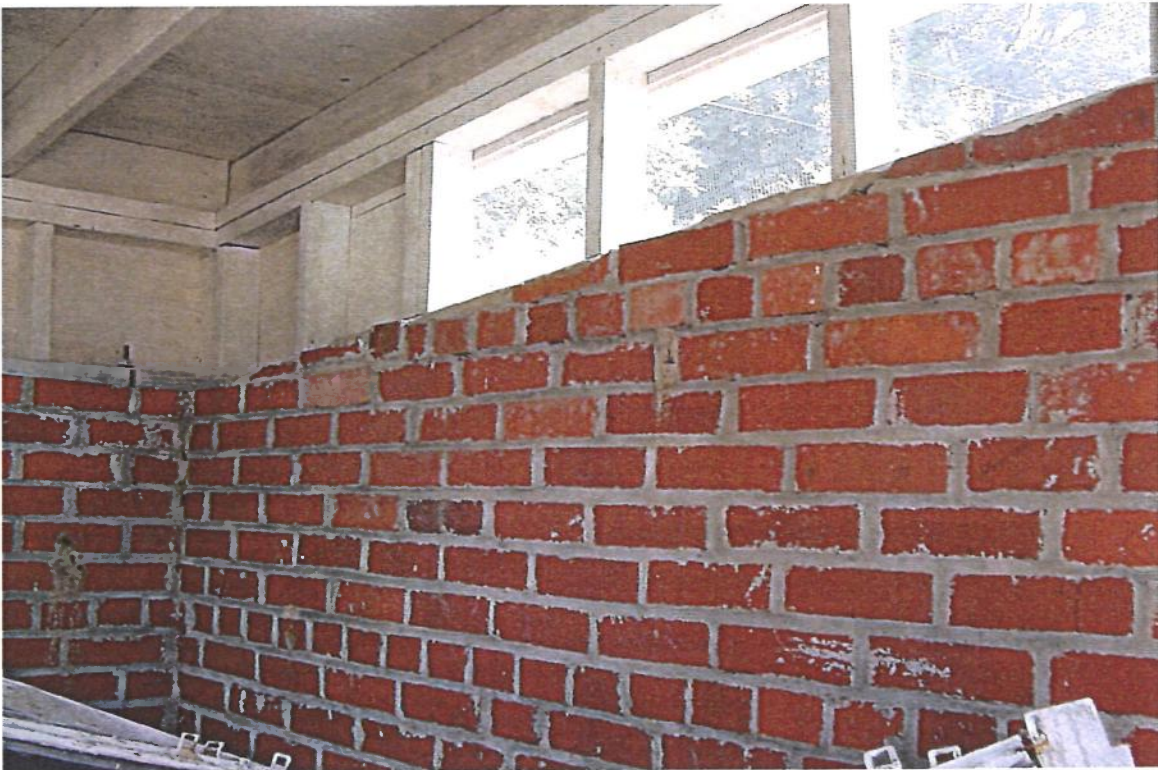
Figure 8: Unpainted interior of the Oil Storage Shed.
