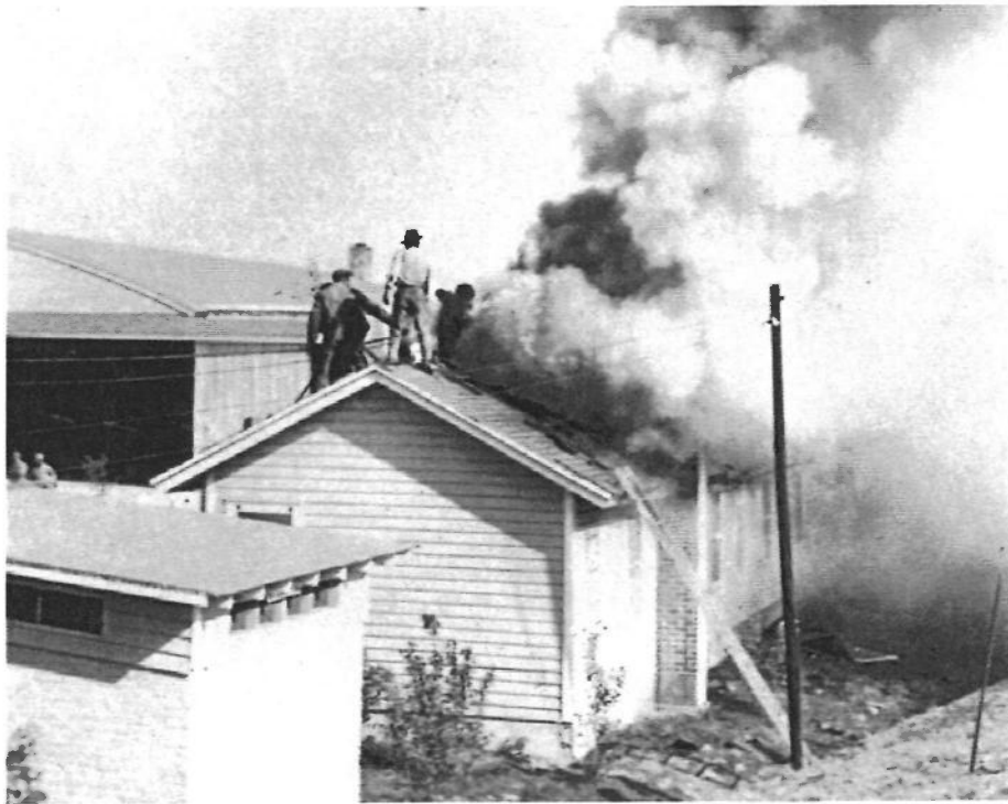
Figure 9: Historic photograph of exposed rafter tails on south elevation of the Oil Storage Shed. Historic Photograph Collection, Howard University.
