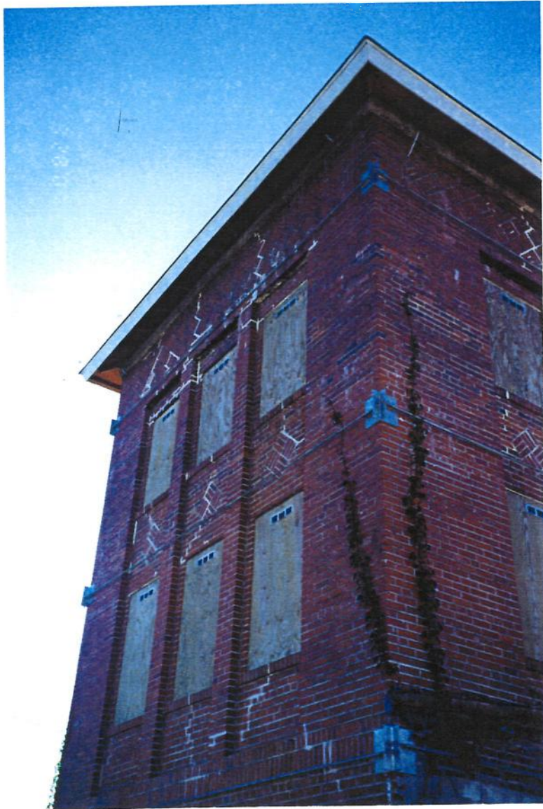
Photo 2. Control Tower Building – West Face
