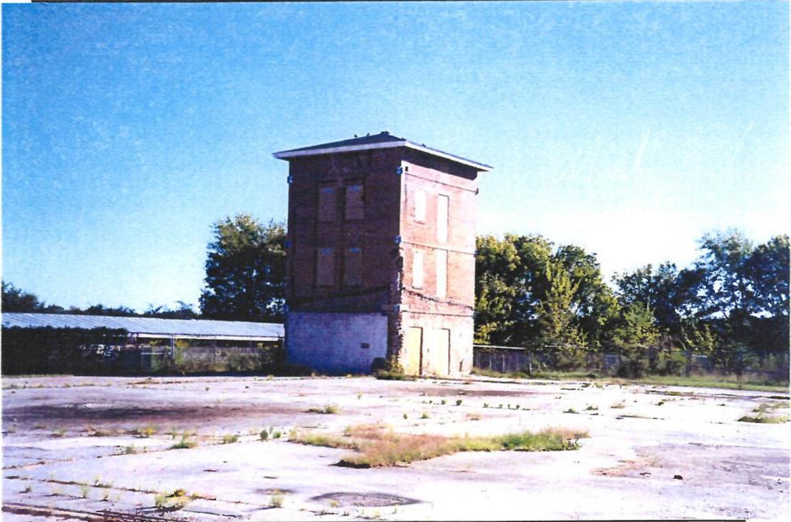
Photo 1. Control Tower Building
