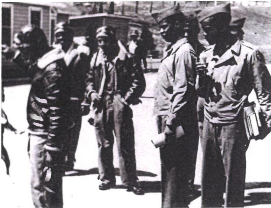
Figure 3: The Oil Storage Shed can be seen in the background of this May 1944 photo. AFHRA, Maxwell AFB.
