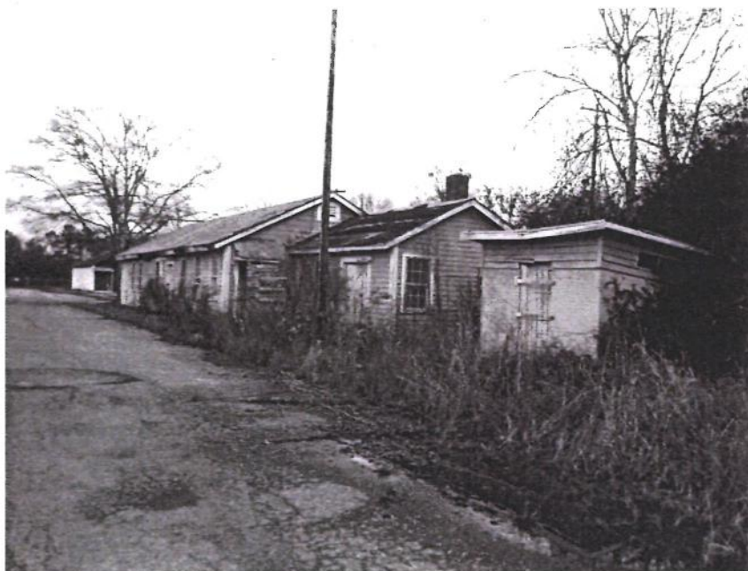
Figure 5: 1997 view from the west of the structure showing signs of roof deterioration. National Park Service, SERO, Atlanta, Georgia.
