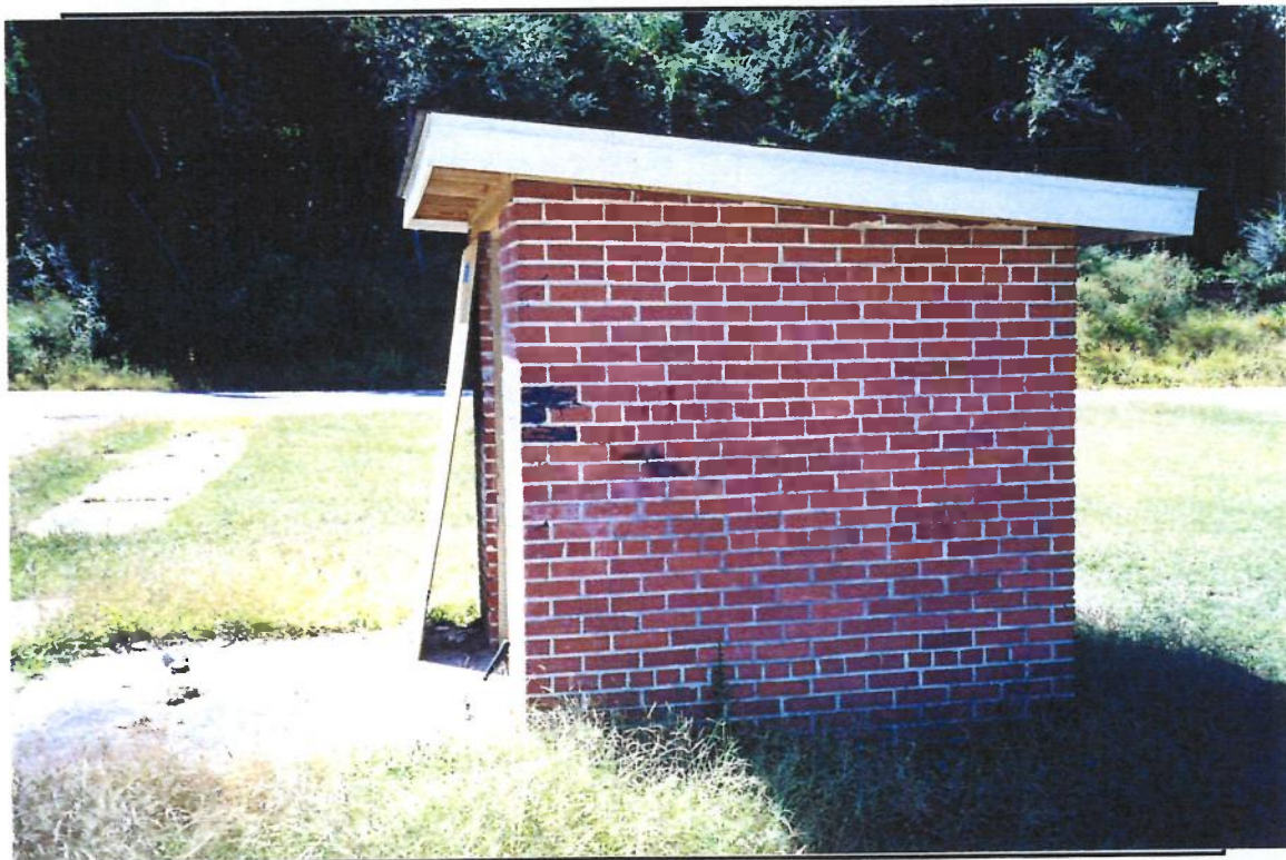
Photo 14. Fire Protection Shed – East Face
