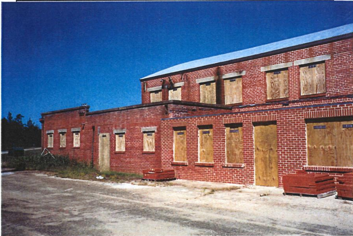
Photo 9. Hangar No. 1 – South Face
