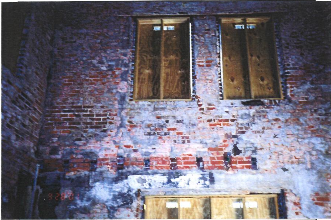
Photo 3. Control Tower Building – Interior North Face
