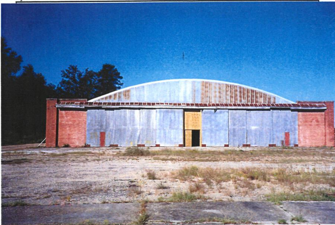
Photo 7. Hangar No. 1 – East Face
