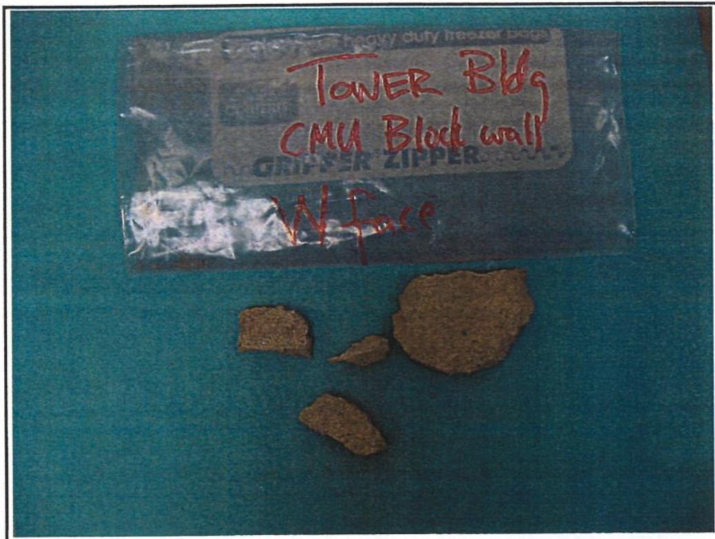
Photo 5. Mortar samples from Control Tower – exterior west face of building
