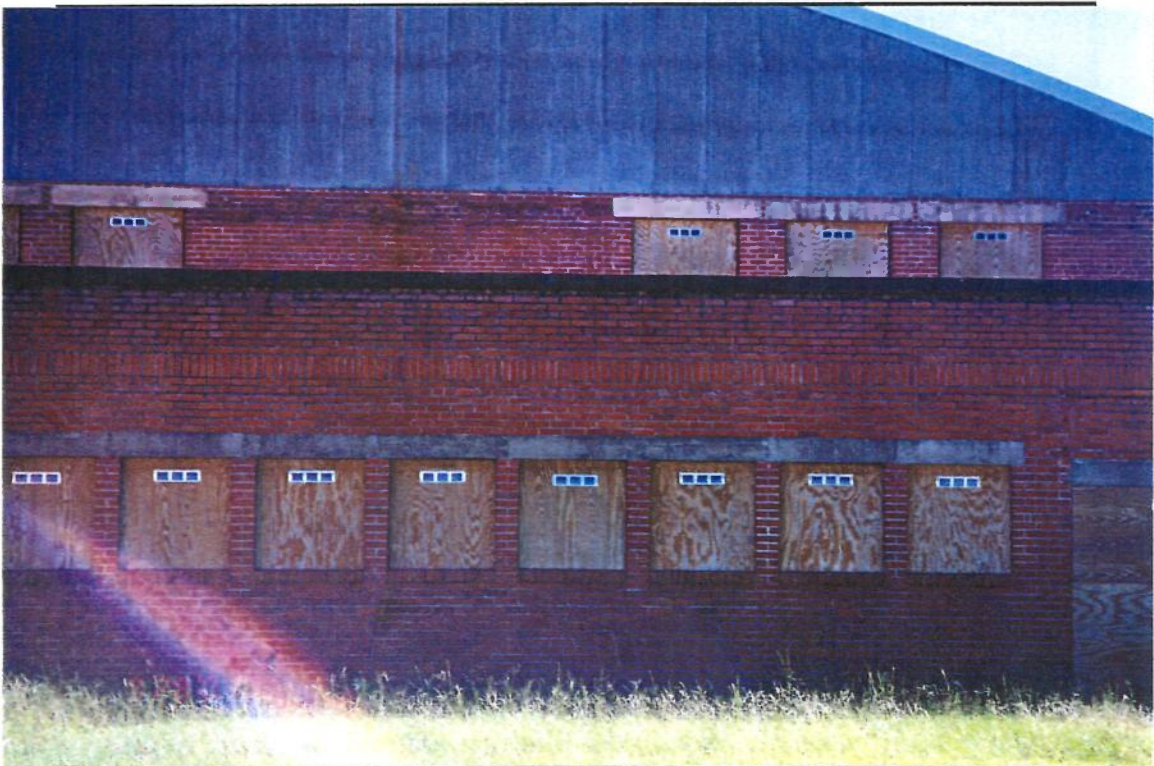
Photo 8. Hangar No. 1 – West Face
