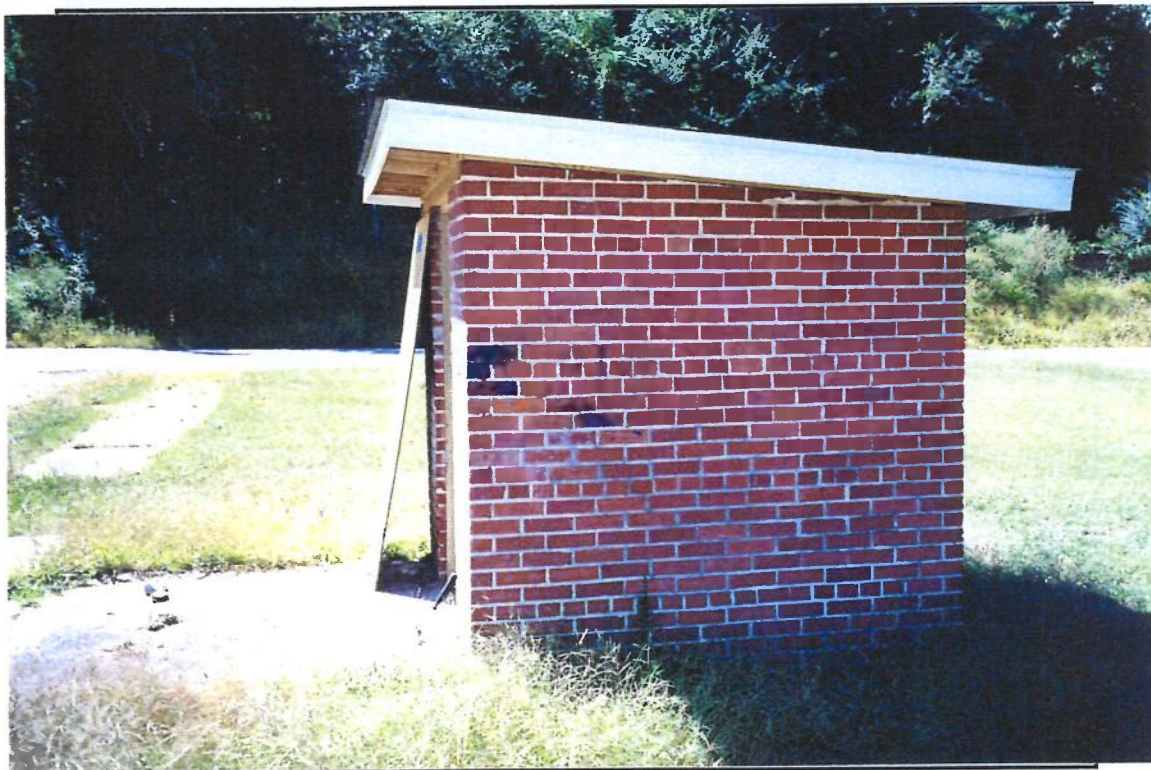
Photo 14. Fire Protection Shed – East Face
