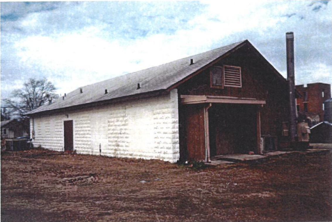
Figure 6: Looking northwest at the Warehouse/Vehicle Storage Building. Pond & Company.
