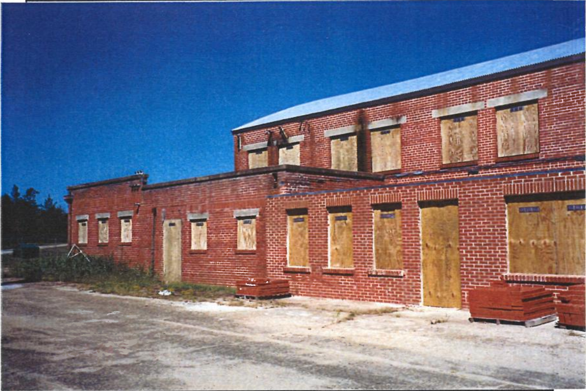
Photo 9. Hangar No. 1 – South Face
