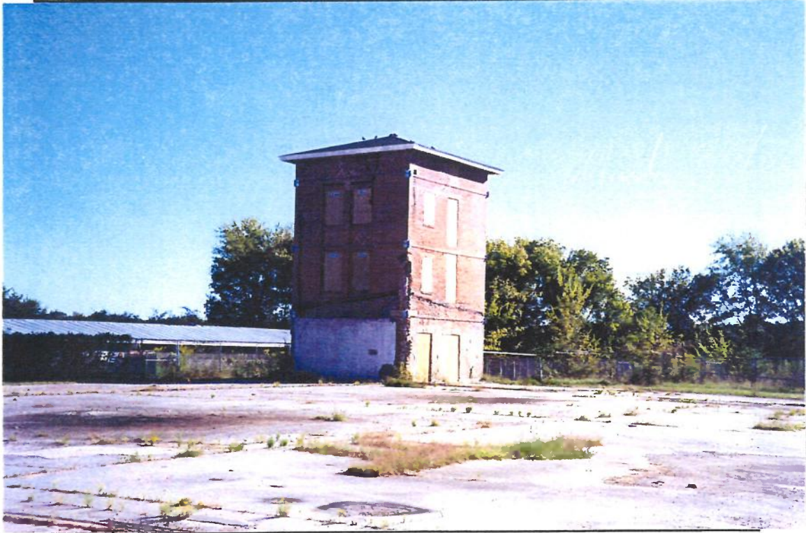
Photo 1. Control Tower Building
