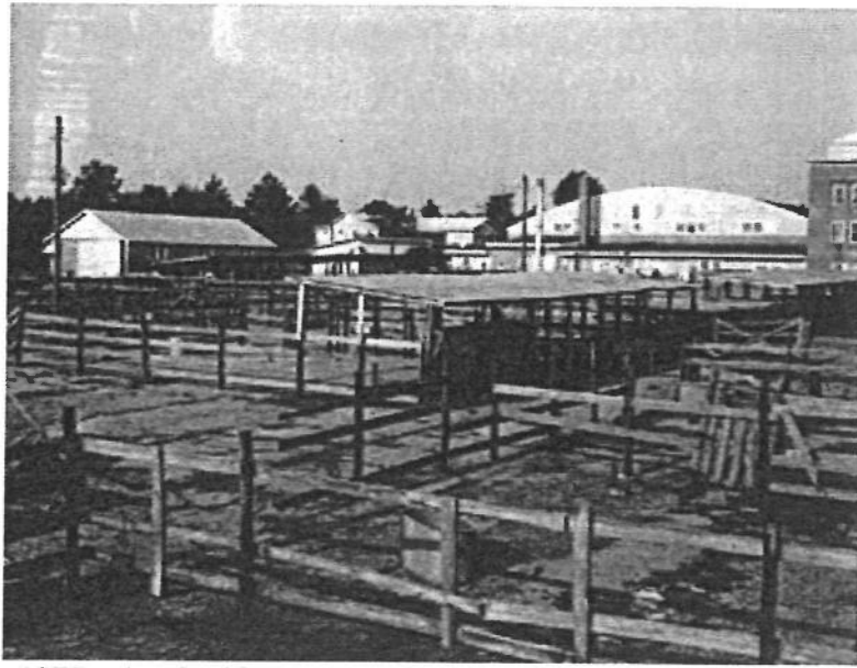
Figure 4: Early 1970s view looking west at the rear of Hangar Number Two. The Warehouse/Vehicle Storage Building, at the left of the photograph, has not yet been renovated by the Veterinary School. Booker Conley's Files, Physical Plant, Tuskegee University.
