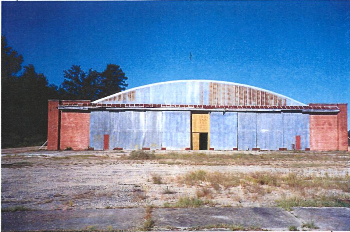
Photo 7. Hangar No. 1 – East Face
