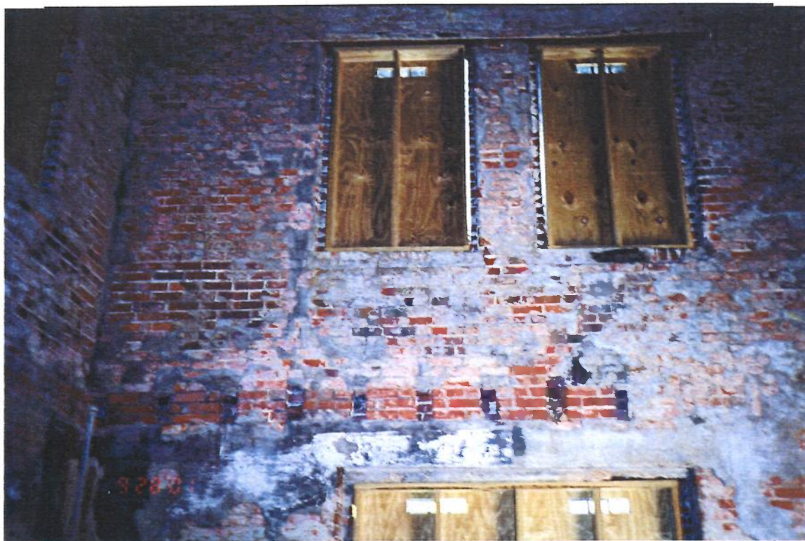
Photo 3. Control Tower Building – Interior North Face
