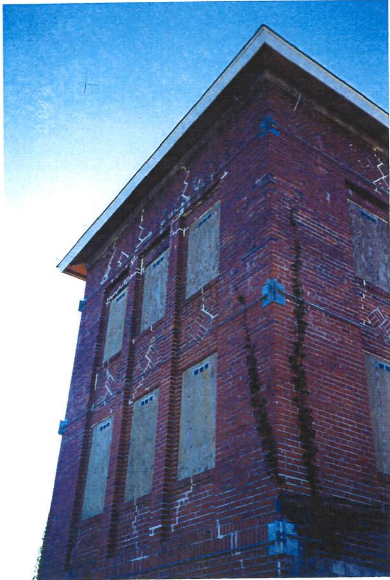
Photo 2. Control Tower Building – West Face
