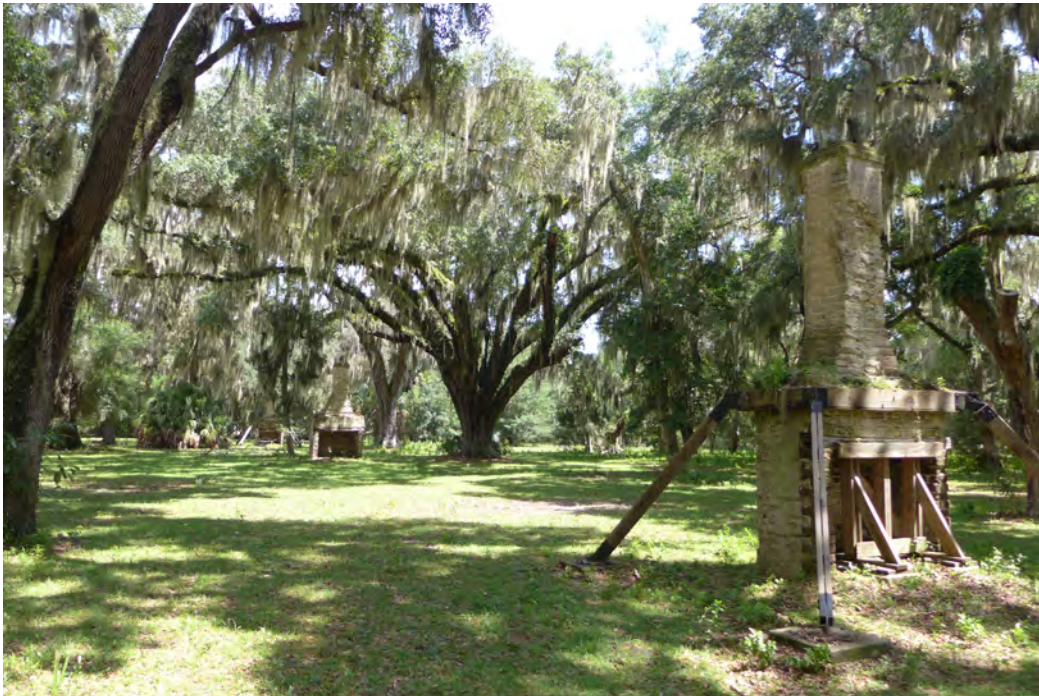
Image 2. General setting of the majority of the chimneys, located in a shaded tree grove in approximately the middle of the island. Some chimneys were previously stabilized in 2008.
