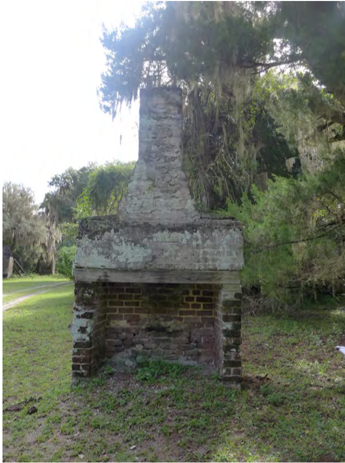
Image 1. Typical intact chimney with replaced wood lintel. Note the use of red brick for the hearth and firebox and the use of tabby brick elsewhere.
