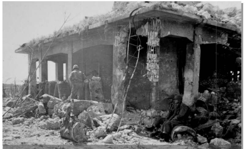
Figure 24. The Japanese Airfield Operations Center, with heavy damage to the west wall.
