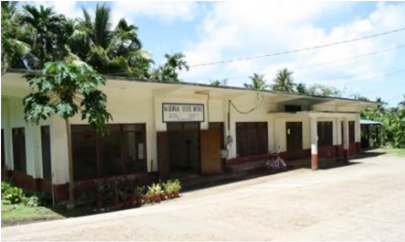
Figure 5. Ngardmau Government State office and community center located in Ngardmau State. (Photo taken by BAC/HPO during 2010 survey of the states of Palau)
