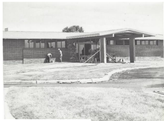
Figure 7. Visitor Center under construction
