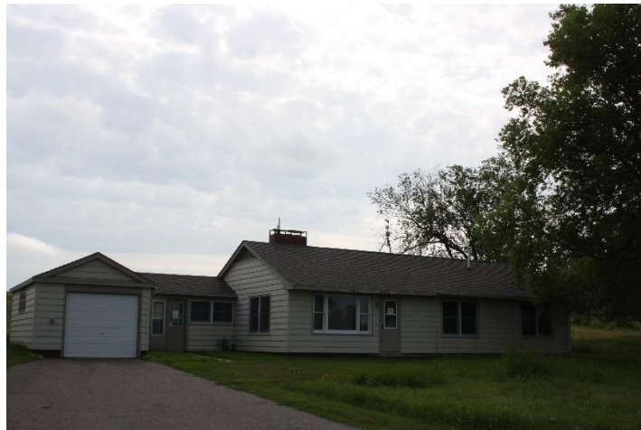
Figure 37. West façade of Residence 1. August 2020.
