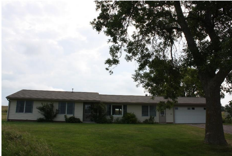
Figure 45. West façade of residence 2. August 2020.
