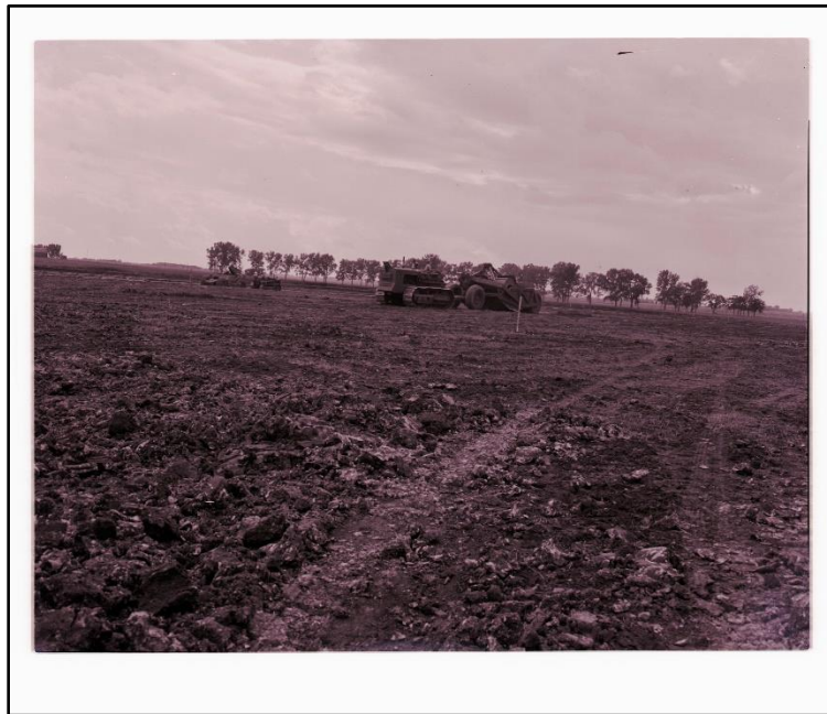
Figure 6. Ground clearing in preparation for construction of Visitor Center and road Photo courtesy Pipestone County Historical Society.
