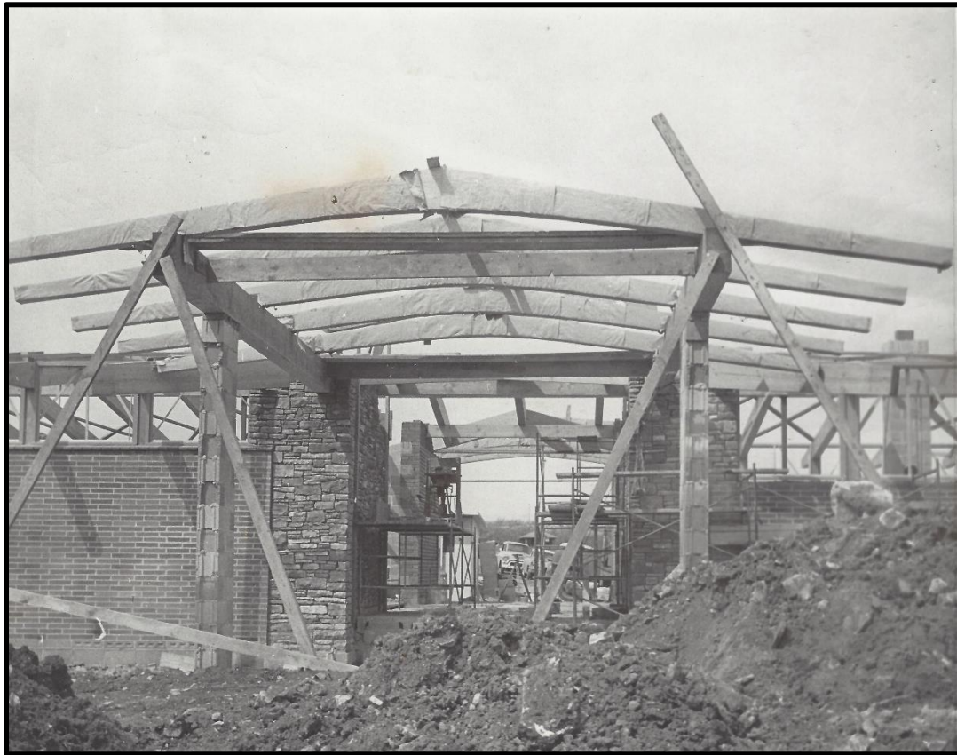
Figure 21. Stonework and brick walls up while roof under construction. View through Visitor Center is notable. Photo courtesy Pipestone County Historical Society.
