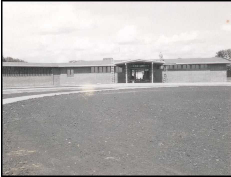
Figure 19. Visitor Center nearing completion. Photo courtesy Pipestone County Historical Society.
