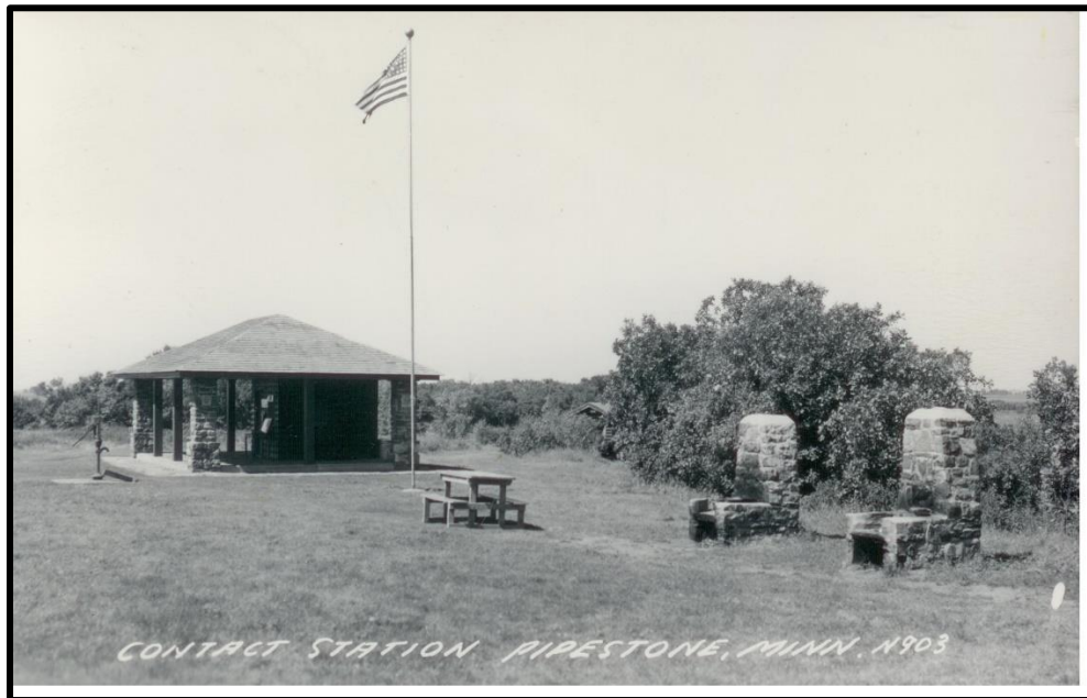
Figure 4. CCC-ID Picnic shelter and fire pits. Photo courtesy NPS digital gallery.
