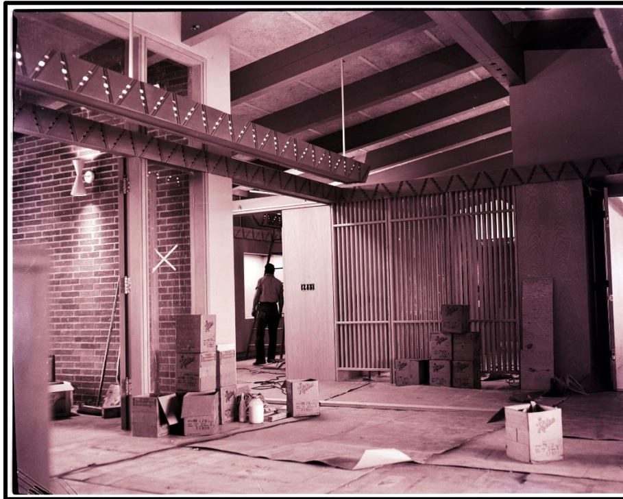
Figure 23. Visitor Center interior under construction.
