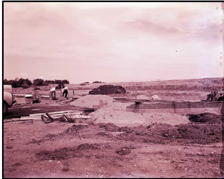
Figure 17. Visitor Center under construction, with concrete foundation laid and brick walls just beginning to rise. The image shows how the long, low, single-story design evokes the distant horizon line of the northern plains. Photo courtesy Pipestone County Historical Society.
