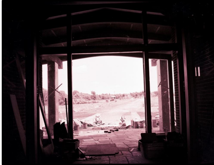
Figure 15. Visitor Center under construction showing the view from the Visitor Center toward the trail, a significant part of the design. Photo courtesy Pipestone County Historical Society.
