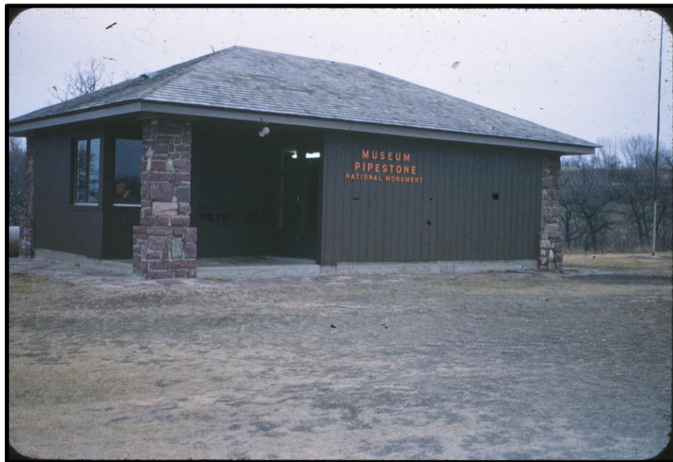
Figure 5. Pipestone Visitor Center and Museum prior to Mission 66 Era. Photo courtesy NPS digital gallery.
