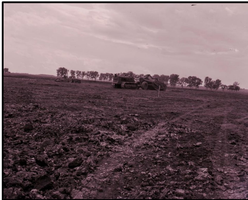
Figure 16. Earth moving equipment preparing the site for construction in the area of the access road and parking lot. Trees and viewshed noticeable in the background. Photo courtesy Pipestone County Historical Society.
