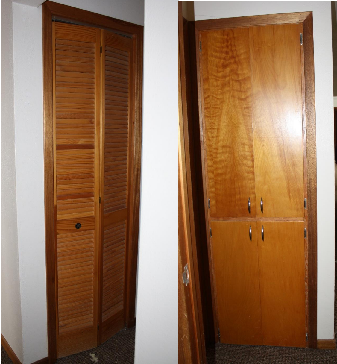
Figure 48. North and south louvered bi-fold closet and paired cabinet doors at bathroom in north residence. November 2019.
