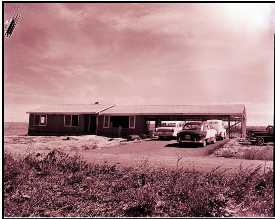
Figure 25. Residence HS-6 under construction in 1958.
