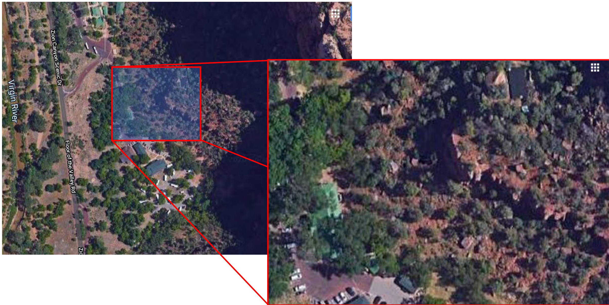
Figure A-4: Route 0412 Concessionaire/ Dorm Access Road near Zion Lodge, Locations of Evaluated Unstable Slopes; Site 1234 (Google Earth, 2020).
