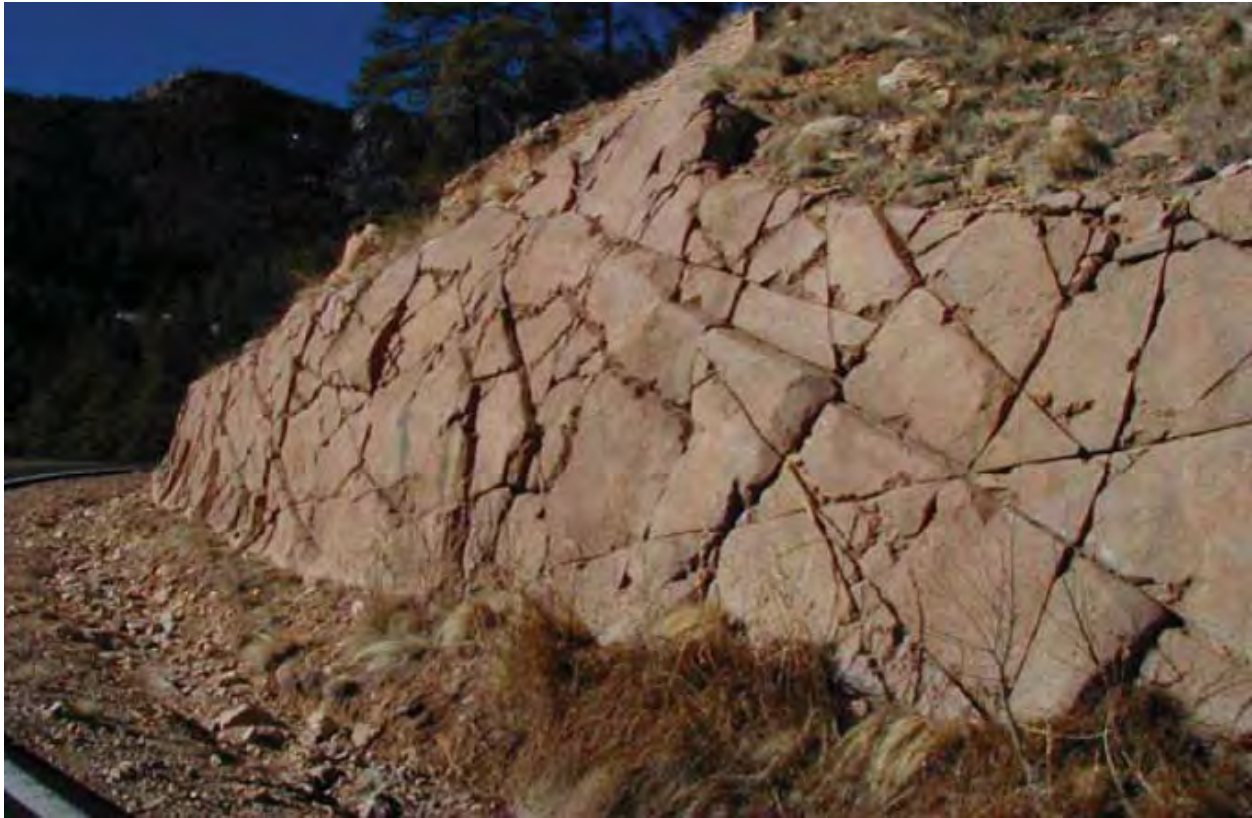
Figure 4-5 Example of Sculpted and Colored Shotcrete (Yosemite National Park, from CFLHD).
