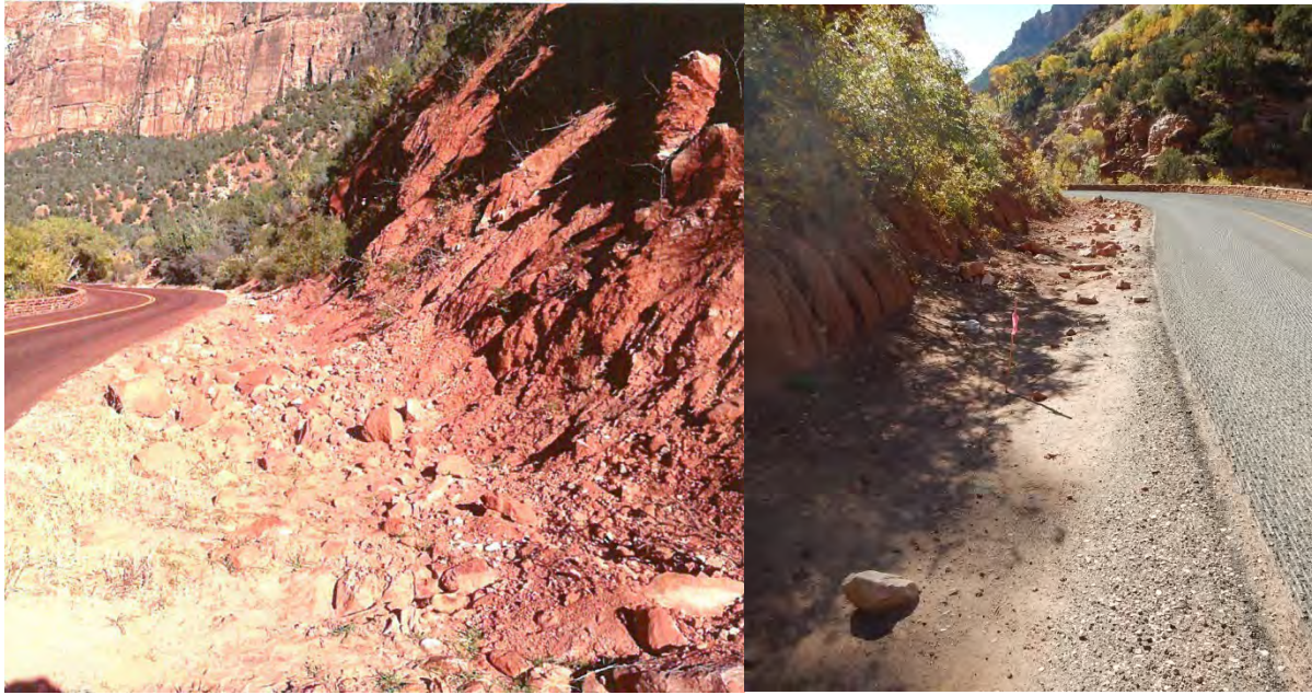
Figure 2-6 Ditch Before (left) and Recently After (right) Cleaning at Site 1222.
