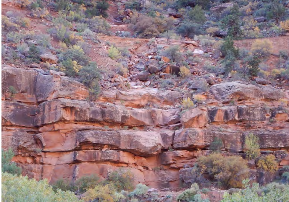
Photograph 1004-A: Drainage 1 from switchback culvert outlet at top of cutslope from upper switchback retaining wall. Recommended hardened basin for easier debris cleanout and reduction of undercutting erosion at the base of the slope.
