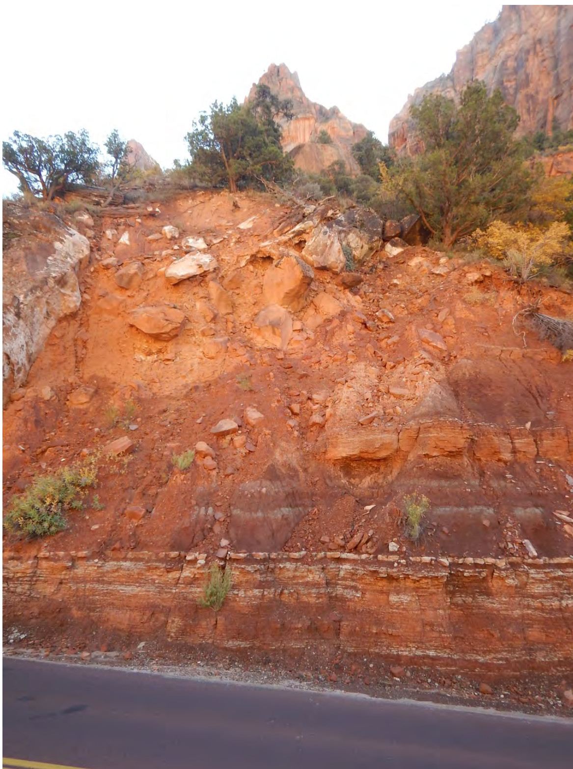
Figure 2-3 Representative Zion-Mt. Carmel Highway Switchbacks where Block-in-Matrix Colluvium is above Thinly Interbedded Siltstone, Mudstone, and Sandstone Prone to Differential Erosion.
