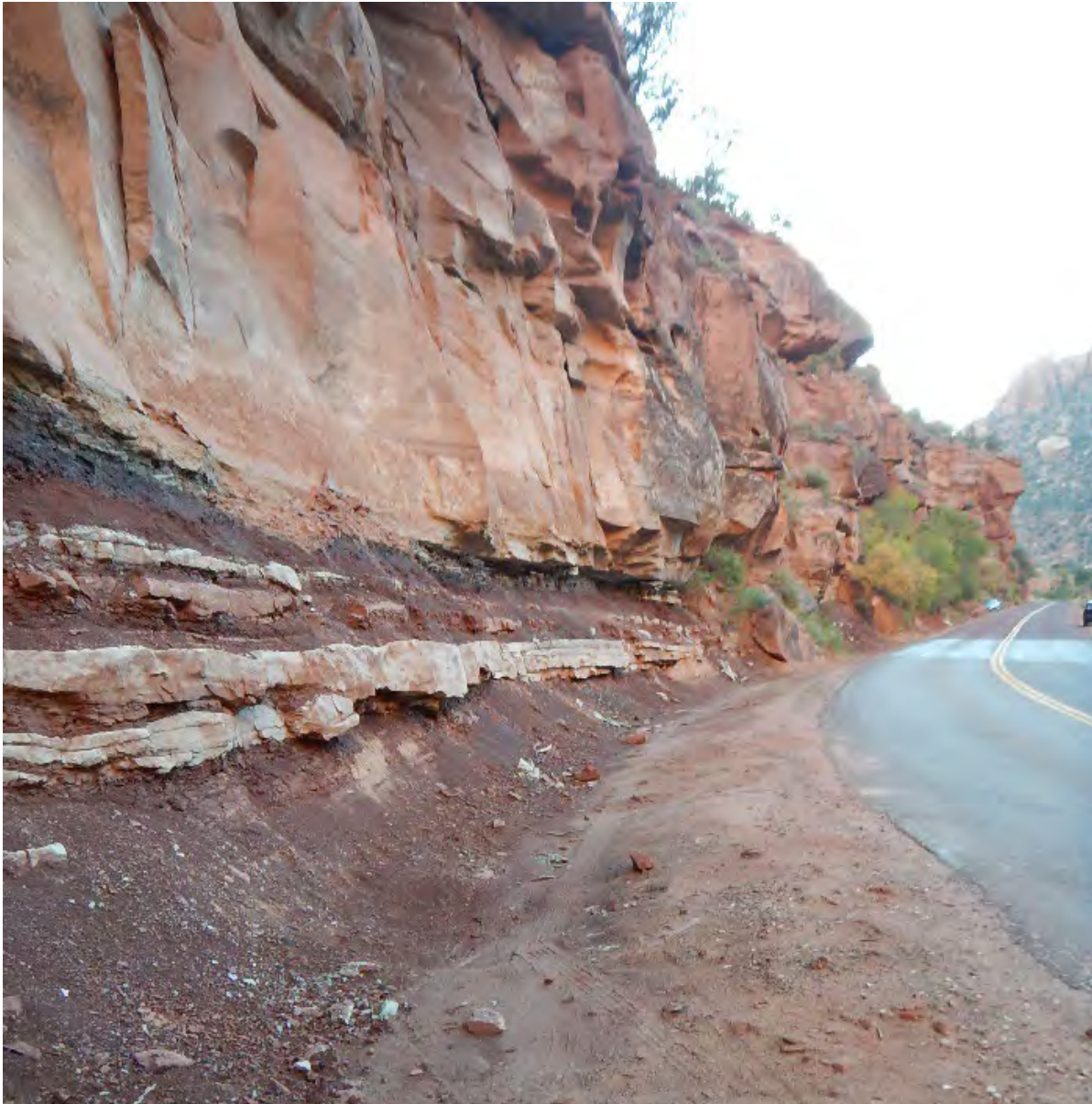
Figure 2-2 Representative Zion-Mt. Carmel Highway Switchbacks with Bedrock Differential Erosion and Rockfall Debris in Unpaved Ditches.
