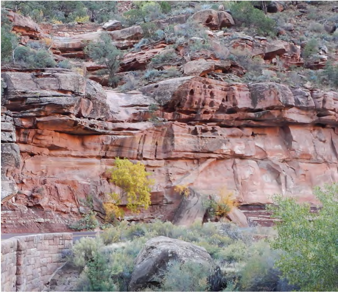
Photograph 1002A: Scaling would include cleanout of the drainage channel at the top of the cut slope and the dry-stacked retaining wall (check dam) at the top of the slope.
