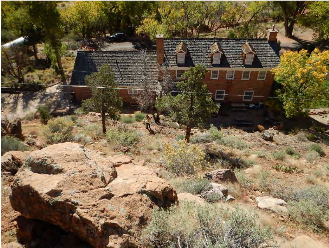
Figure 2-9 View Above the Sandstone Boulder Looking Down at the Residence at Site 1431.
