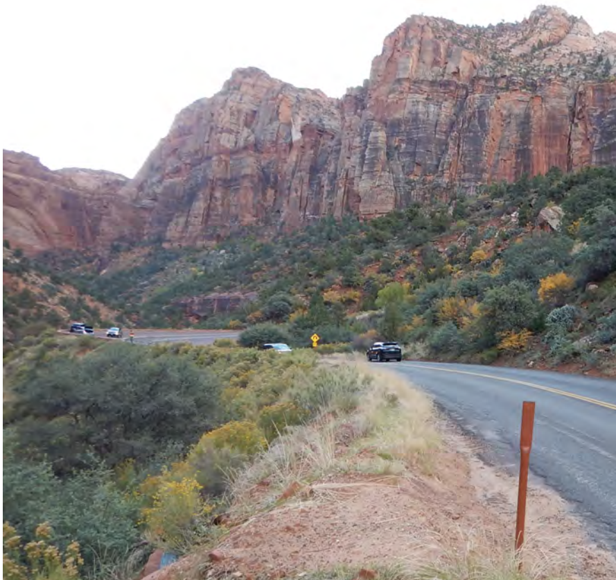
Figure 5104B: Photograph of Carl's Bend in large landslide complex.
