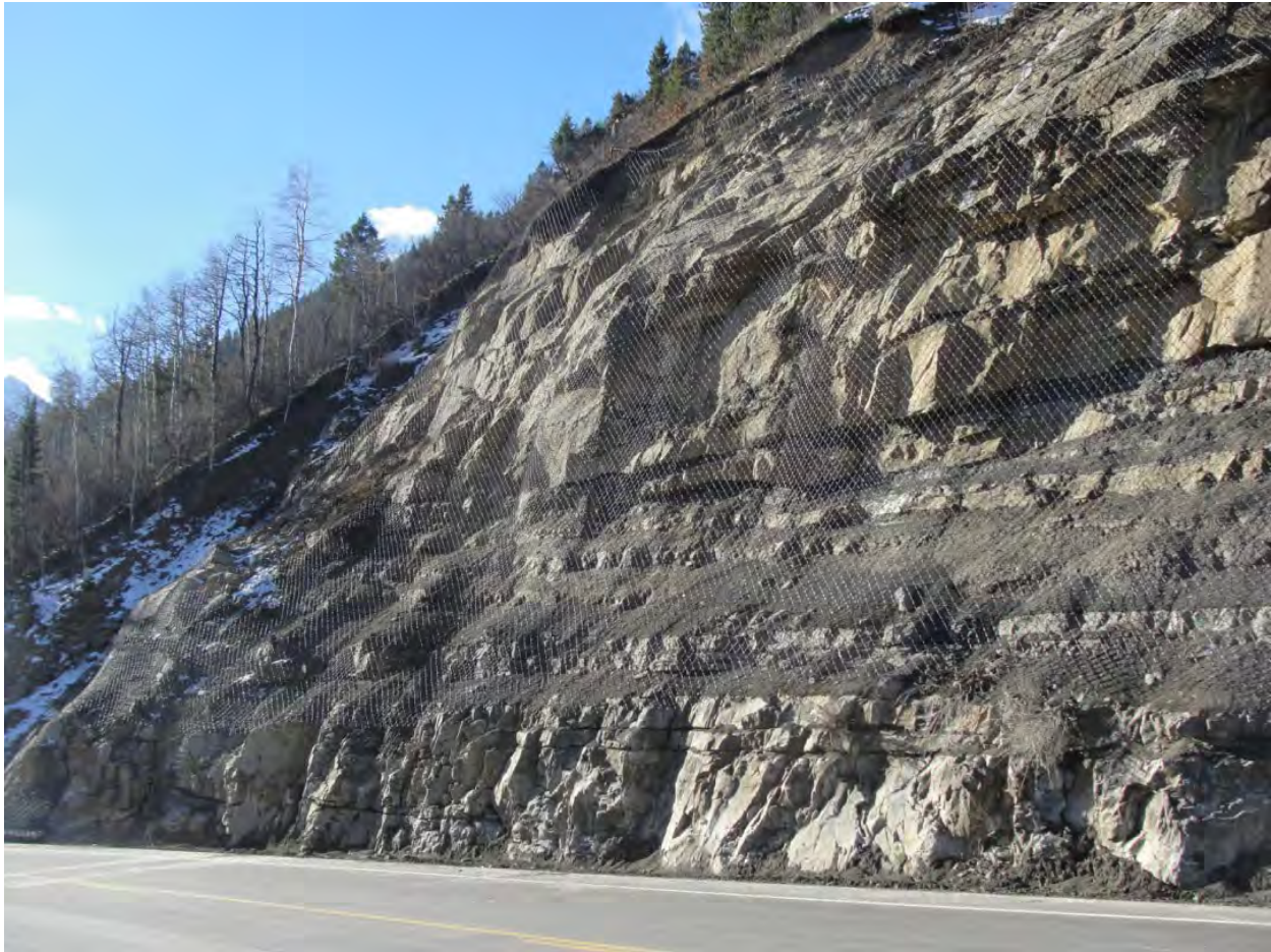
Figure 4-9 Example of Draped Mesh Rock Cut with Differential Weathering (from Arndt, 2016).
