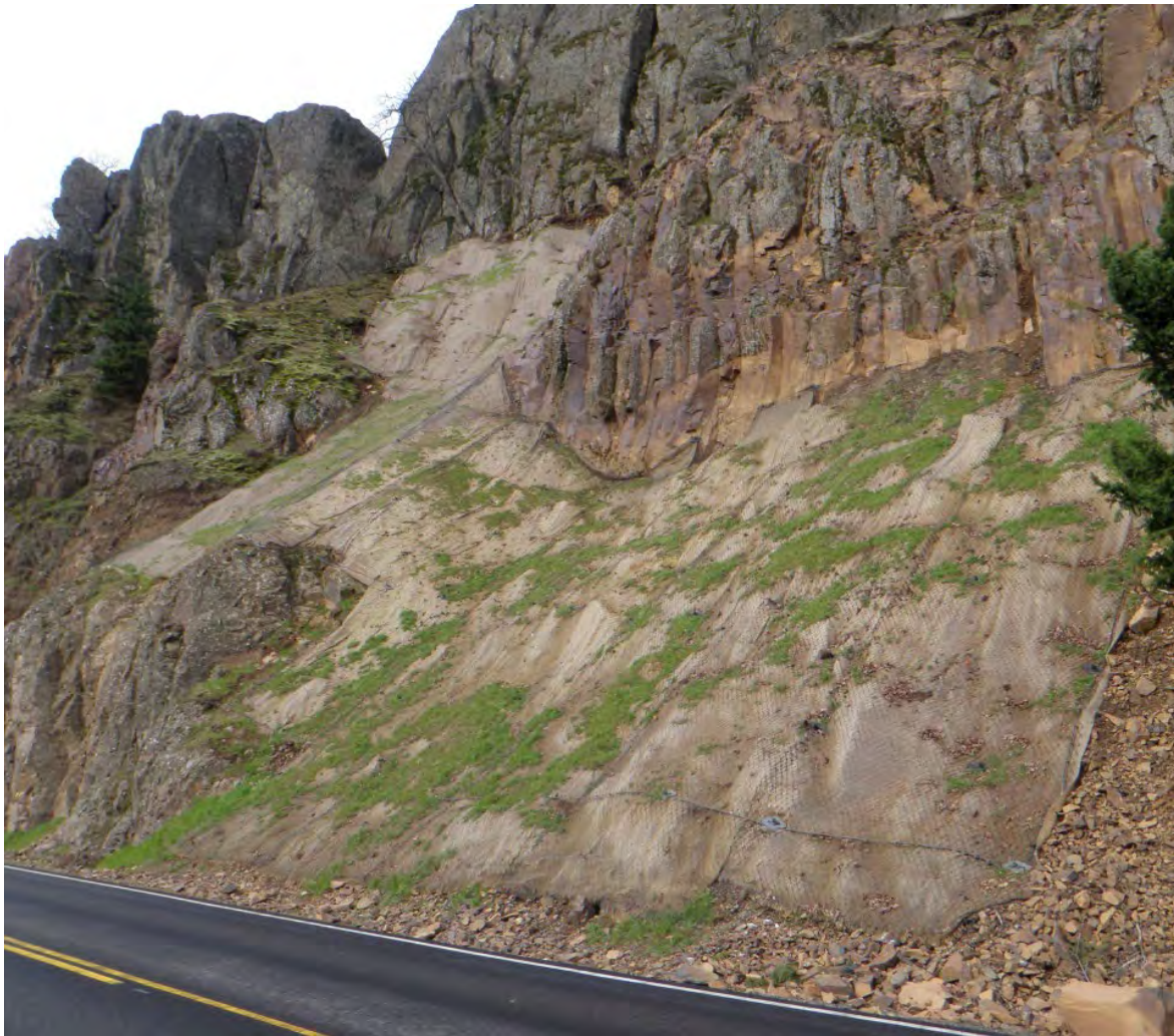
Figure 4-10 Example of Pinned Wire Mesh Slope (WSDOT).
