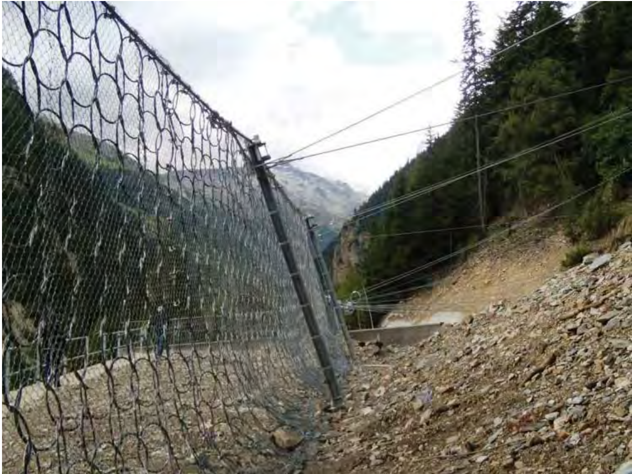
Figure 4-6 Example of a Ring-Net Flexible Barrier (from Andrew et al., 2011).
