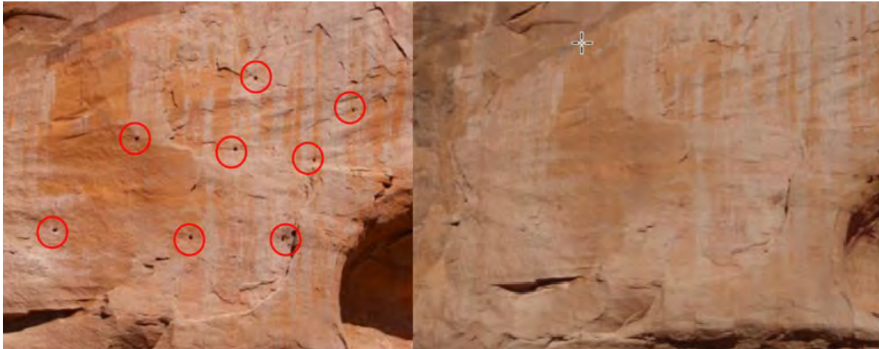
Figure 4-3 Before and After Camouflaged Rock Reinforcement (Colorado National Monument, from CFLHD).
