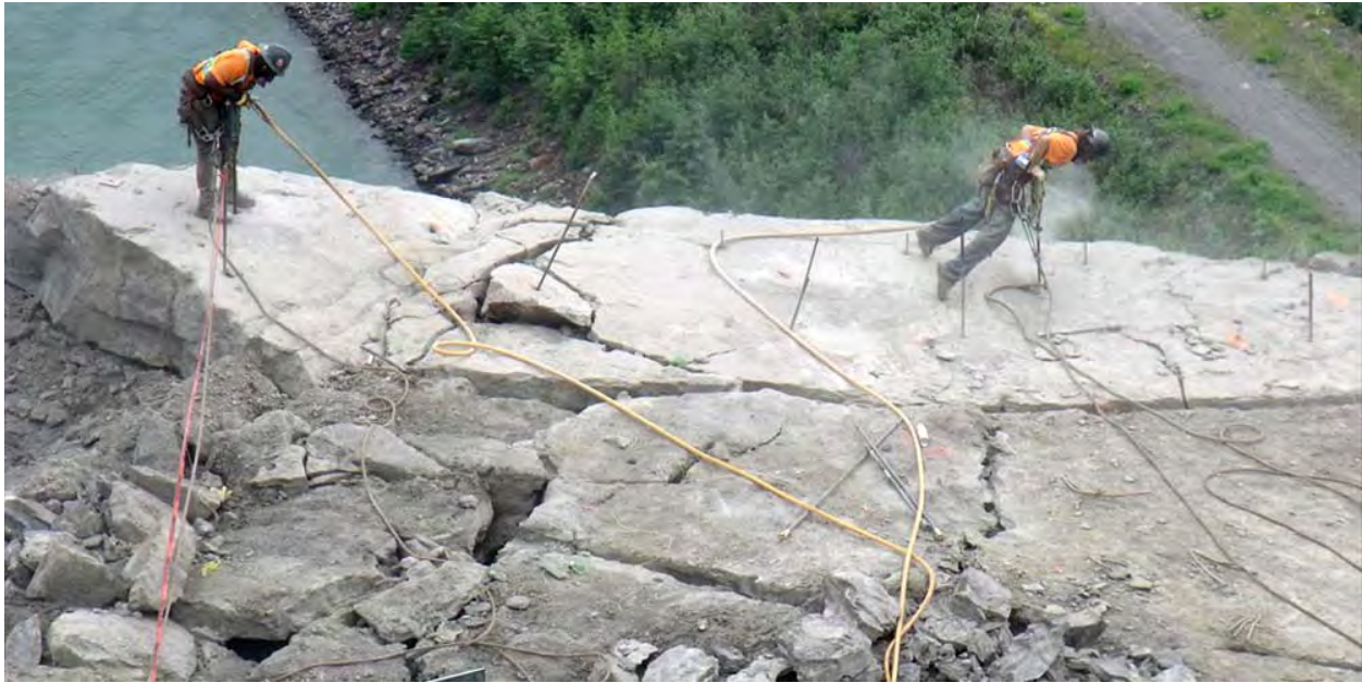
Figure 4-4 Hand Drilling for Trim Blasting on a Fractured Slope (from Matcon).
