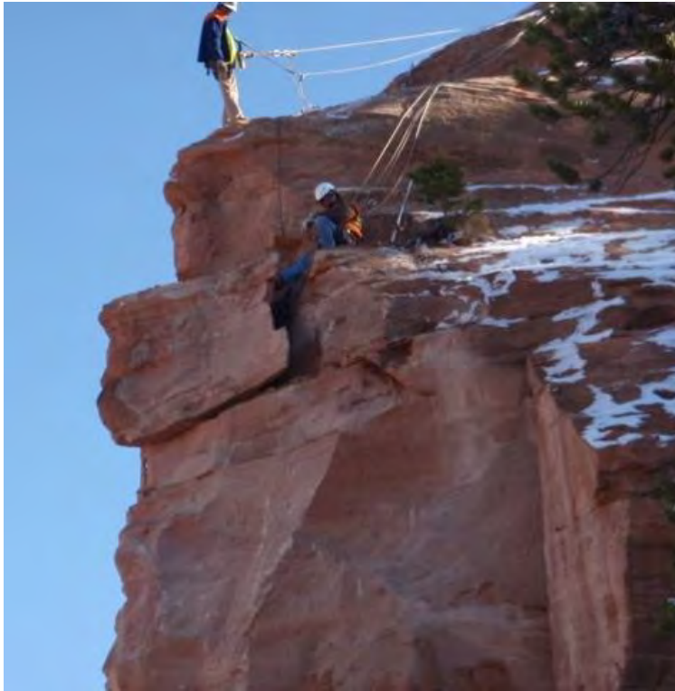
Figure 4-1 Typical Hand Scaling Setup (Colorado National Monument, from CFLHD).
