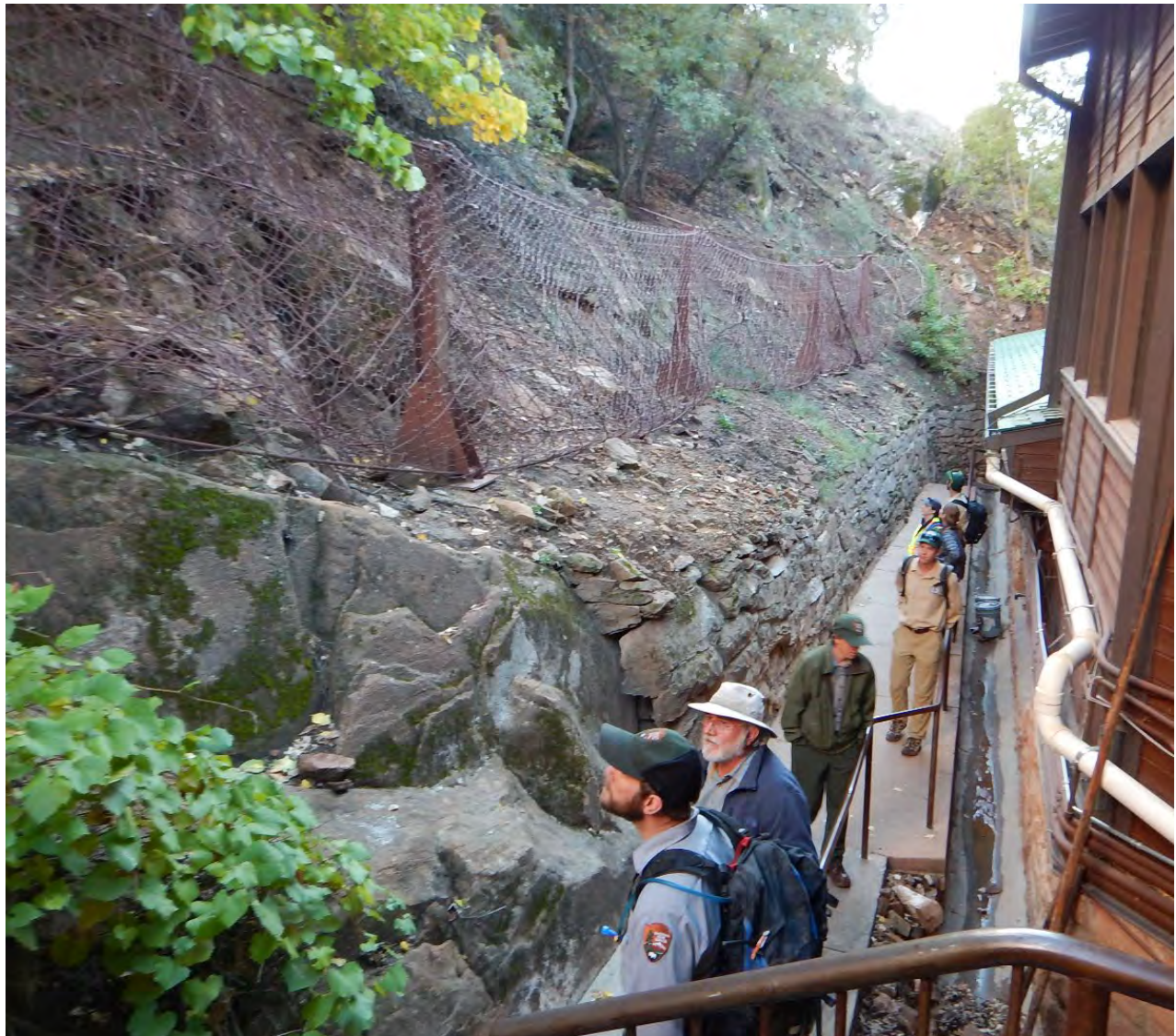
Figure 4-7 Rockfall Fence behind Zion Lodge.
