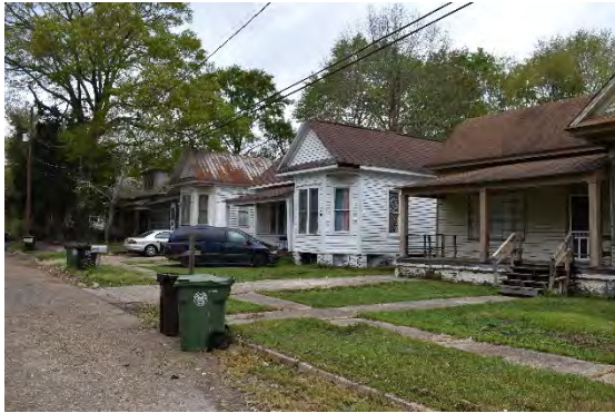
Photograph 7. Row of Bayed Cottages Along Short Katie Avenue, 2020
