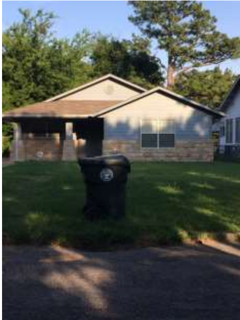
New construction on North 14 th St. modern Bungalow design
