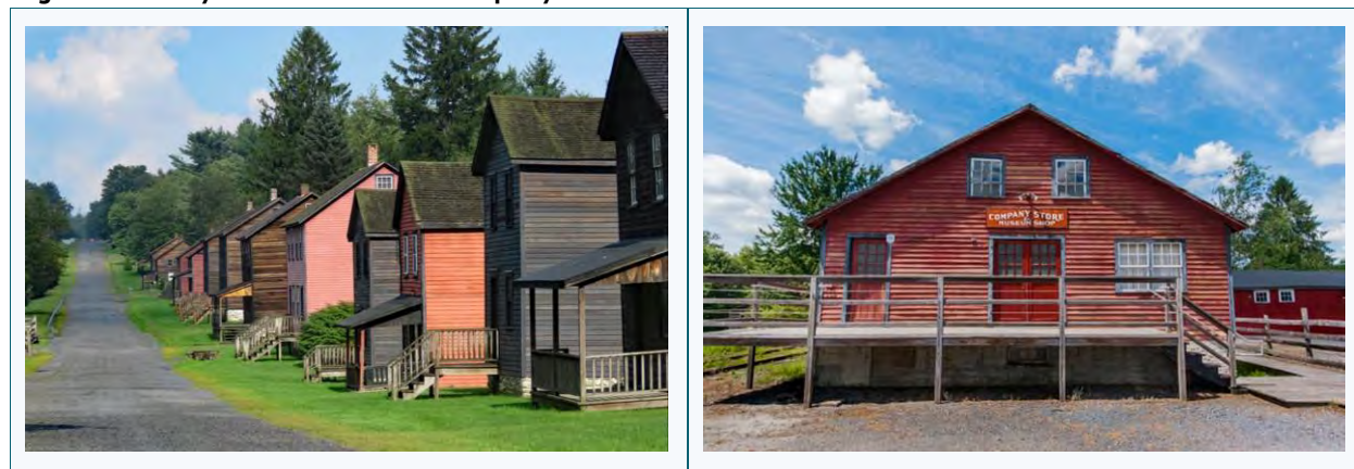
Figure 2: Eckley Houses and the Company Store
