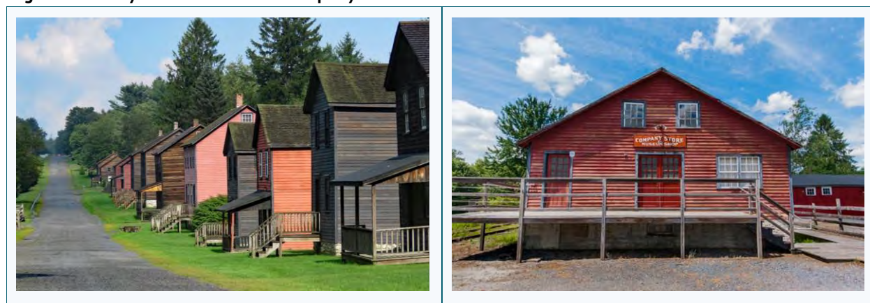
Figure 2: Eckley Houses and the Company Store
